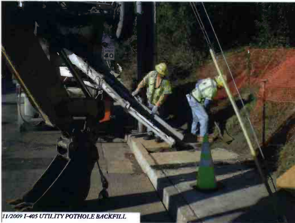
I-405 utility pothole backfill.
