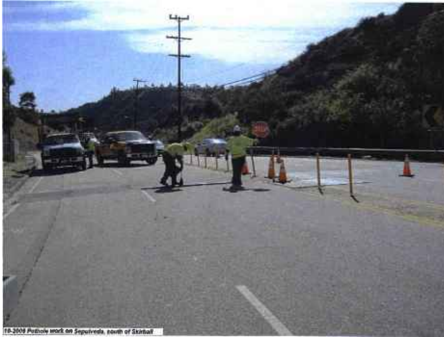
Pothole work on Sepulveda south of Skirball.
