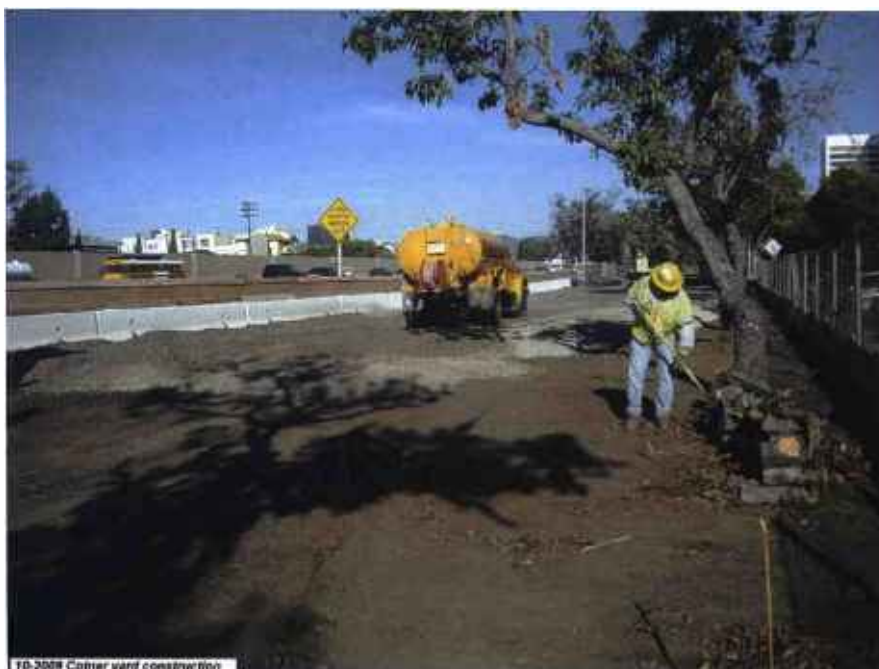
Cotner Yard construction.
