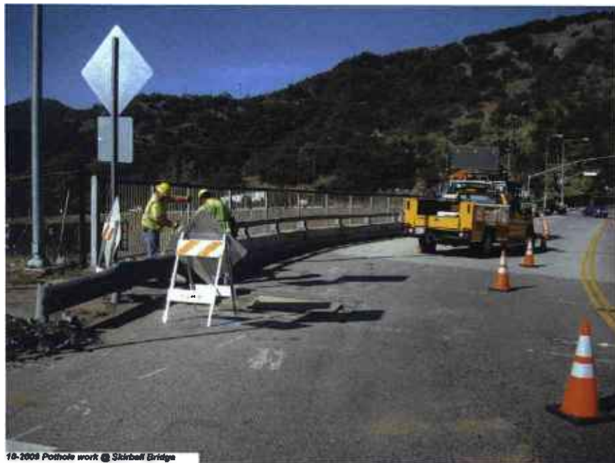
10-2009 Pothole work @ Skirball Bridge
