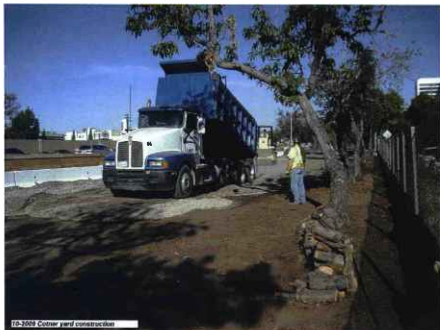
Cotner Yard construction.
