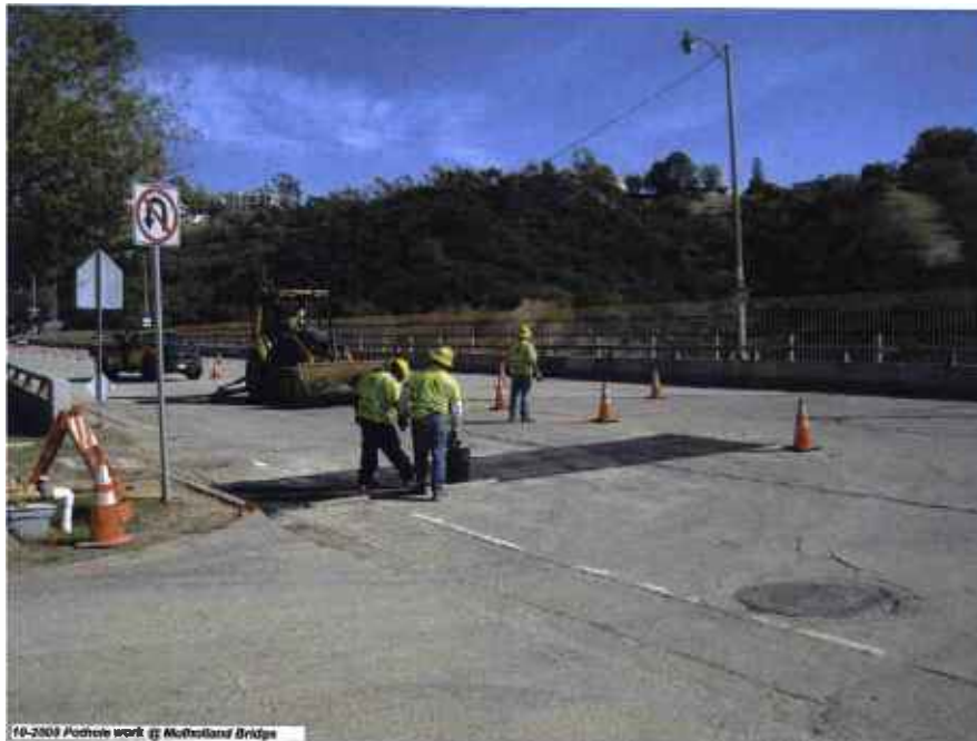
Pothole work at Mulholland Bridge.
