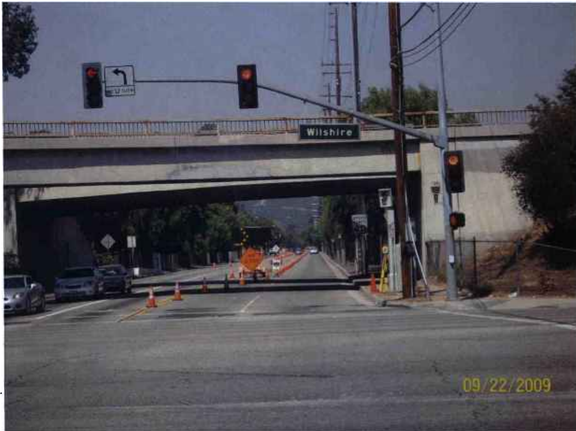
Maintenance of Traffic (MOT) Sepulveda Blvd. & Wilshire.
