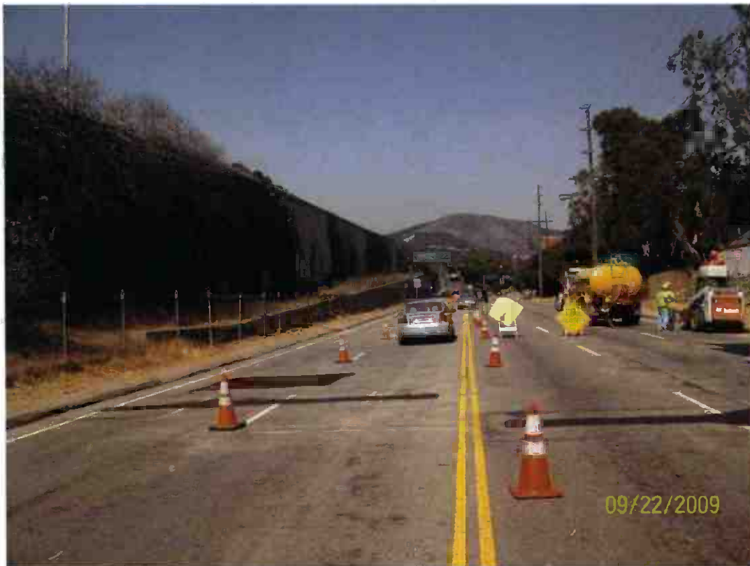
Maintenance of Traffic (MOT) Sepulveda Blvd.
