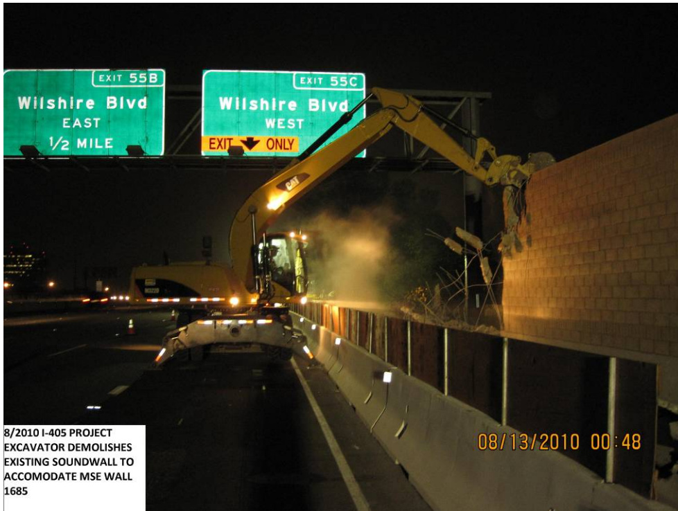
Excavator demolishes existing soundwall to accommodate MSE Wall 1685.
