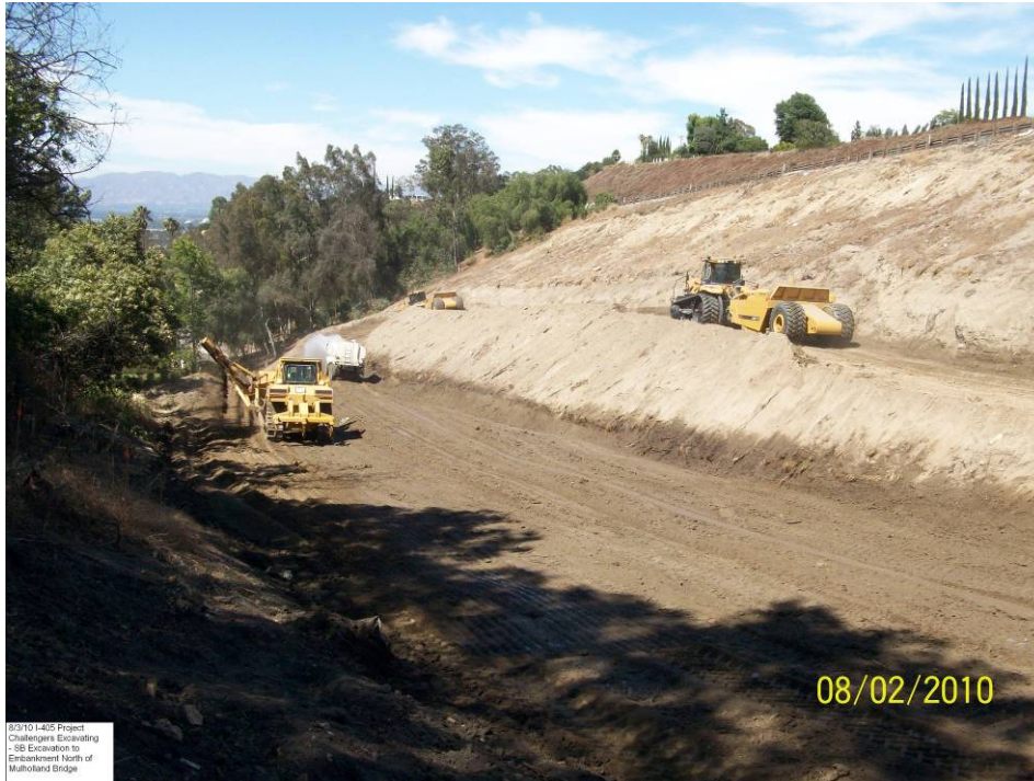
Challengers excavating – SB excavation to embankment north of Mulholland Bridge.
