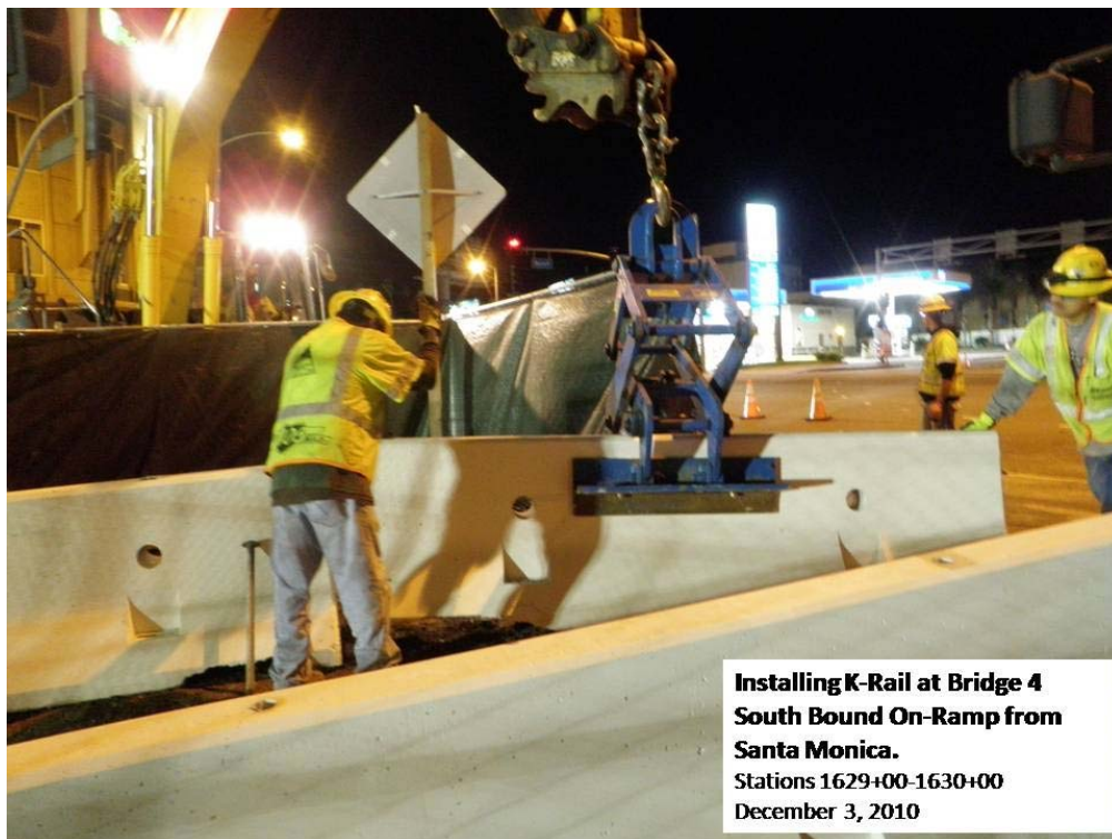
Installing k-rail at Bridge 4 south bound on-ramp from Santa Monica.
