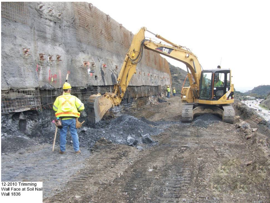
Trimming wall face at soil nail Wall 1836.
