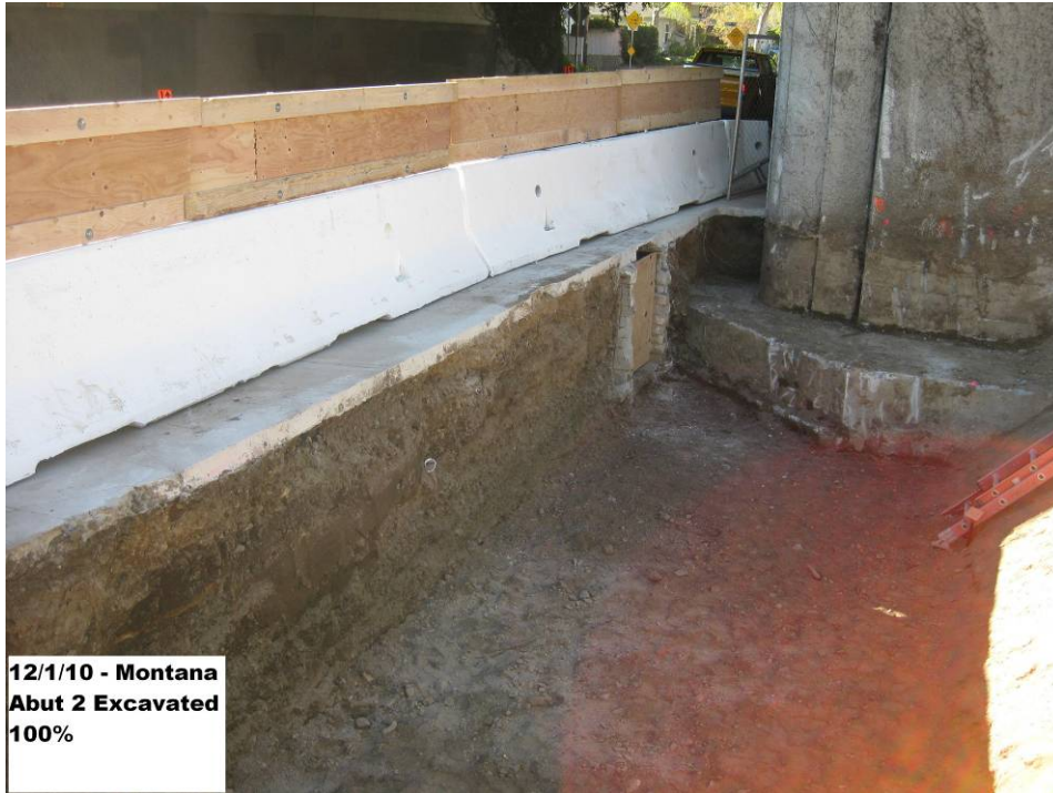
Montana abutment #2 excavated 100%.
