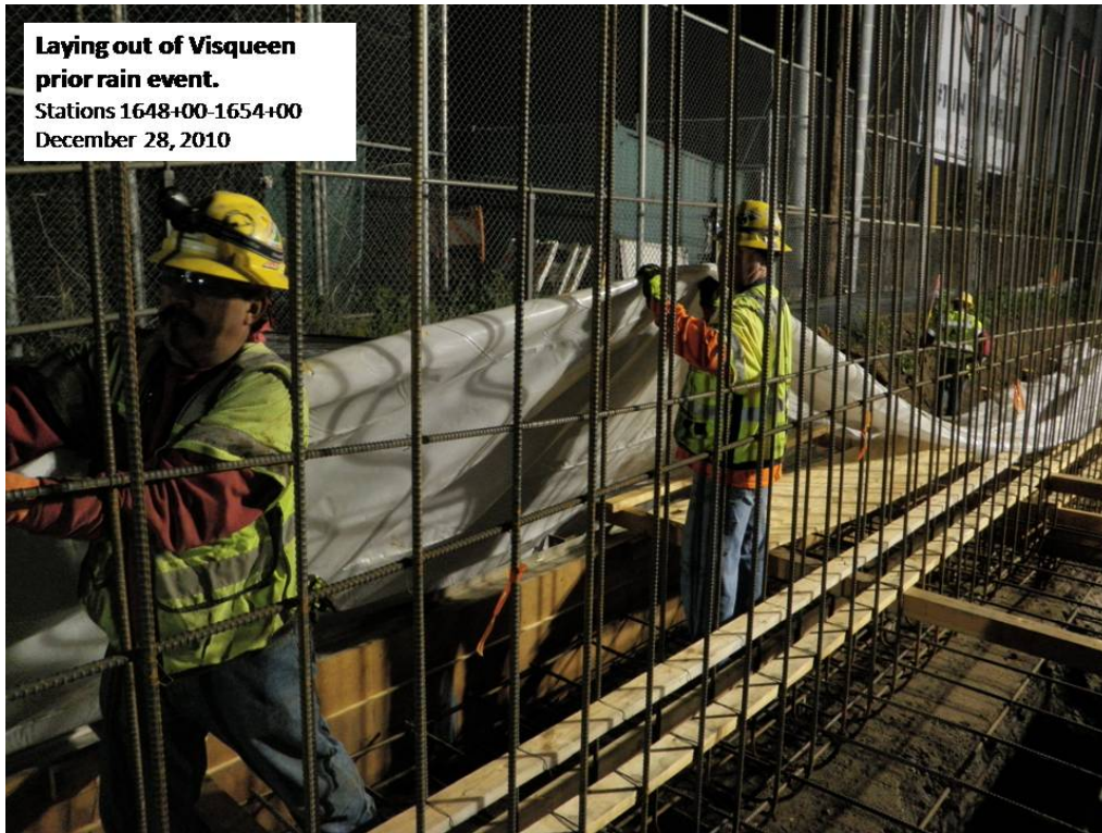
Laying out visqueen prior to rain event.
