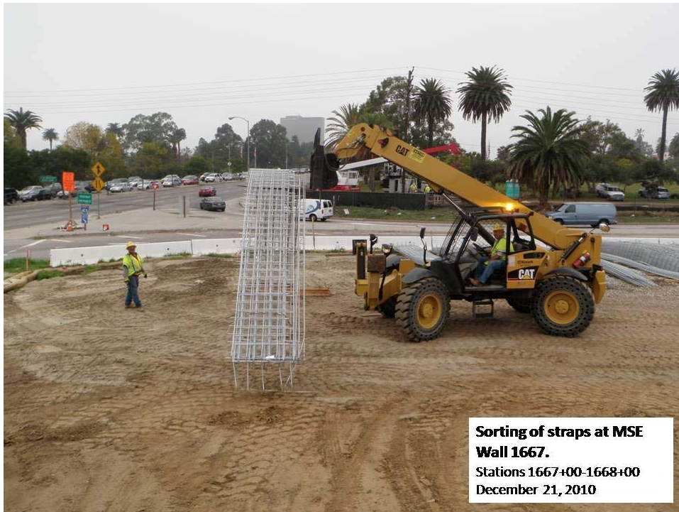
Sorting of straps at MSE Wall 1667.
