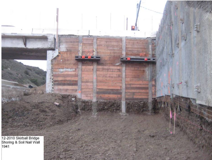
Skirball Bridge shoring and soil nail Wall 1941.
