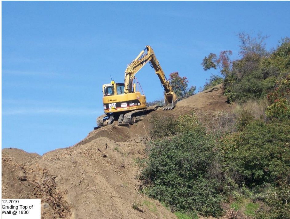
Grading top of Wall 1836.
