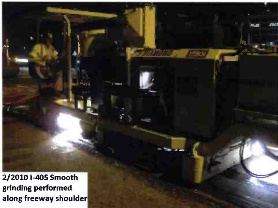
Smooth grinding performed along freeway shoulder.
