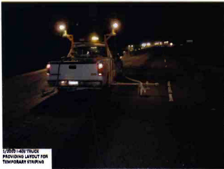
Truck providing layout for temporary striping.
