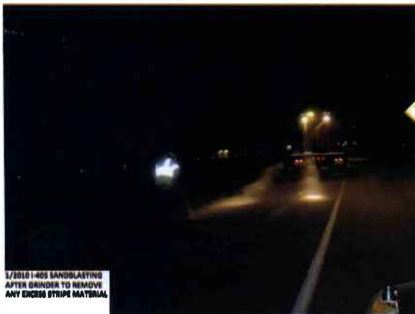
Sandblasting after grinder to remove any excess stripe material.
