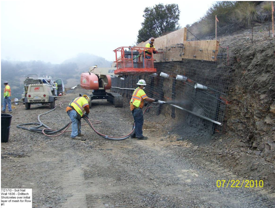
Soil Nail Wall 1836 – Shotcretes over initial layer of mesh for row 1.
