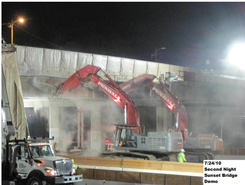
Second night Sunset Bridge demo.
