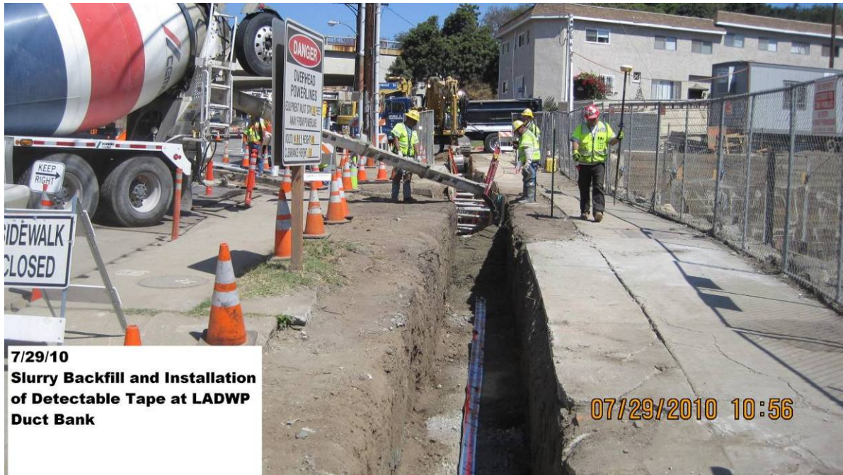
Slurry backfill and installation of detectable tape at LADWP ductbank.
