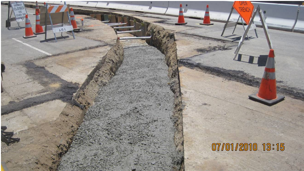
Sepulveda ductbank concrete encasement.
