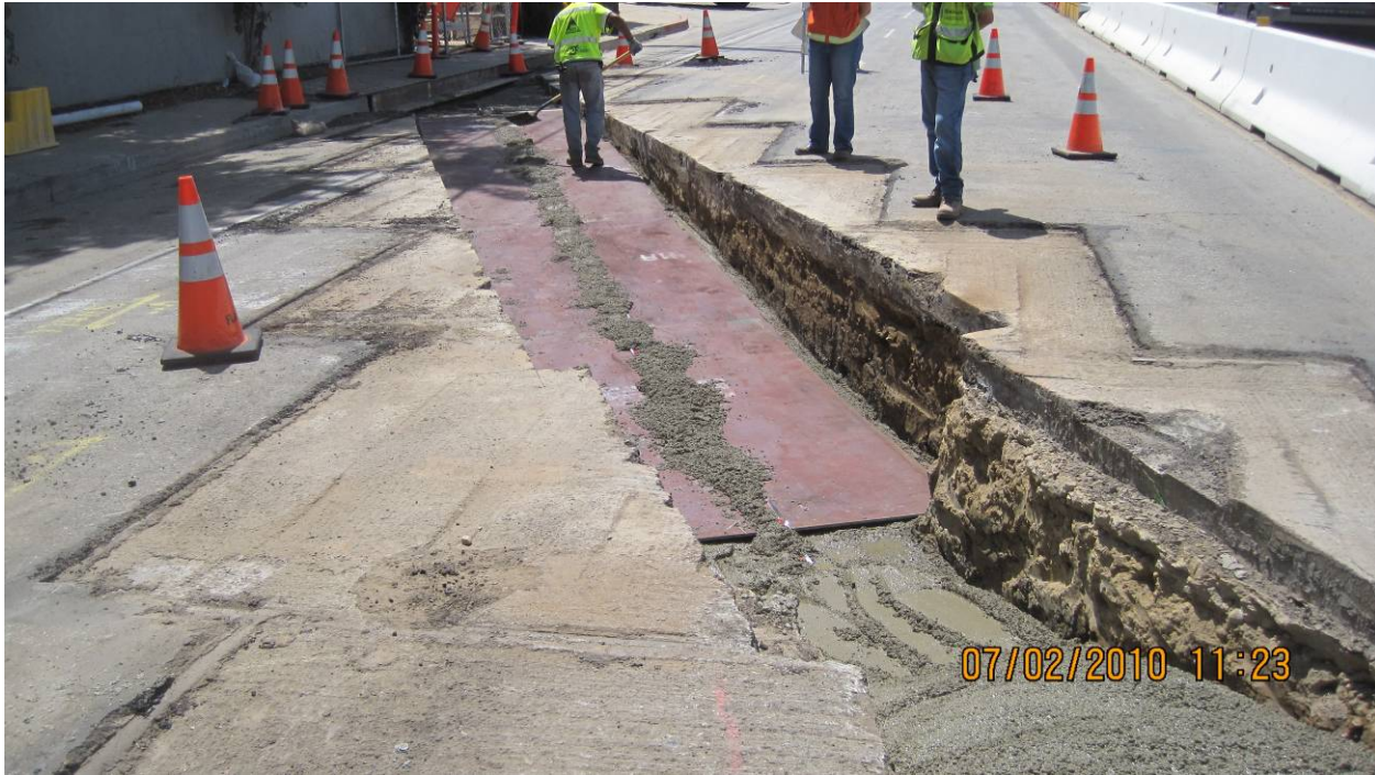
Ductbank slurry backfill with ½" plates.
