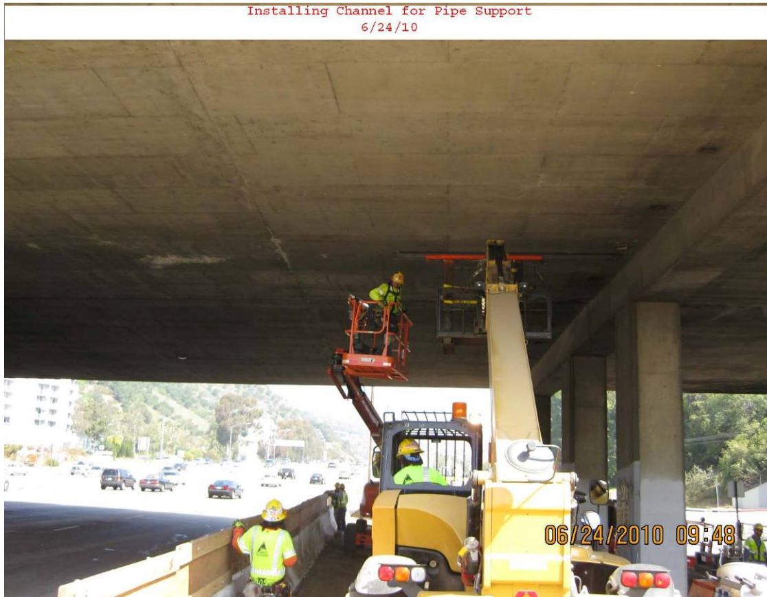
Install channel under Sunset Bridge for pipe support.
