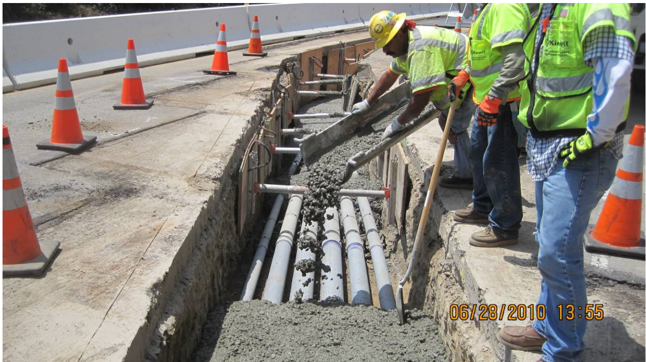
Sepulveda ductbank concrete encasement.
