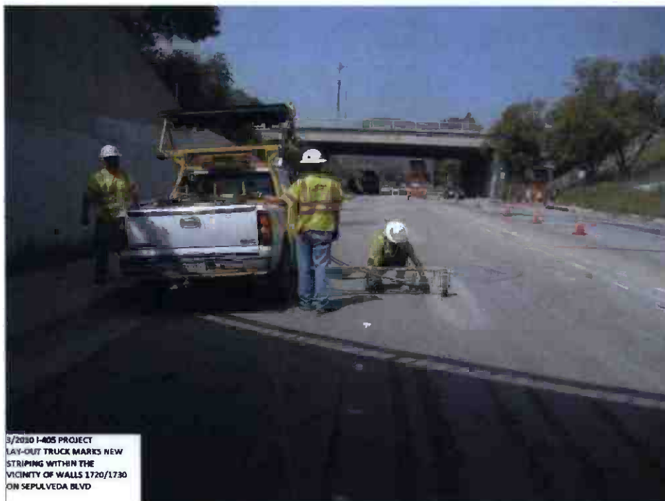
Lay-out truck marks new striping within the vicinity of walls 1720/1730 on Sepulveda Blvd.
