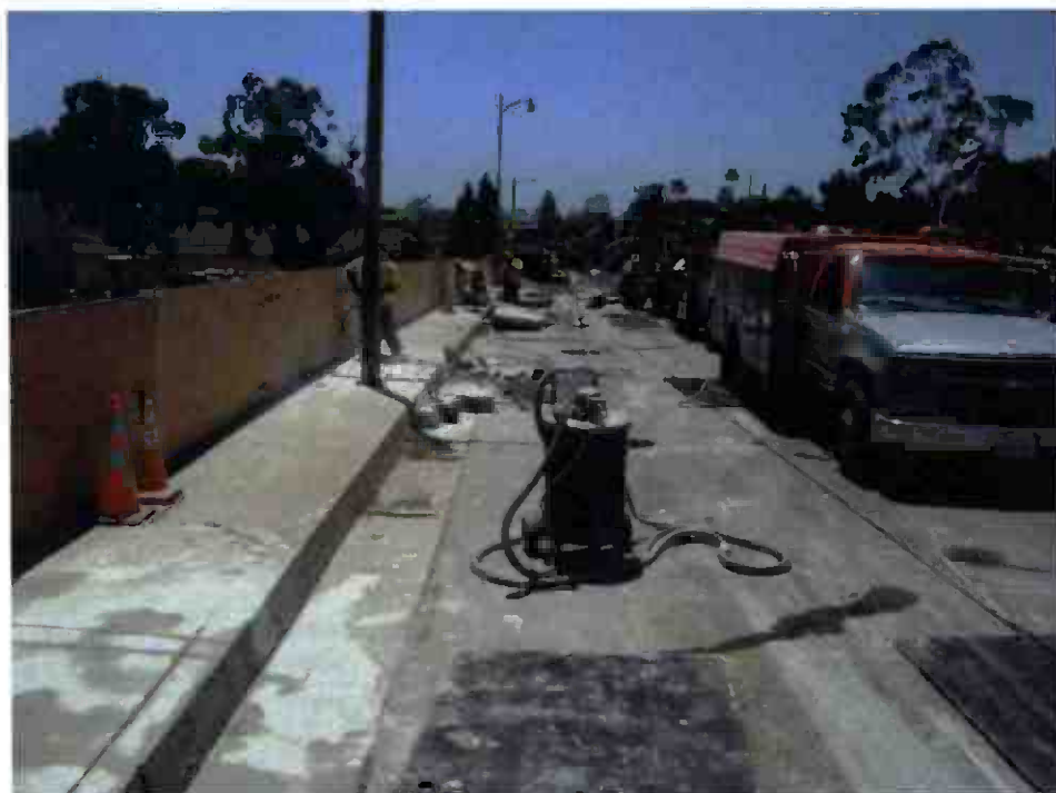
Penhall cutting access holes on Sunset Bridge for demo.
