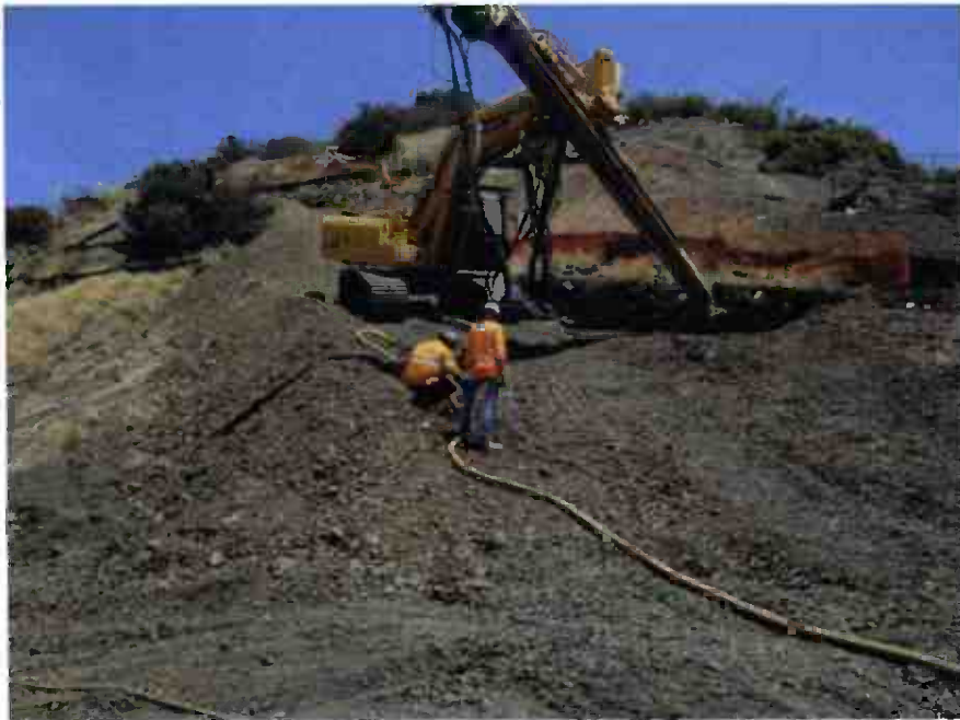
Soil Nail Test at Wall 1836.
