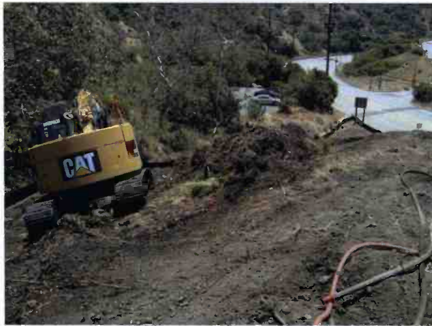
Clear and grub at Wall 1836.
