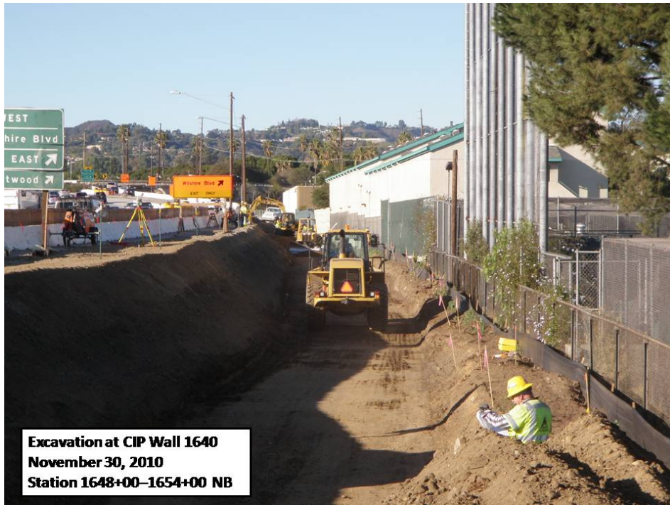
Excavation at CIP Wall 1640.
