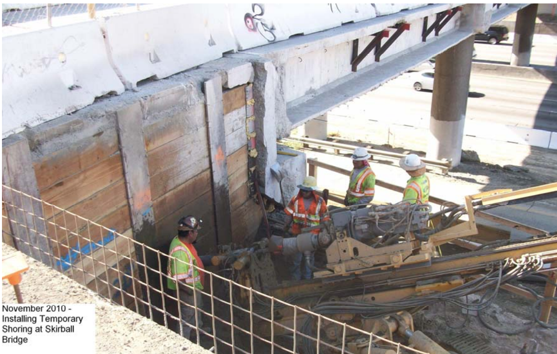
Installing temporary shoring at Skirball Bridge.
