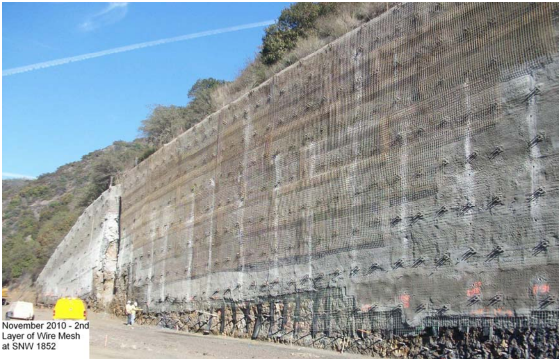
Second layer of wire mesh at SNW 1852.
