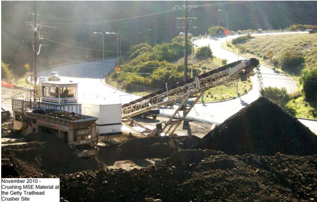
Crushing MSE material at the Getty Trailhead crusher site.
