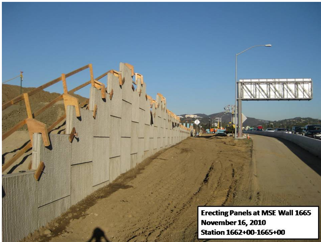
Erecting panels at MSE Wall 1665.
