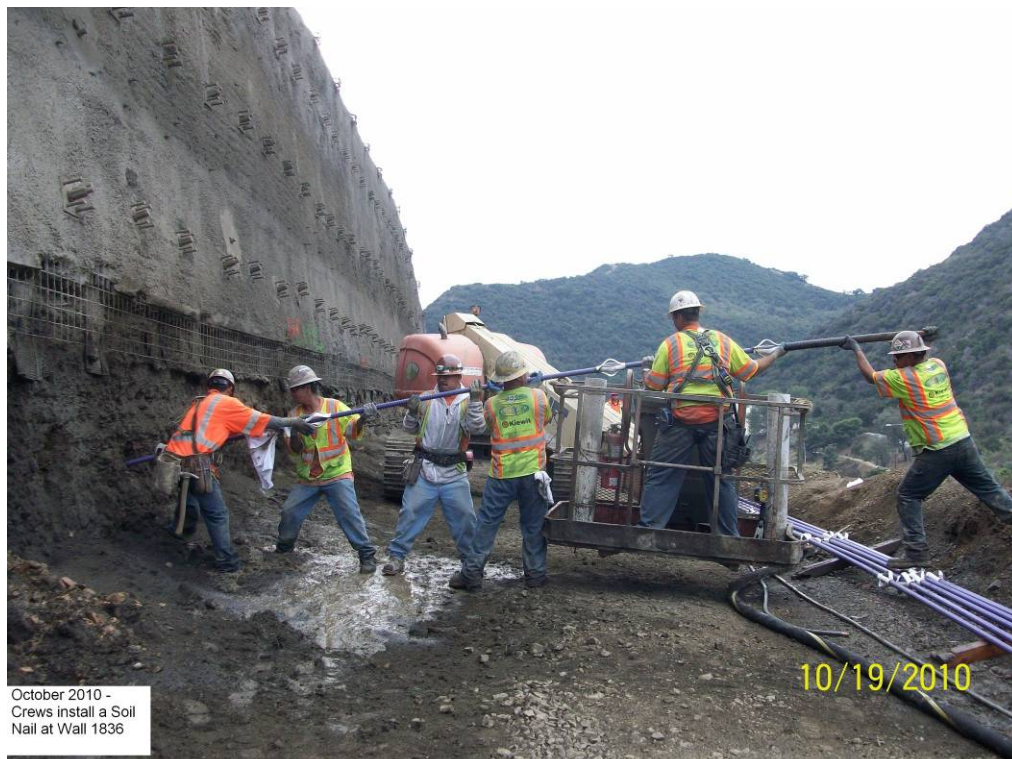
Crews install a soil nail at Wall 1836.
