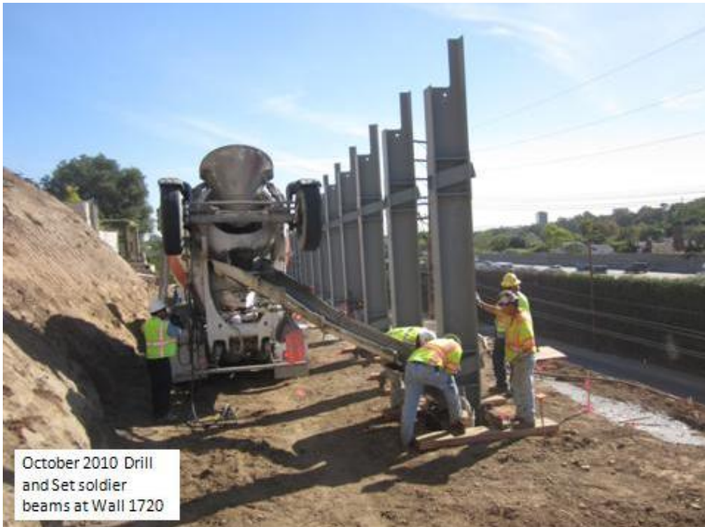
Drill and set soldier beams at Wall 1720.
