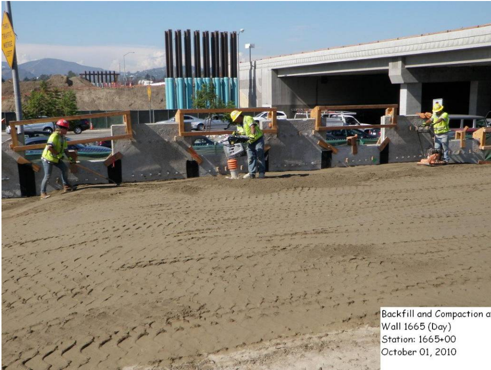
Backfill and compaction at Wall 1665.
