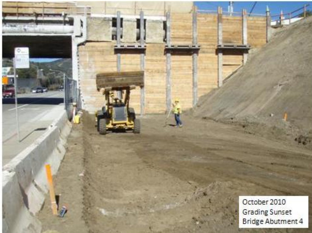
Grading Sunset Bridge Abutment 4.
