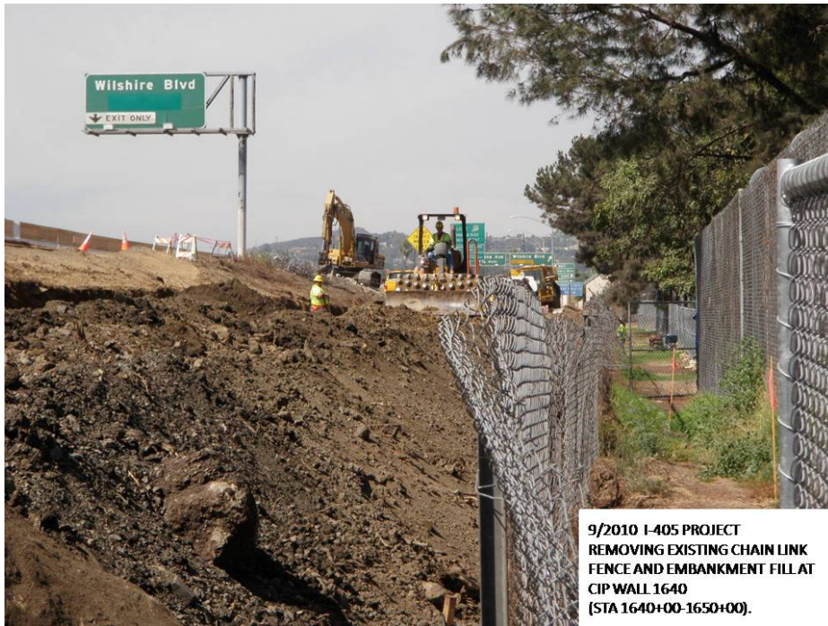
Removing existing chain link fence and embankment fill at CIP Wall 1640.
