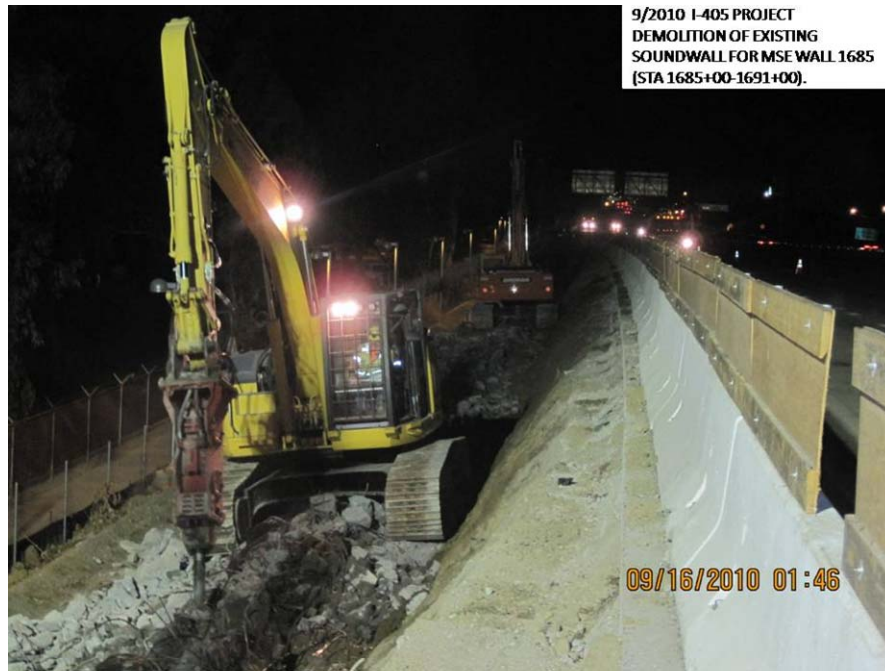
Demolition of existing soundwall for MSE Wall 1685.
