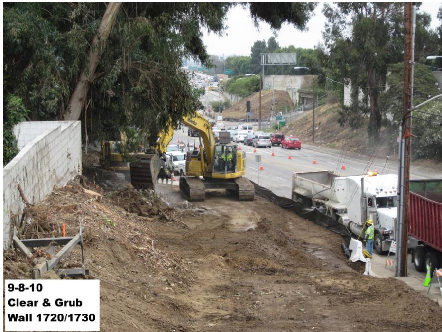
Clear and grub Wall 1720/1730.
