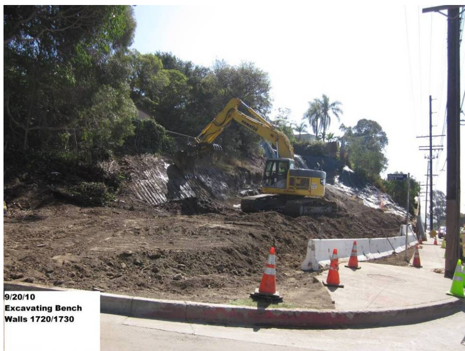
Excavating bench Walls 1720/1730.
