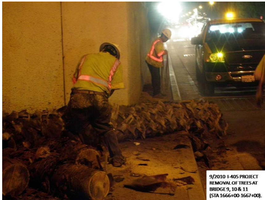
Project removal of trees at bridges 9, 10 and 11.
