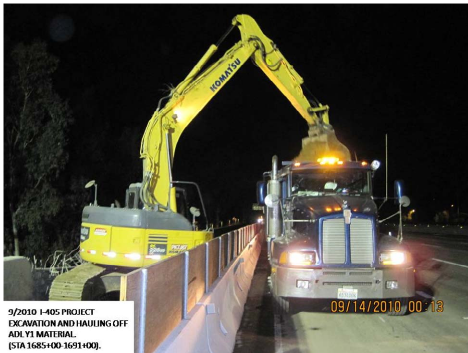
Excavation and hauling off ADLY1 material.
