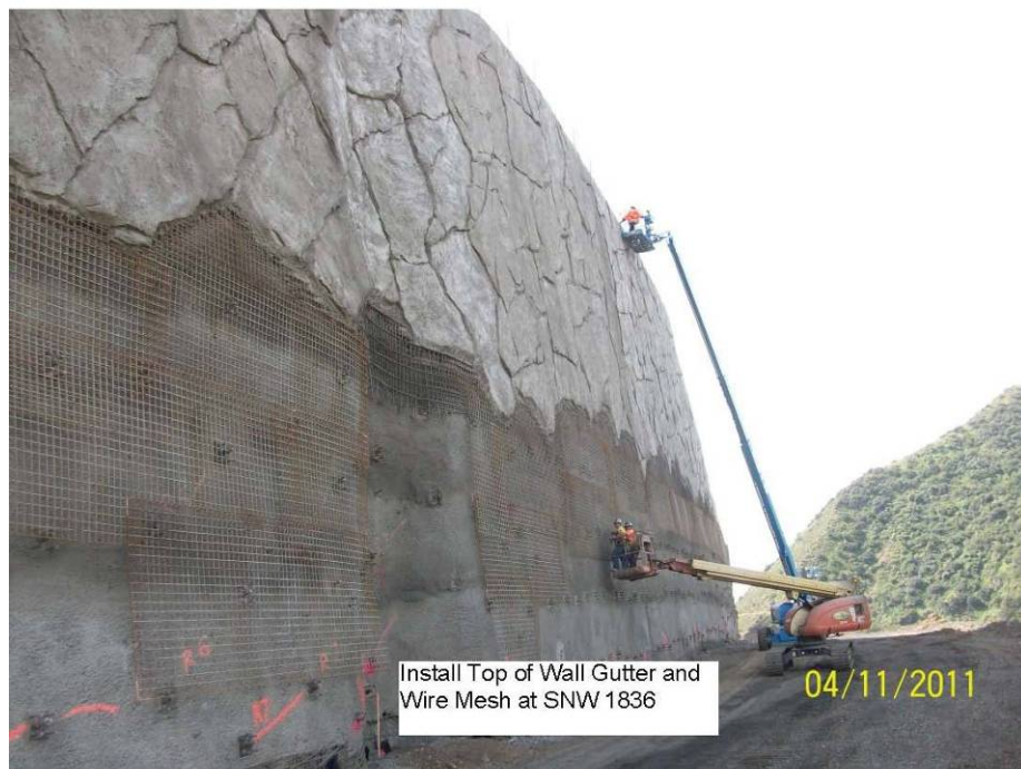
Install top of wall gutter and wire mesh at SNW 1836.
