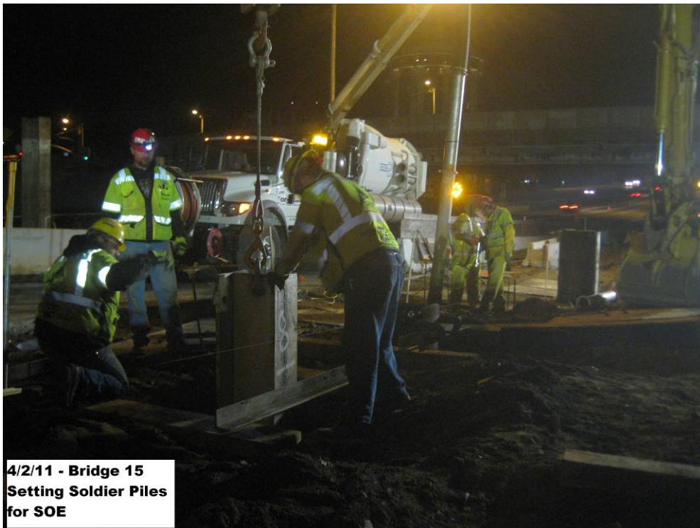
Bridge 15 setting soldier piles for SOE.
