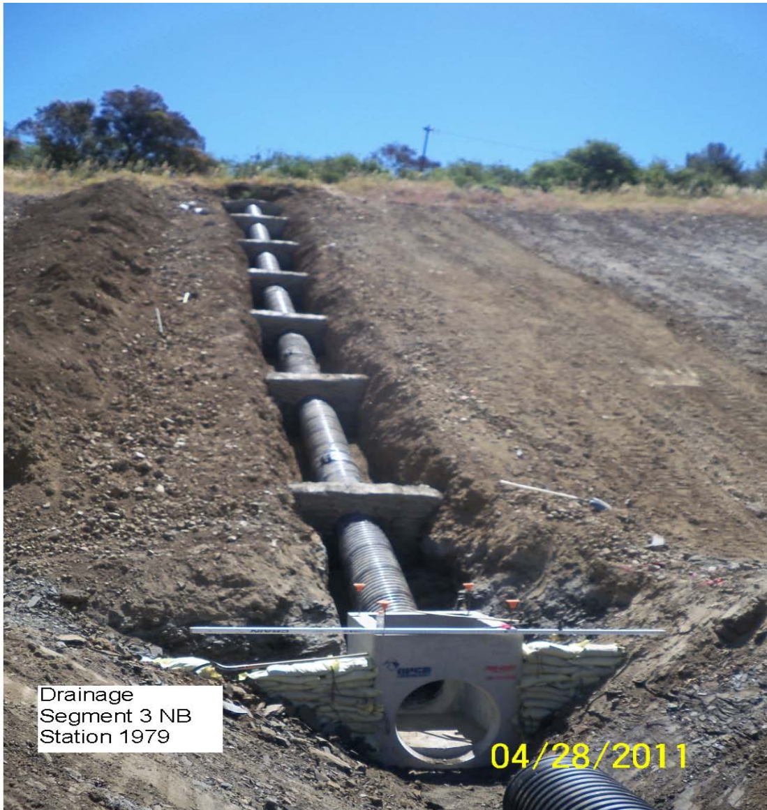
Drainage Segment 3 NB Station 1979.
