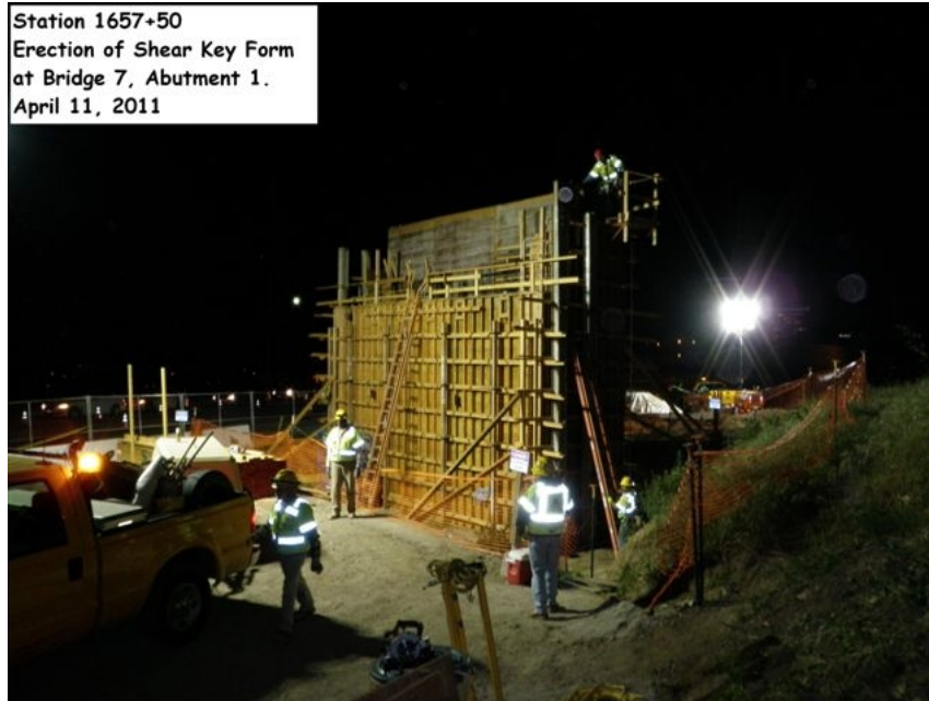
Station 1657+50. Erection of shear key form at Bridge 7, Abutment 1.
