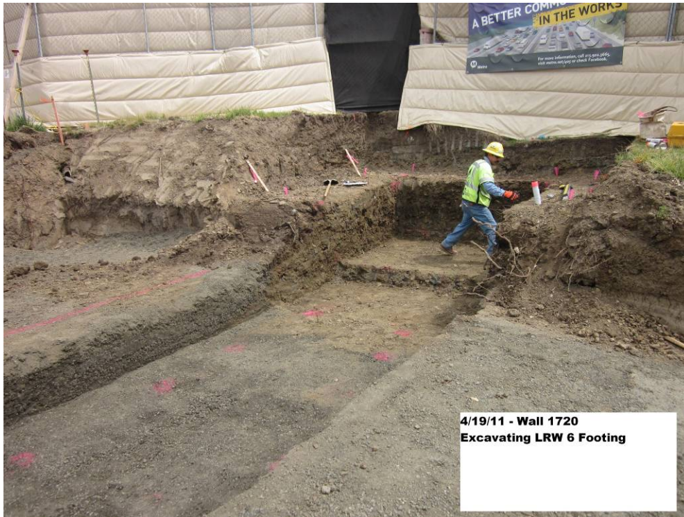
Wall 1720. Excavating LRW 6 footing.
