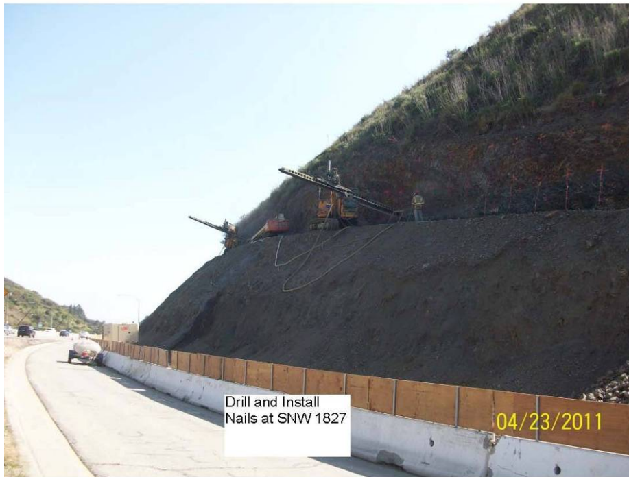
Drill and install nails at SNW 1827.
