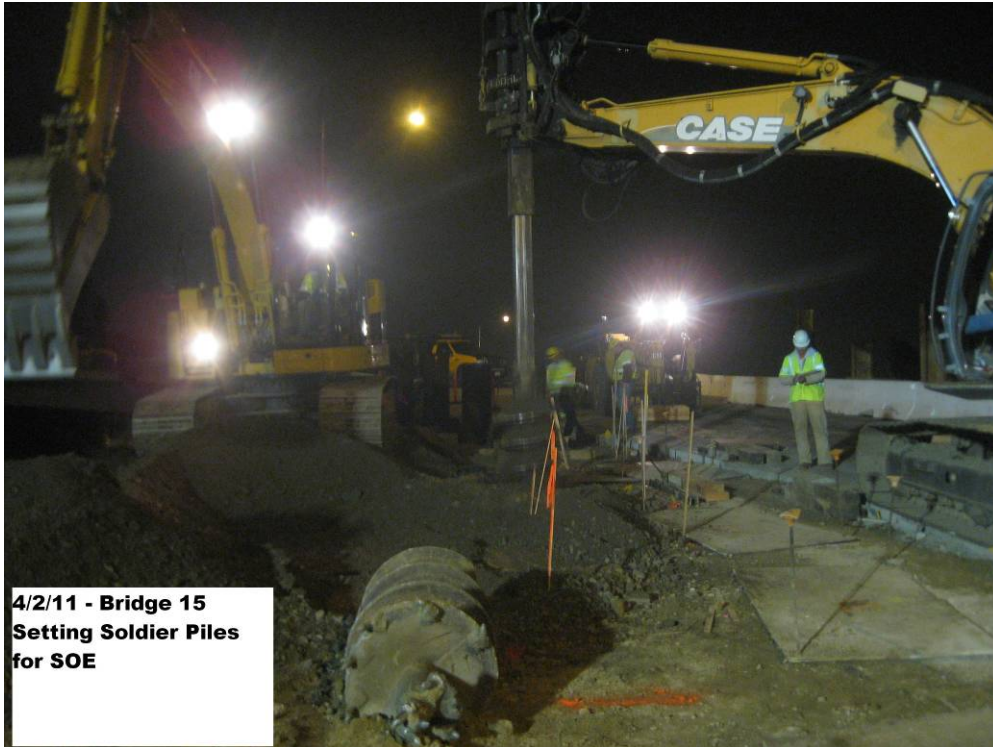
Bridge 15 setting soldier piles for SOE.
