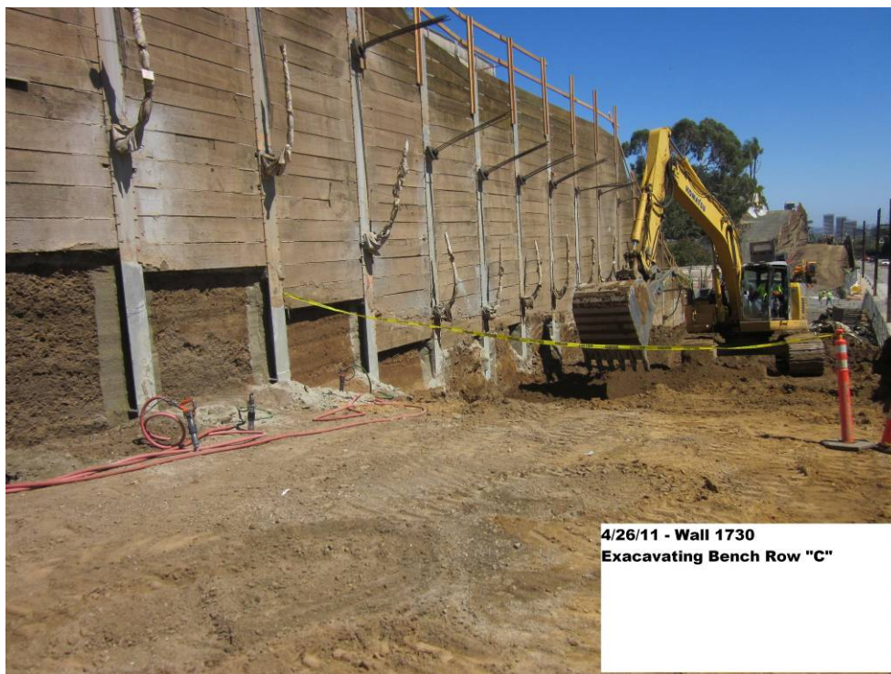
Wall 1730. Excavating bench row "C".
