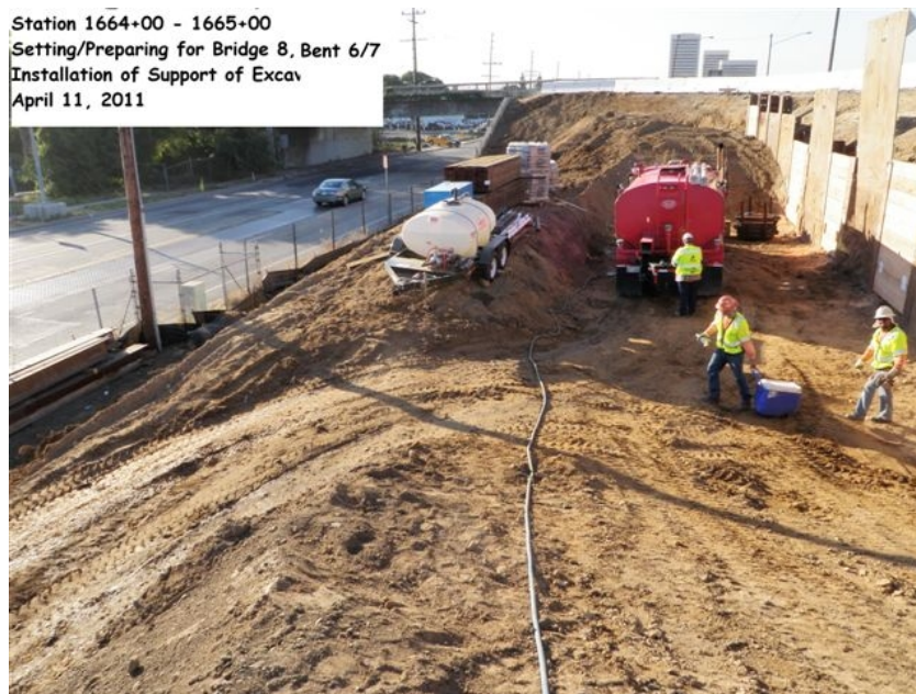
Station 1664+00 – 1665+00. Setting/preparing for Bridge 8, Bent 6/7. Installation of Support of Excavation.
