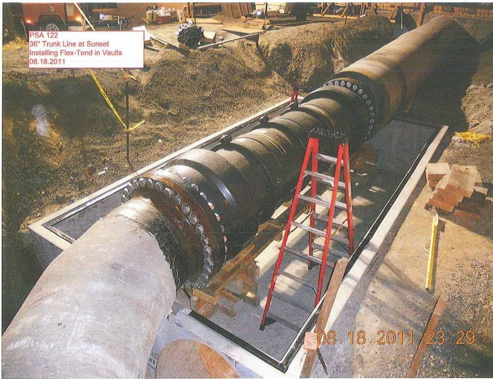
36" trunk line at Sunset installing flex-tend in vaults.
