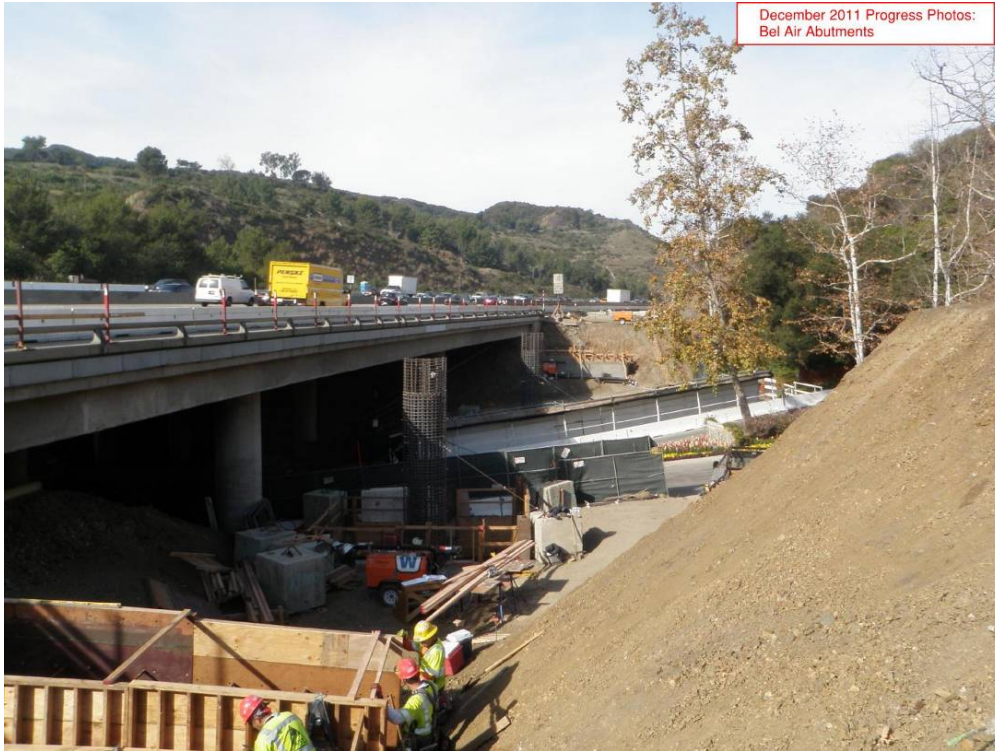
Bel Air Abutments.
