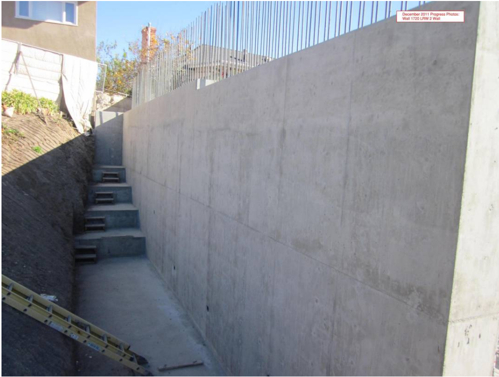
Wall 1720 LRW 2 Wall.
