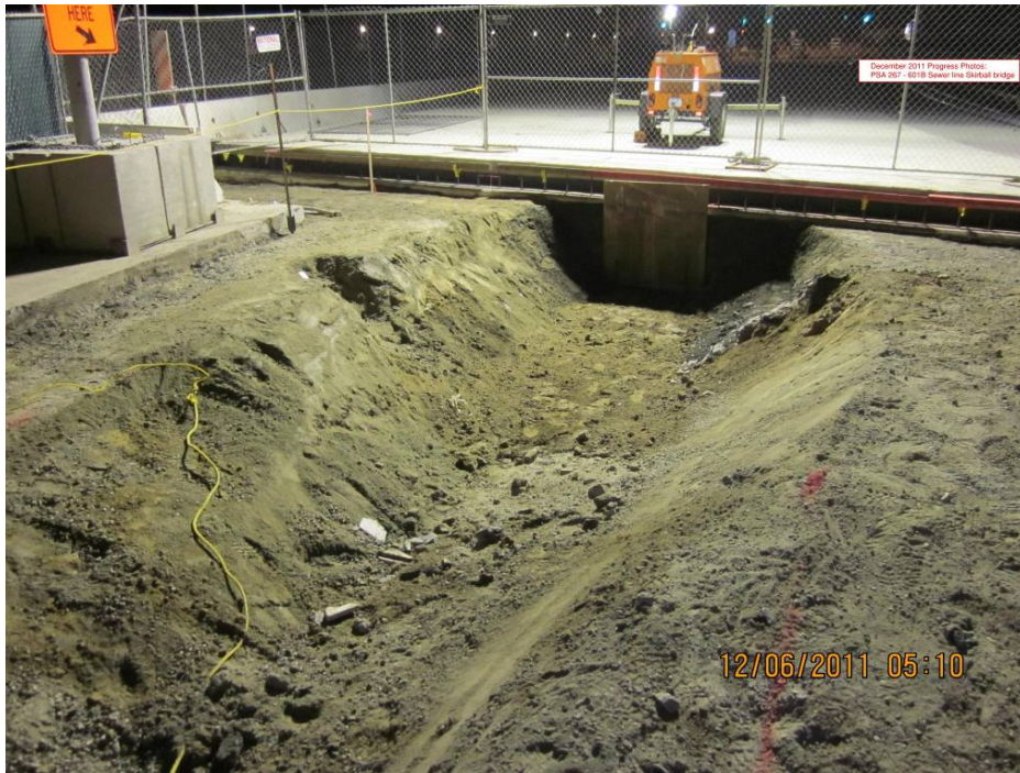
PSA 267 601B sewer line at Skirball Bridge.
