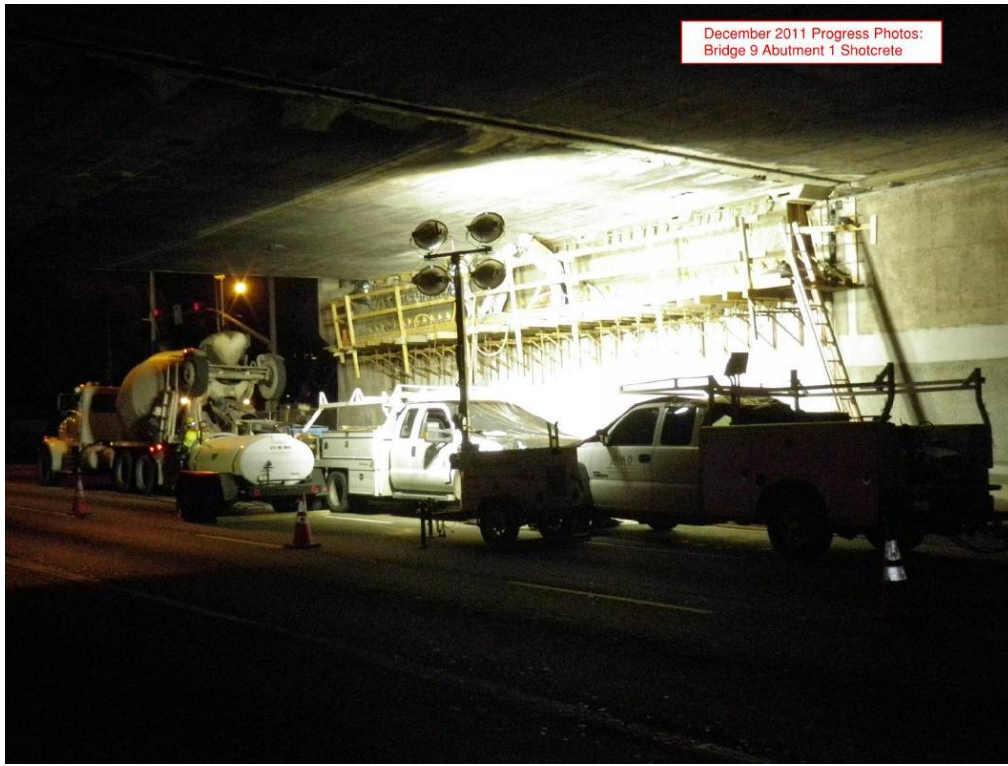
Bridge 9 Abutment 1 shotcrete.
