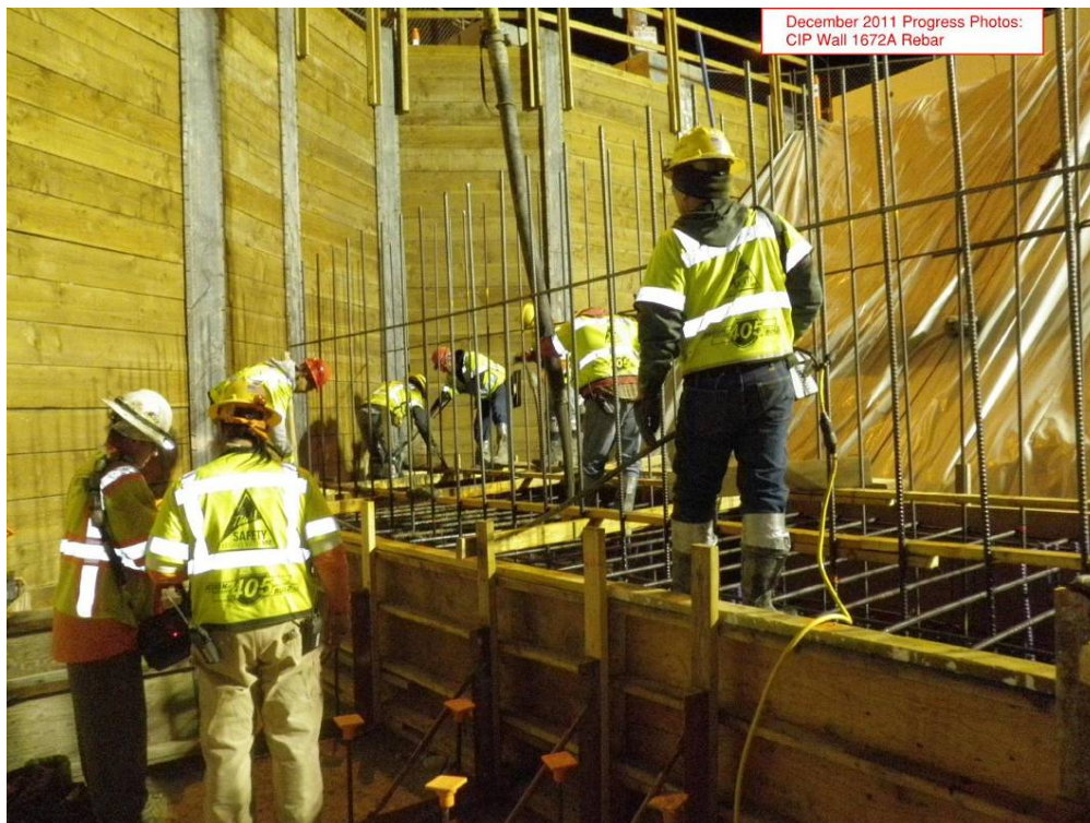
CIP Wall 1672A rebar.
