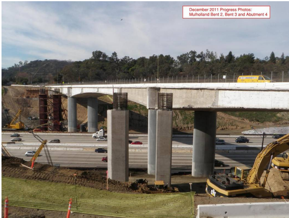
Mulholland Bent 2, Bent 3 and Abutment 4.
