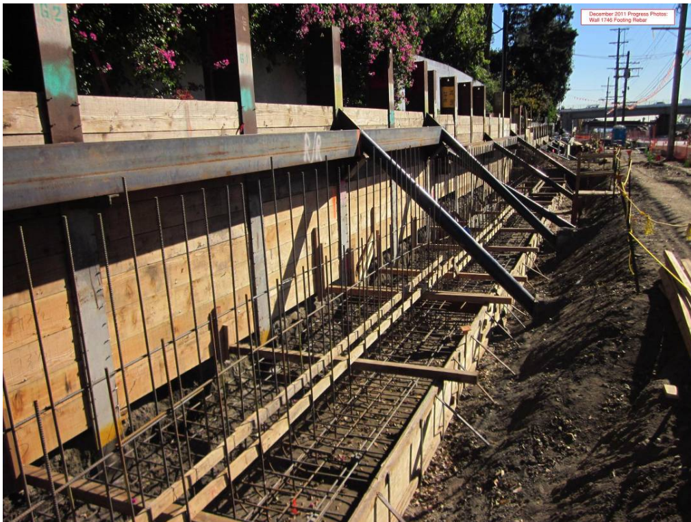
Wall 1746 footing rebar.
