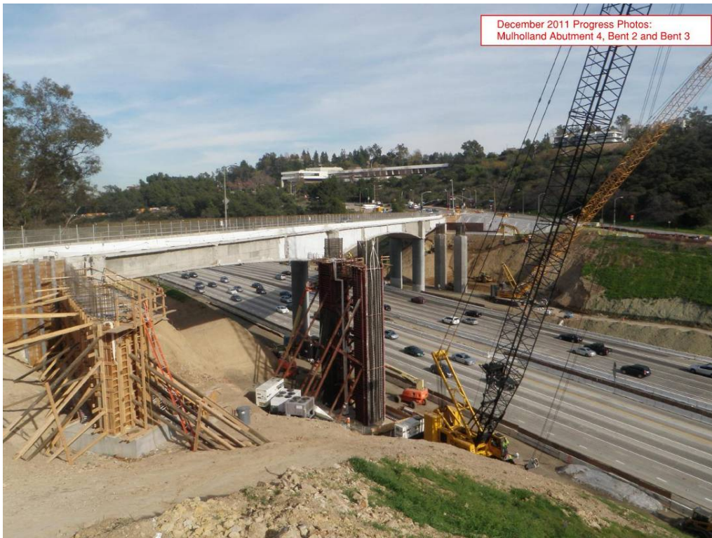
Mulholland Abutment 4, Bent 2 and Bent 3.
