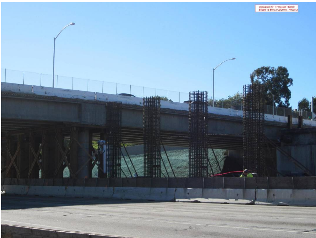
Bridge 16 Bent 2 Columns Phase 2.
