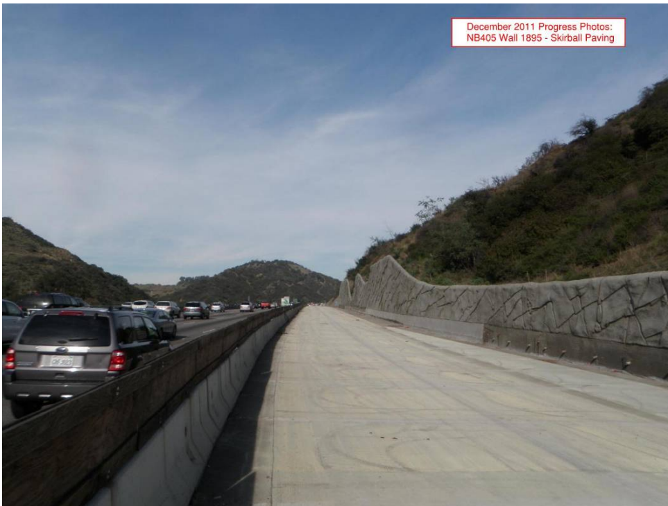
NB 405 Wall 1895 Skirball paving.
