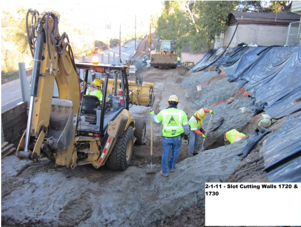
Slot cutting Walls 1720 and 1730.
