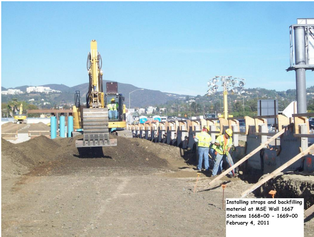
Installing straps and backfilling material at MSE Wall 1667 Stations 1668+00 – 1669+00.
