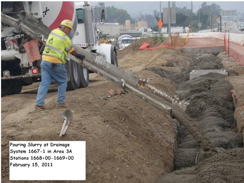
Pouring slurry at drainage system 1667-1 in Area 3A Stations 1668+00 – 1669+00.
