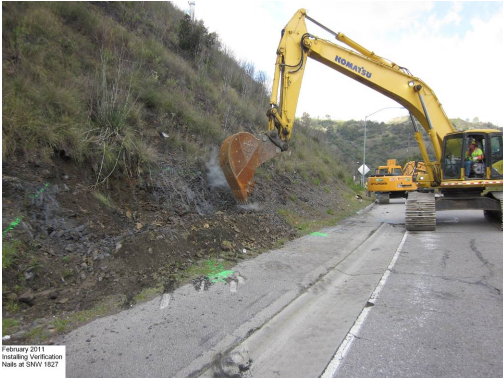
Installing verification nails at SNW 1827.
