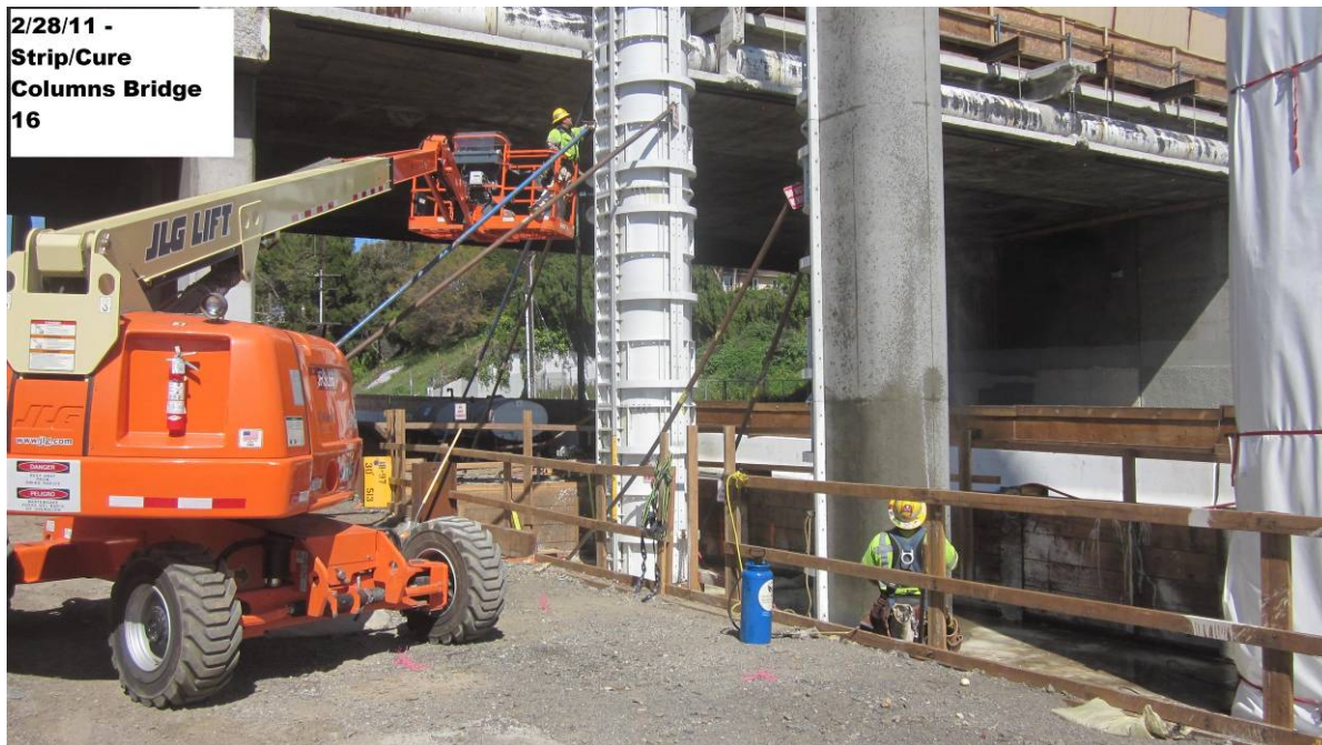
Strip/cure columns Bridge 16.
