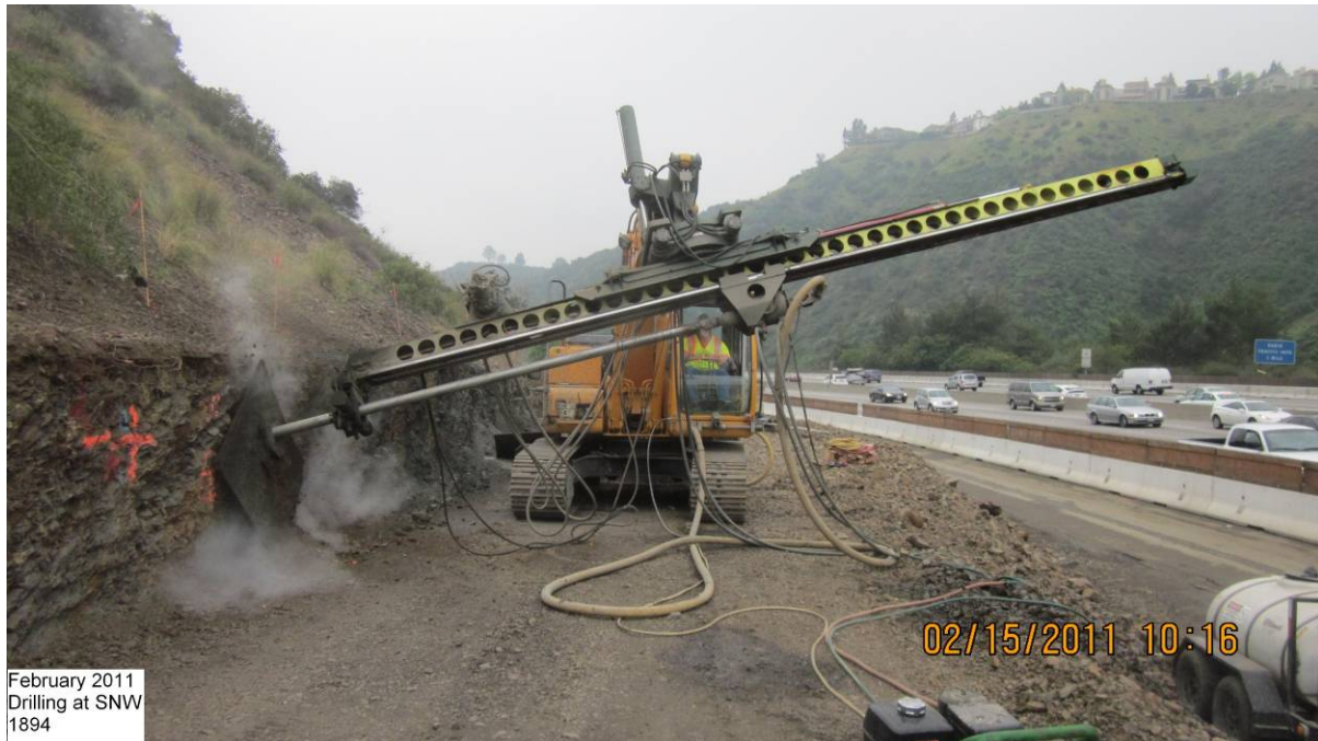
Drilling at SNW 1894.
