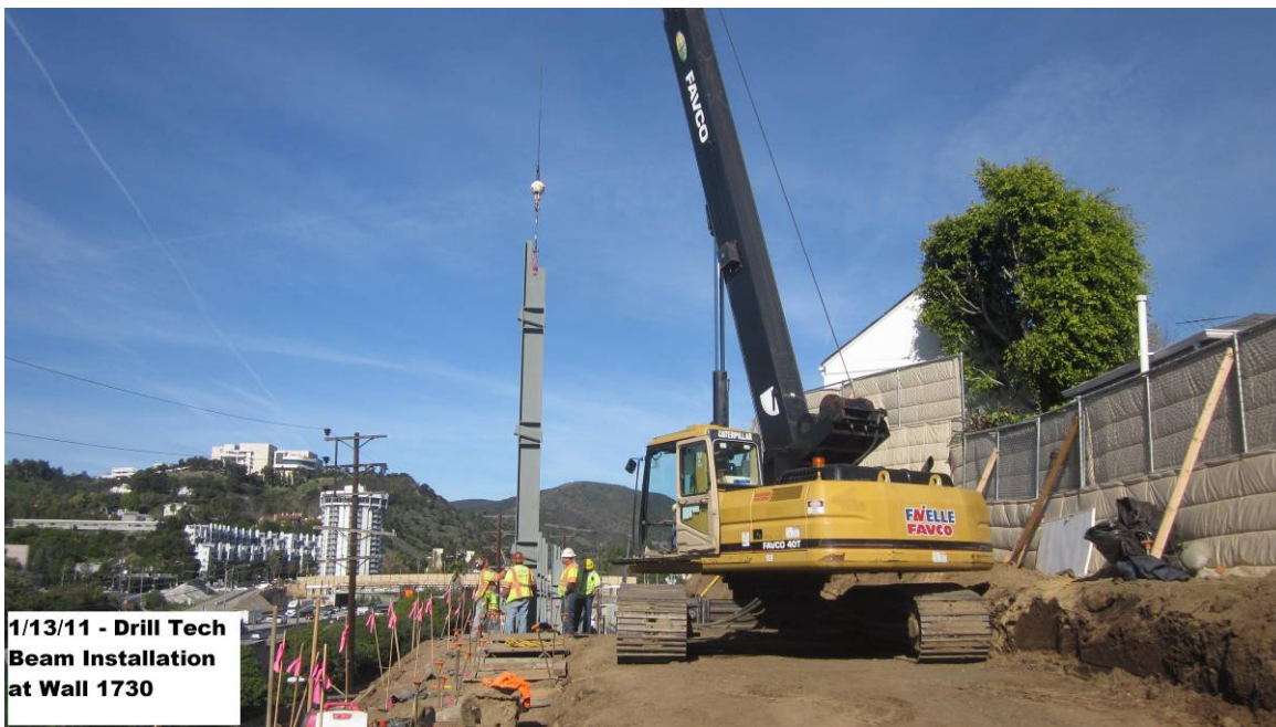
Drill tech beam installation at Wall 1730.
