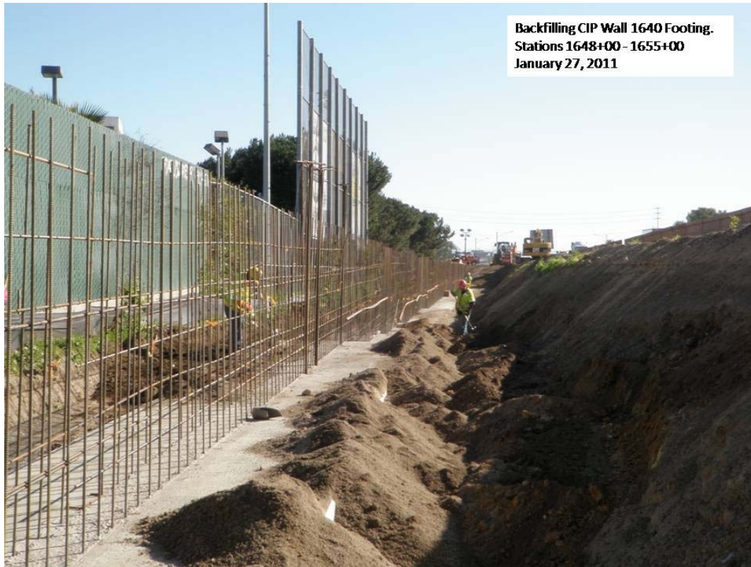
Backfilling CIP Wall 1640 footing. Stations 1648+00 – 1655+00.
