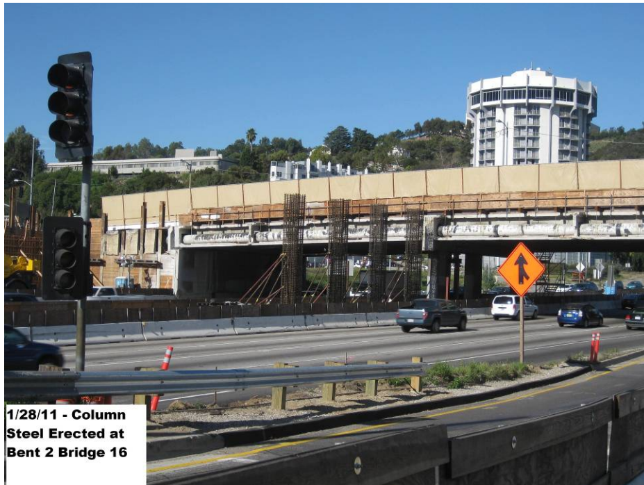
Column steel erected at Bent 2 Bridge 16.
