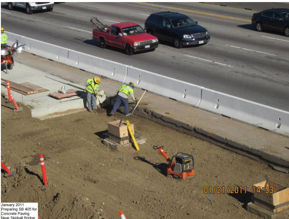
Preparing SB 405 for concrete paving near Skirball Bridge.
