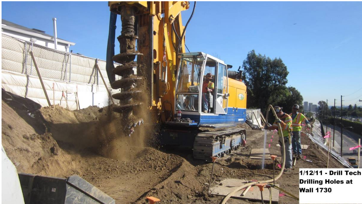
Drill tech drilling holes at Wall 1730.
