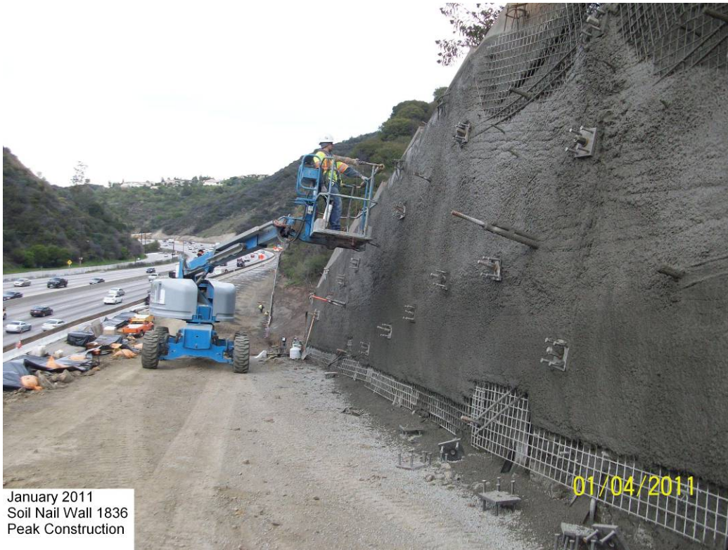
Soil Nail Wall 1836 peak construction.
