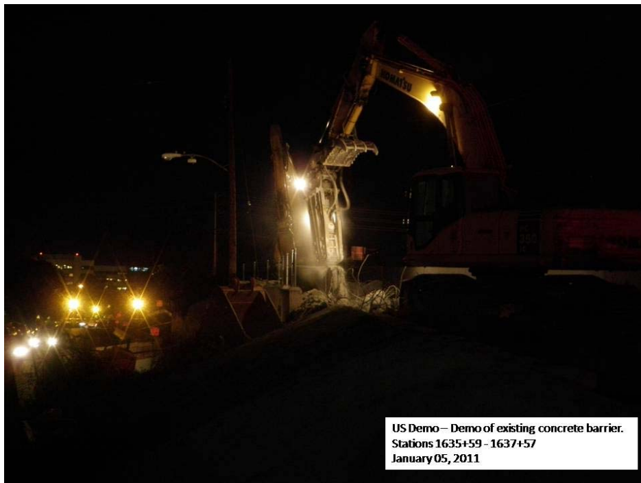
US demo – demo of existing concrete barrier. Stations 1635+59 – 1637+57.
