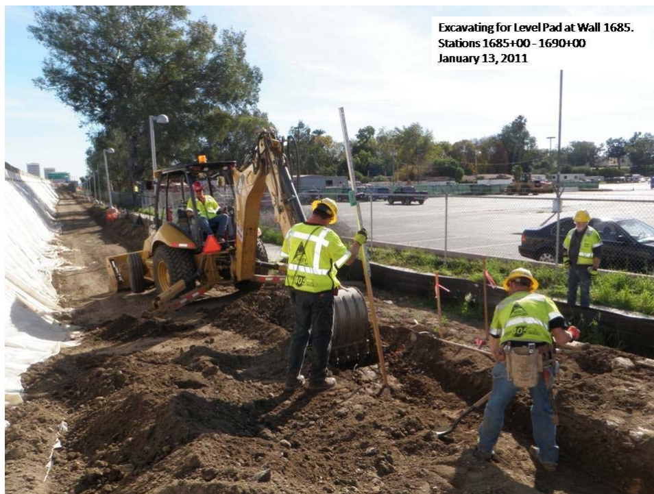
Excavating for level pad at Wall 1685, stations 1685+00 – 1690+00.
