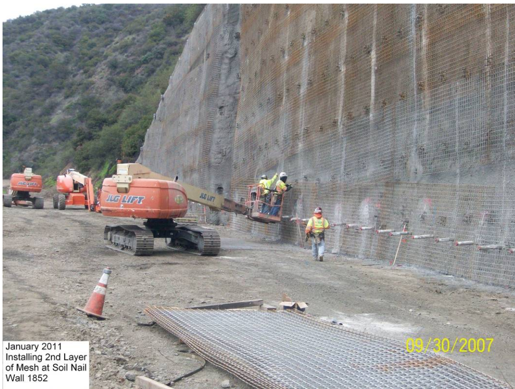
Installing 2 nd layer of mesh at Soil Nail Wall 1852.
