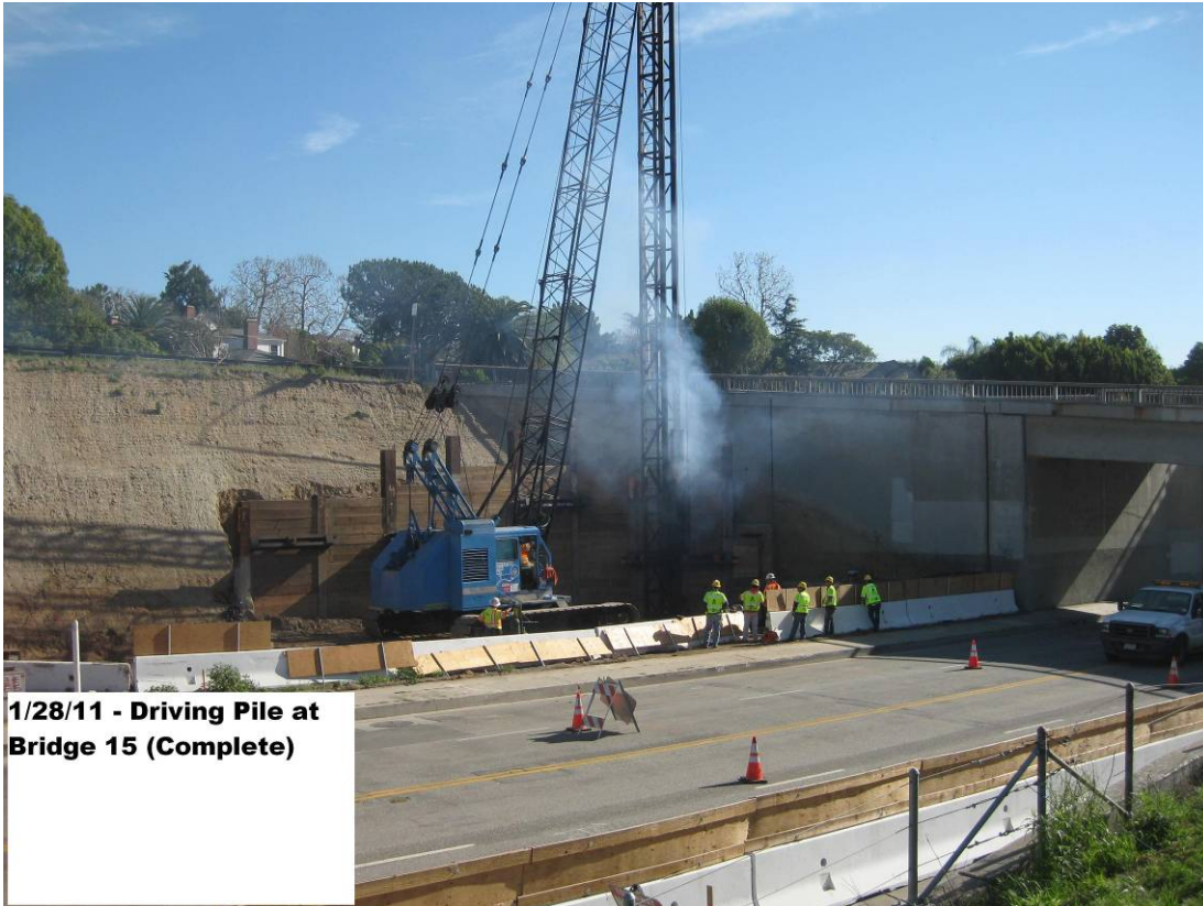
Driving pile at Bridge 15 (complete).
