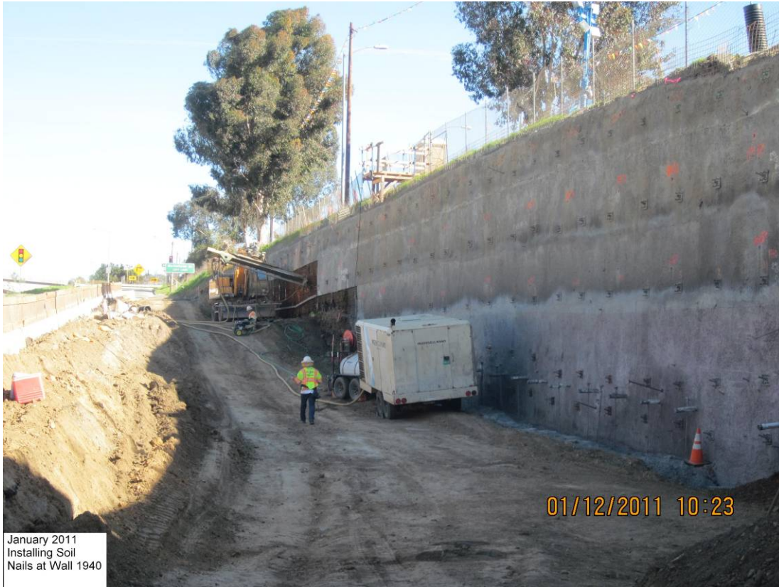
Installing soil nails at Wall 1940.
