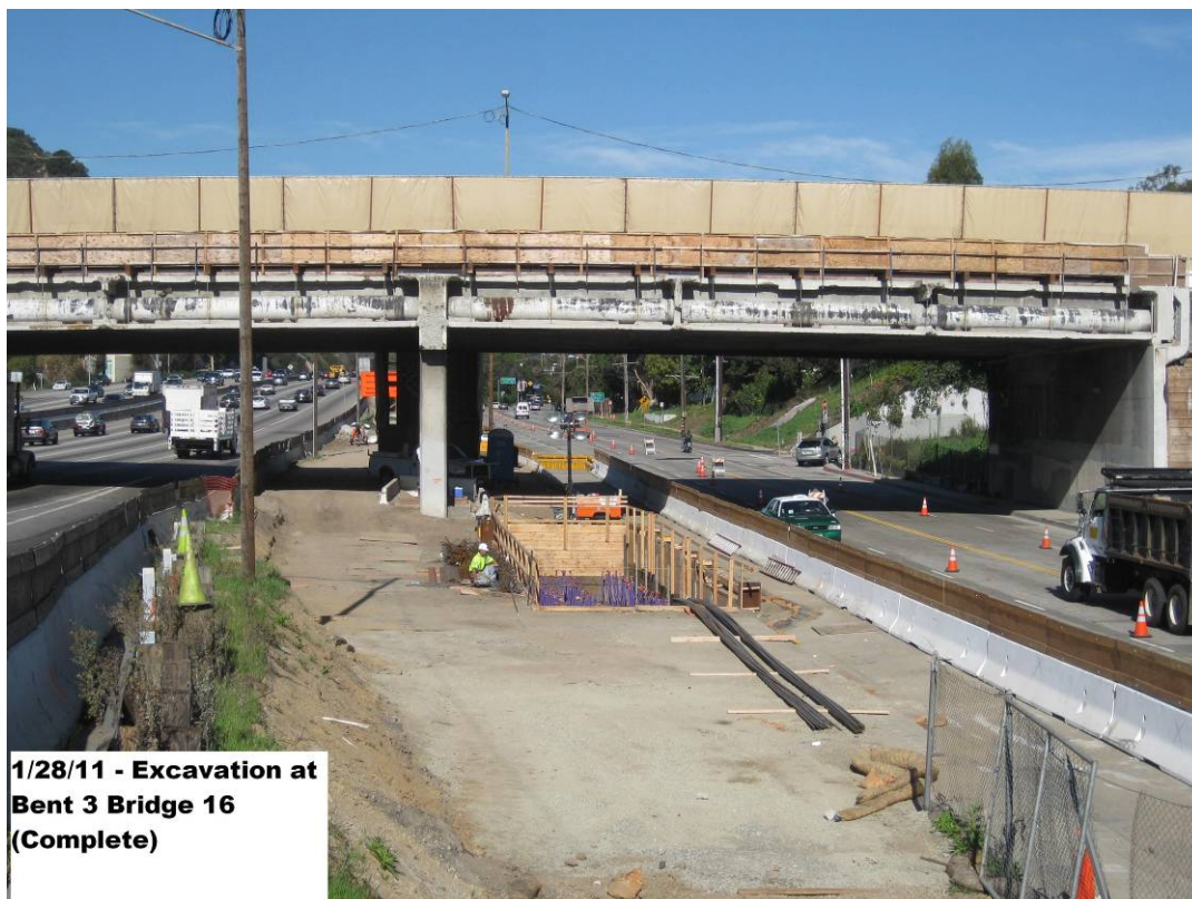
Excavation at Bent 3 Bridge 16 (complete).
