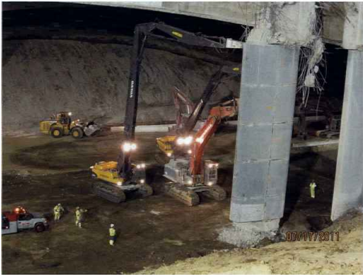
Mulholland Bridge demolition.
