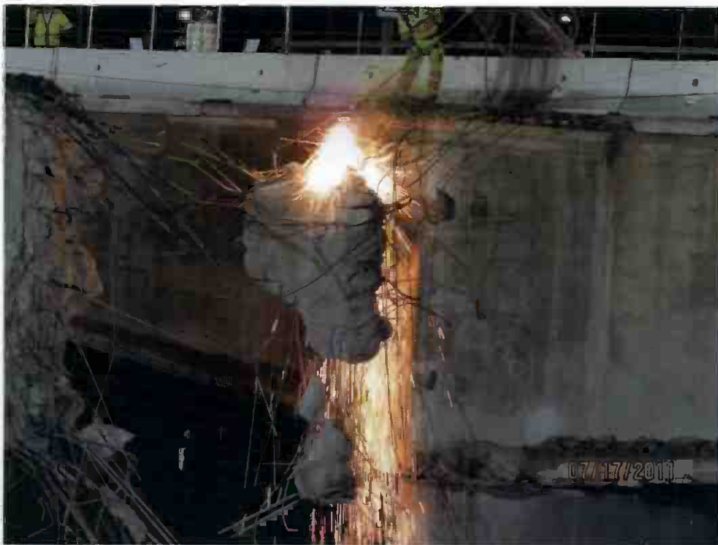
Mulholland Bridge demolition.
