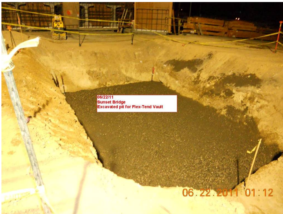
Sunset Bridge excavated pit for Flex-Tend Vault.
