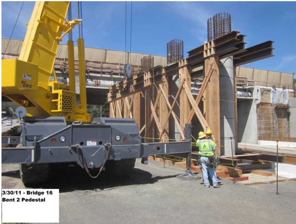
Bridge 16 Bent 2 pedestal.
