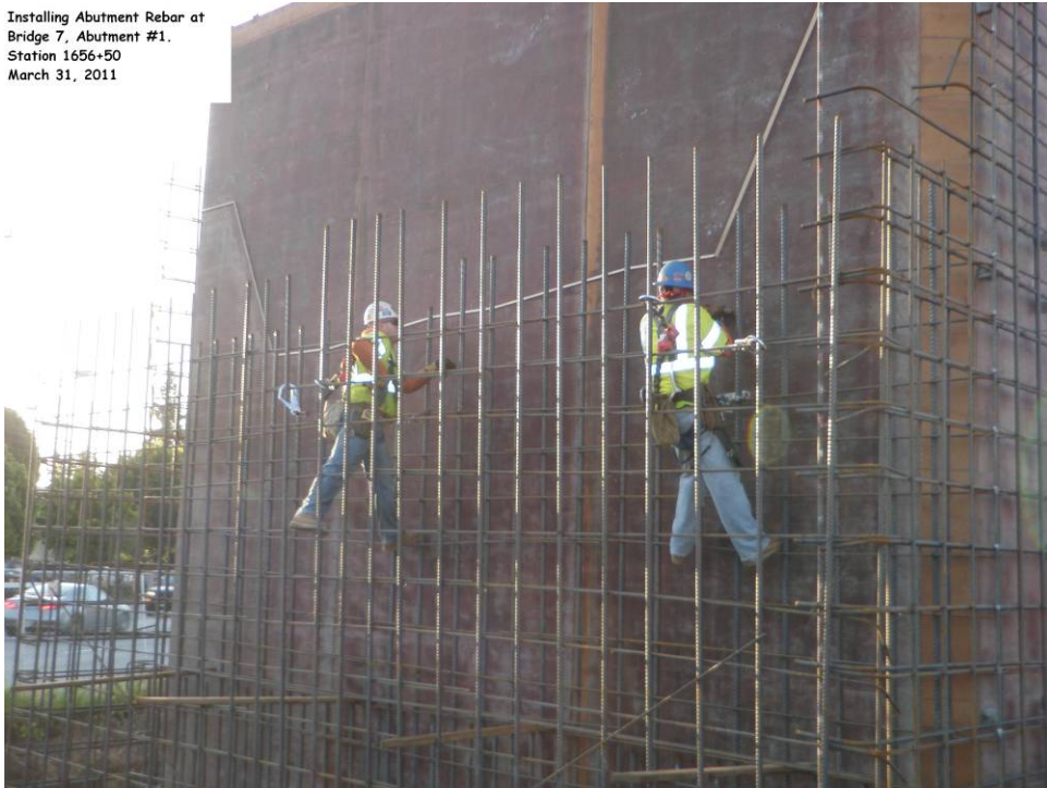
Installing abutment rebar at Bridge 7, Abutment 1 Stations 1656+50.
