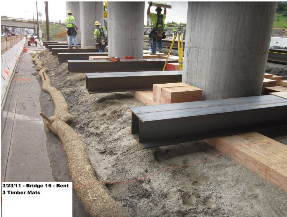
Bridge 16 Bent 3 timber mats.
