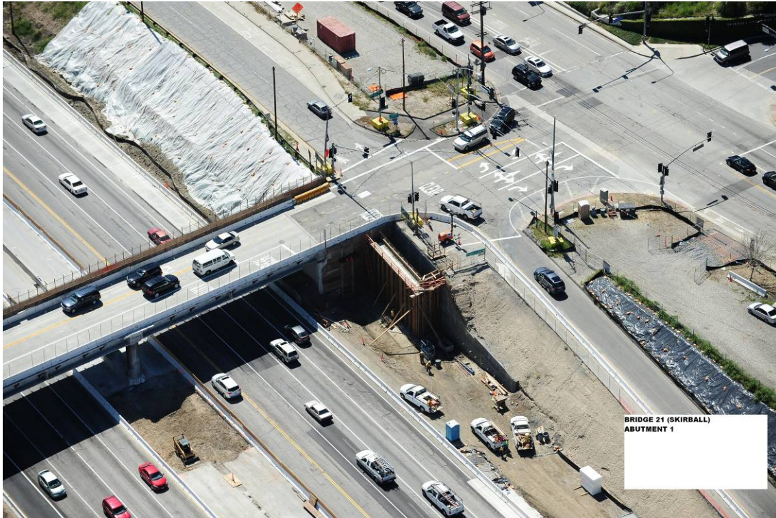
Bridge 21 (Skirball) Abutment 1.
