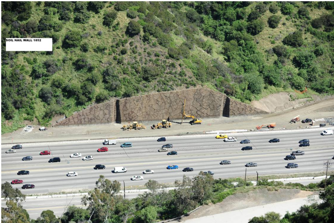
Soil Nail Wall 1852.
