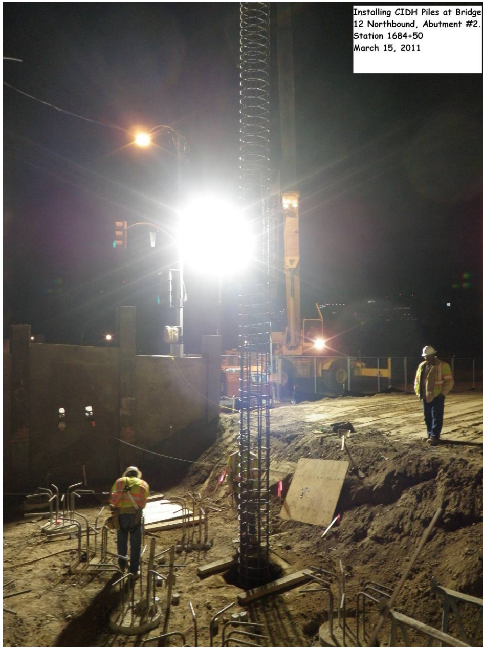
Installing CIDH piles at Bridge 12 northbound, Abutment 2 Station 1684+50.
