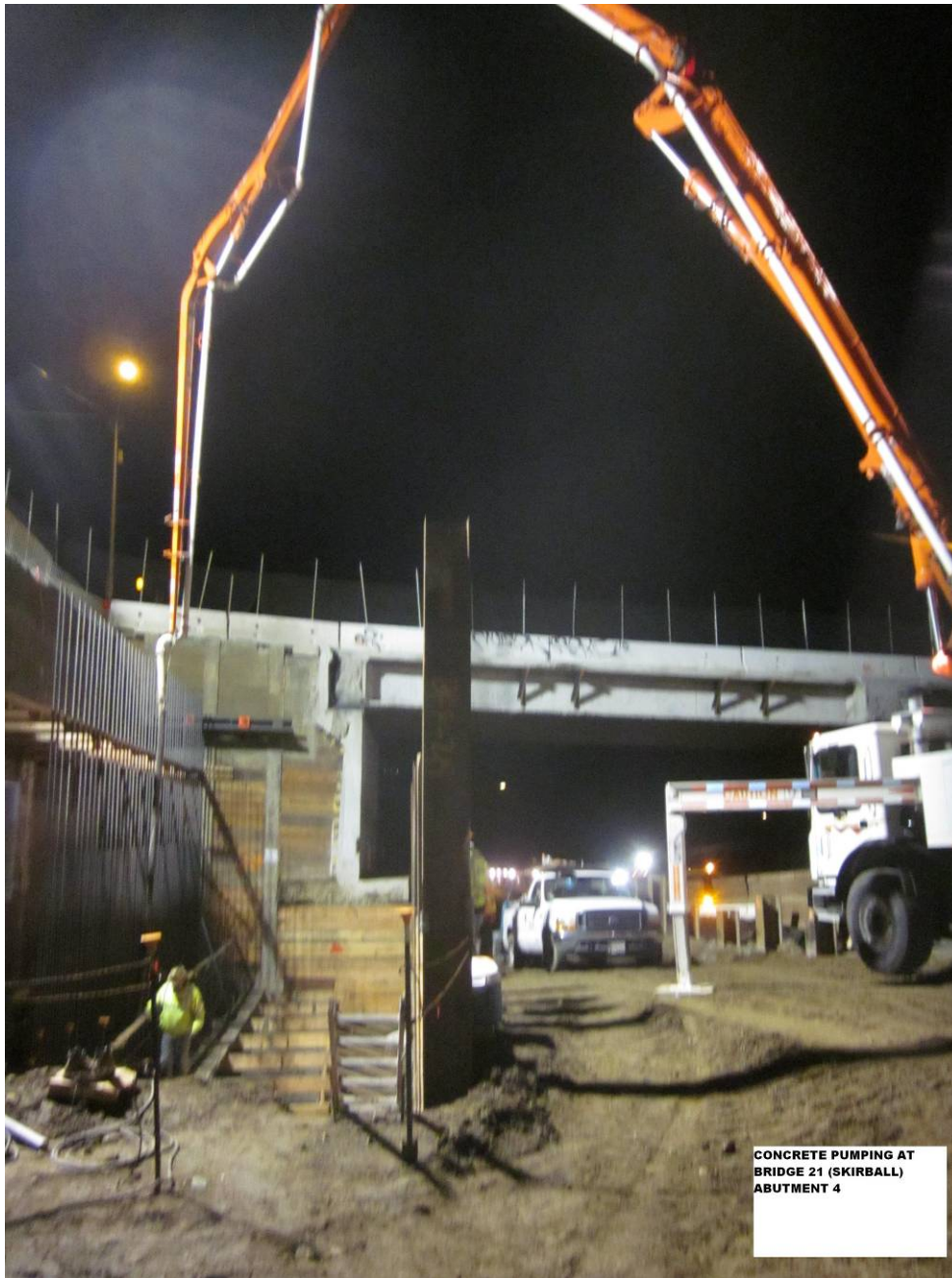
Concrete pumping at Bridge 21 (Skirball) Abutment 4.
