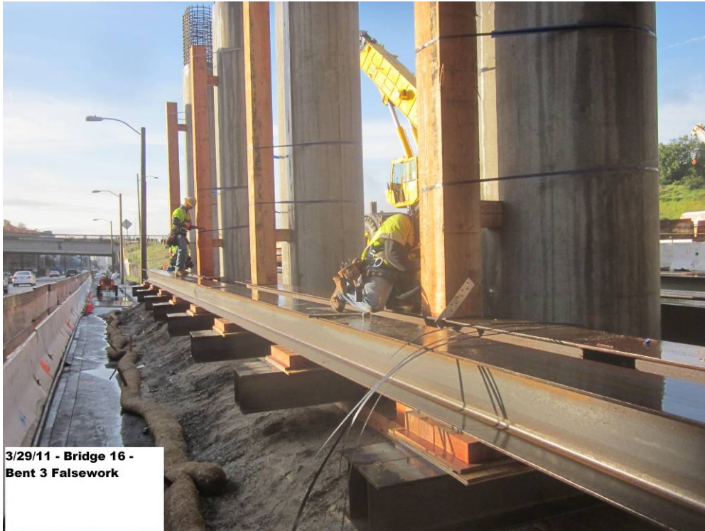
Bridge 16 Bent 3 falsework.
