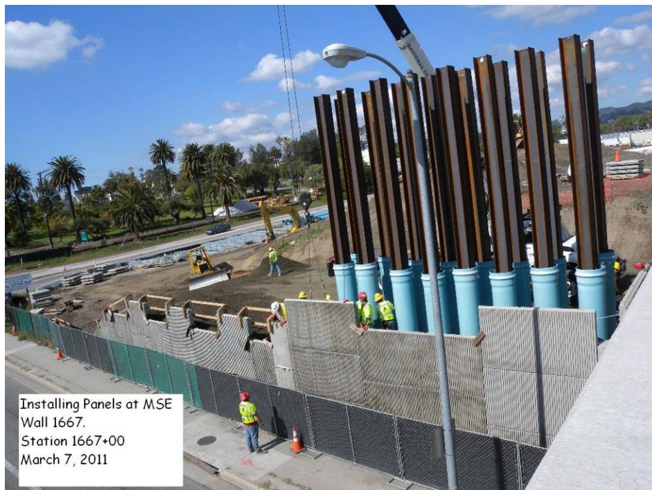
Installing panels at MSE Wall 1667, Stations 1667+00.
