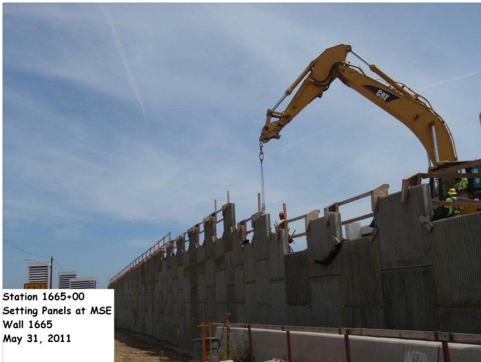
Station 1665+00. Setting panels at MSE Wall 1665.
