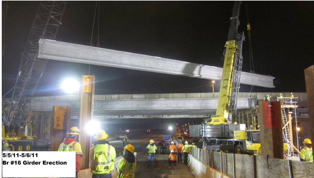
Bridge 16 girder erection.
