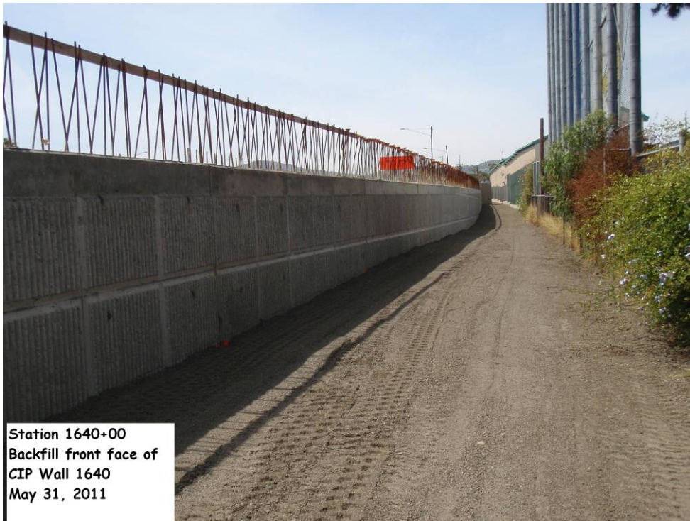
Station 1640+00 backfill front face of CIP Wall 1640.
