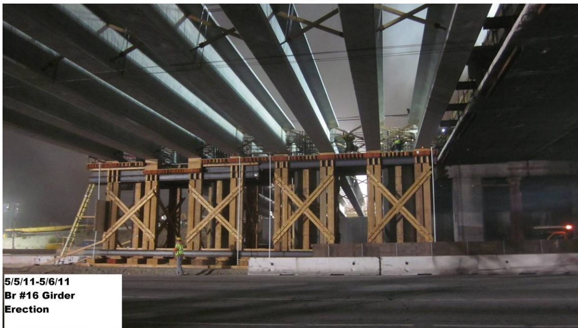
Bridge 16 girder erection.
