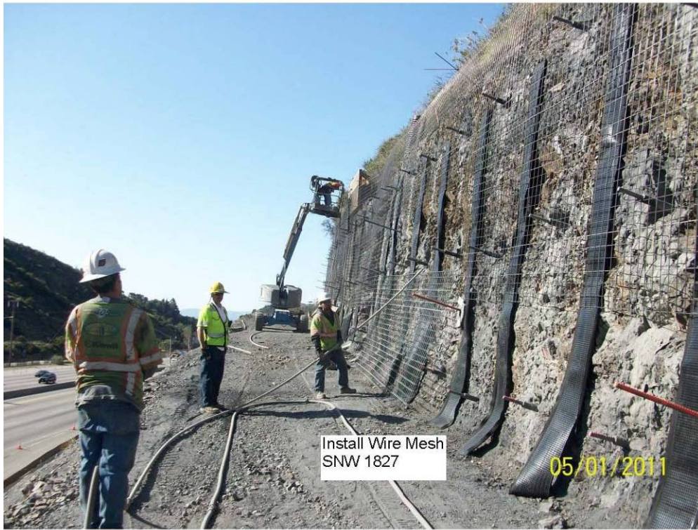
Install wire mesh SNW 1827.
