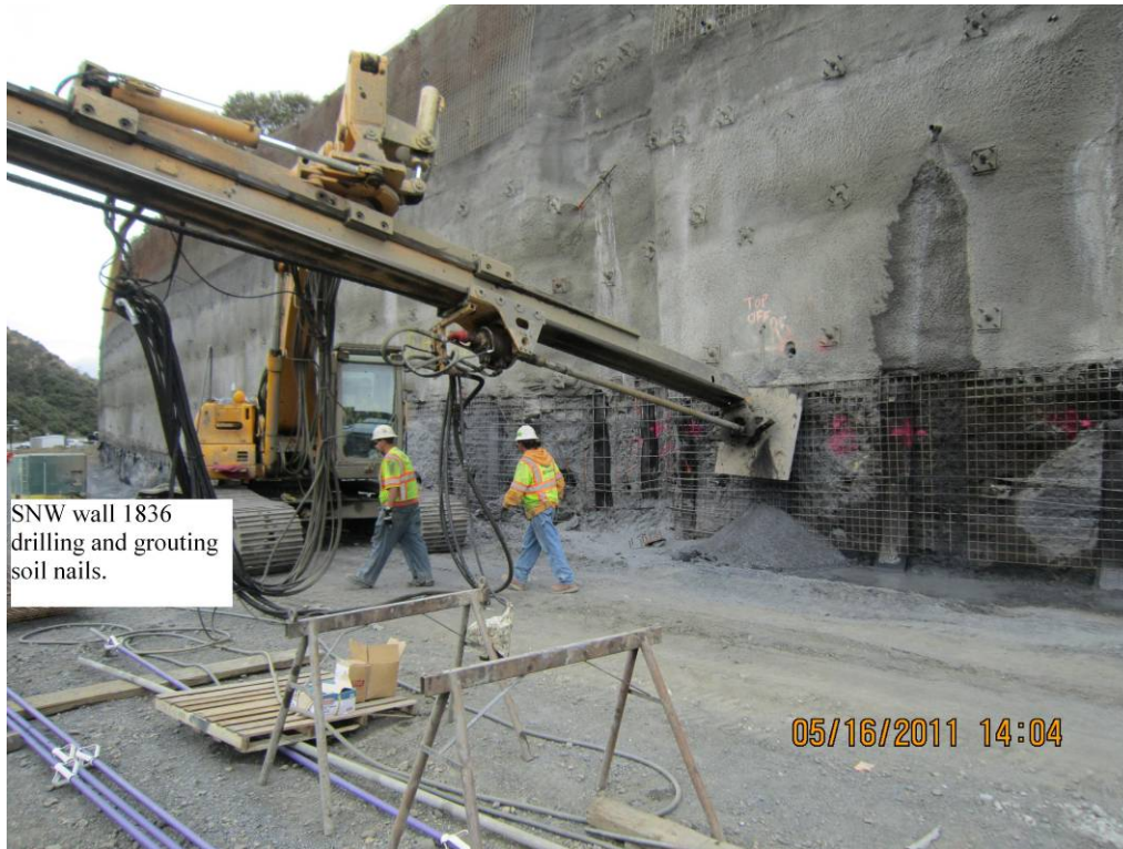
SNW Wall 1836 drilling and grouting soil nails.
