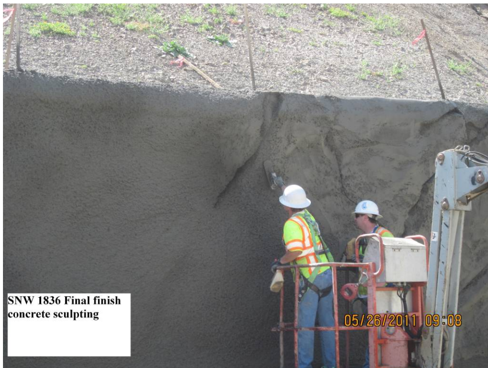
SNW 1836 final finish concrete sculpting.
