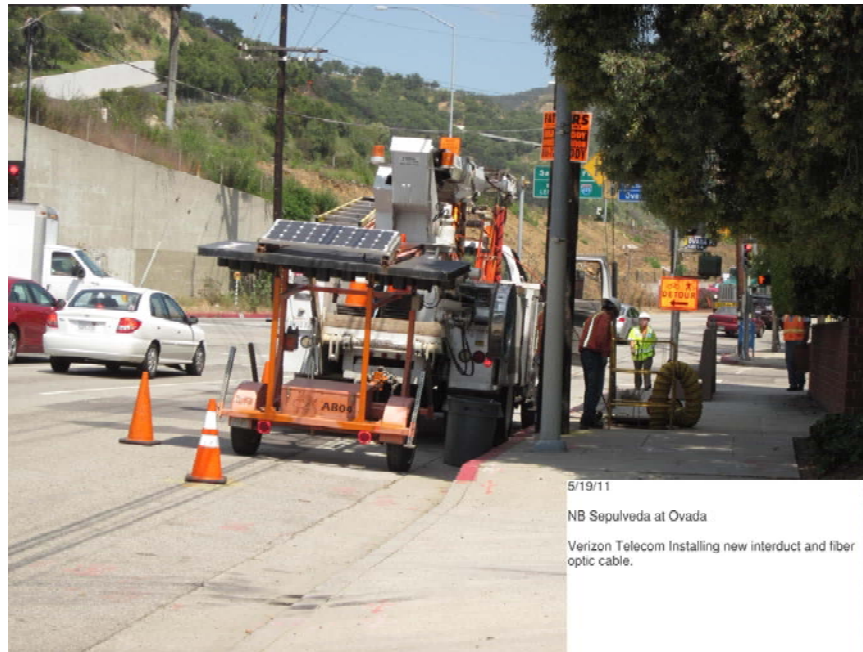
Verizon Telecom installing new interduct and fiber optic cable.
