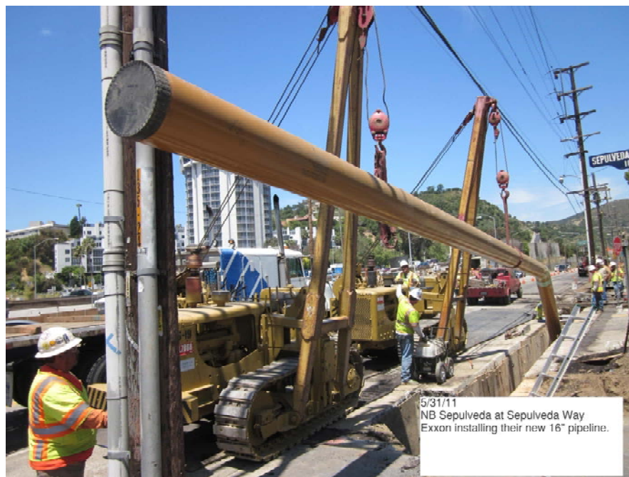
Exxon installing their new 16" pipeline.
