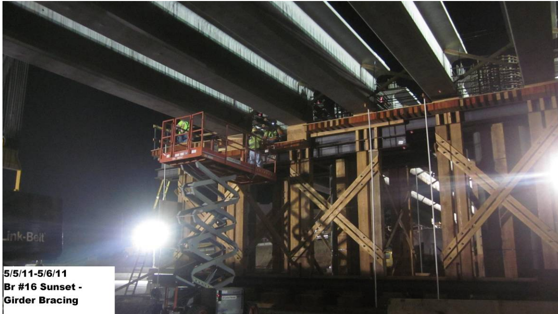
Bridge 16 Sunset girder bracing.
