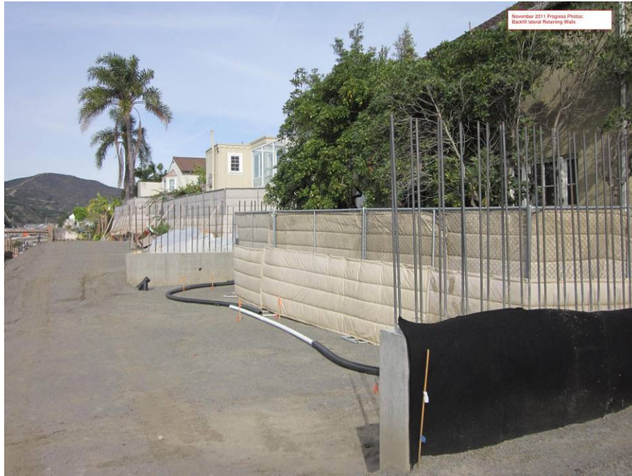
Backfill lateral retaining walls.
