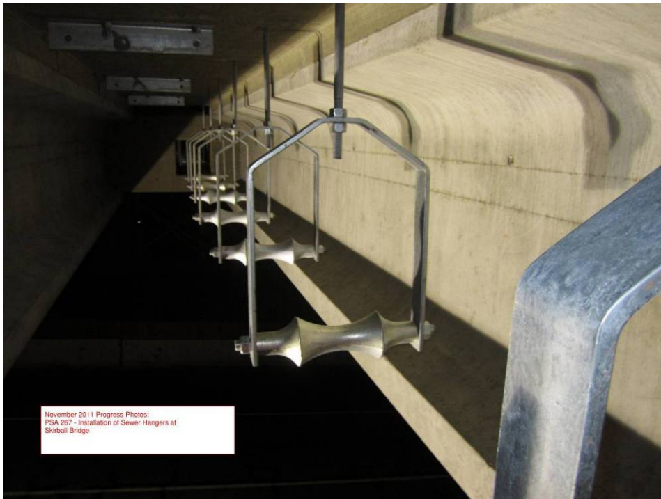
PSA 267 – Installation of sewer hangers at Skirball Bridge.
