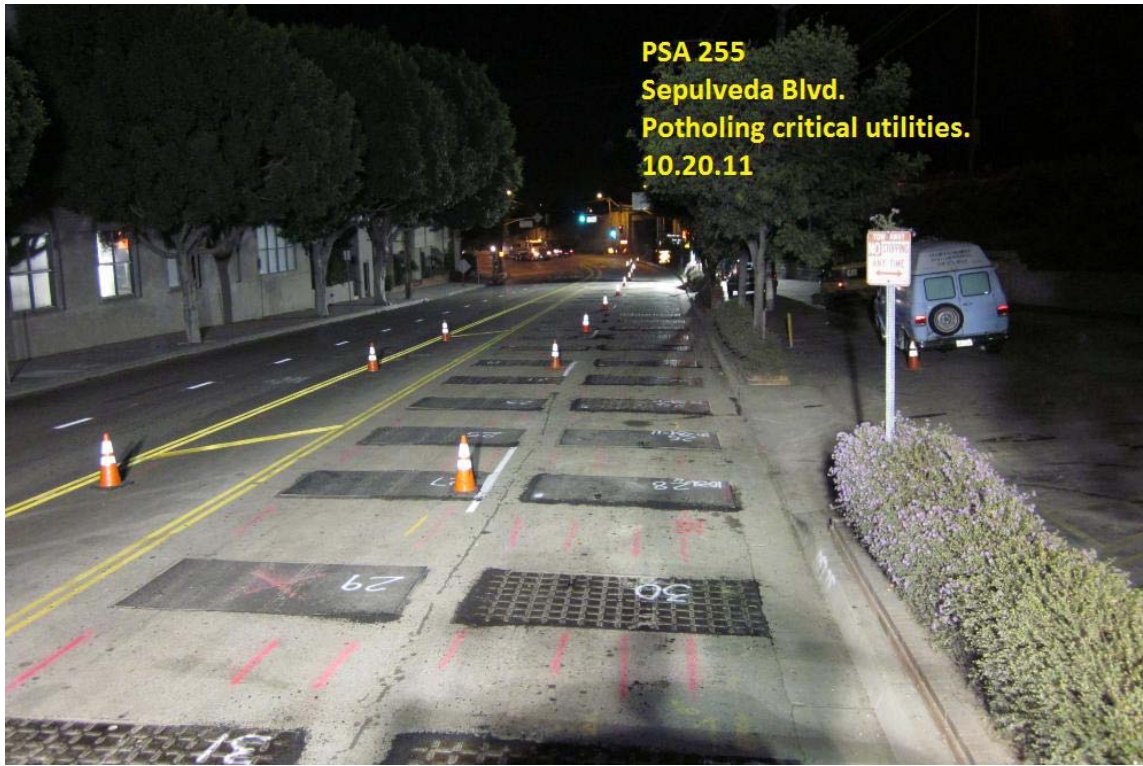
PSA 255 Sepulveda Blvd. potholing critical utilities.
