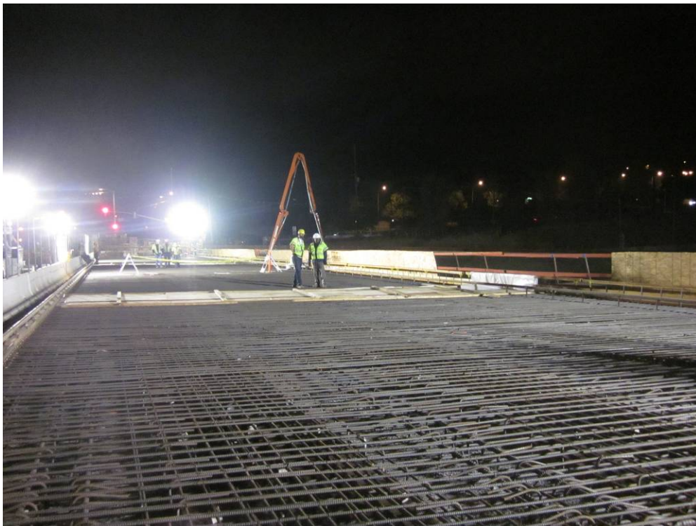
Skirball Bridge deck pour.
