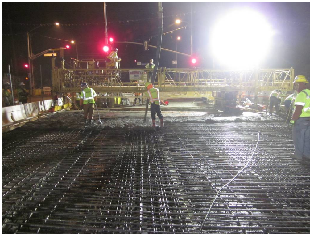
Skirball Bridge deck pour.
