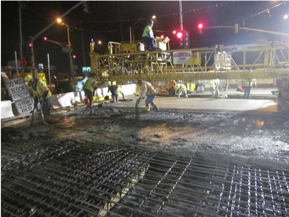
Skirball Bridge deck pour.
