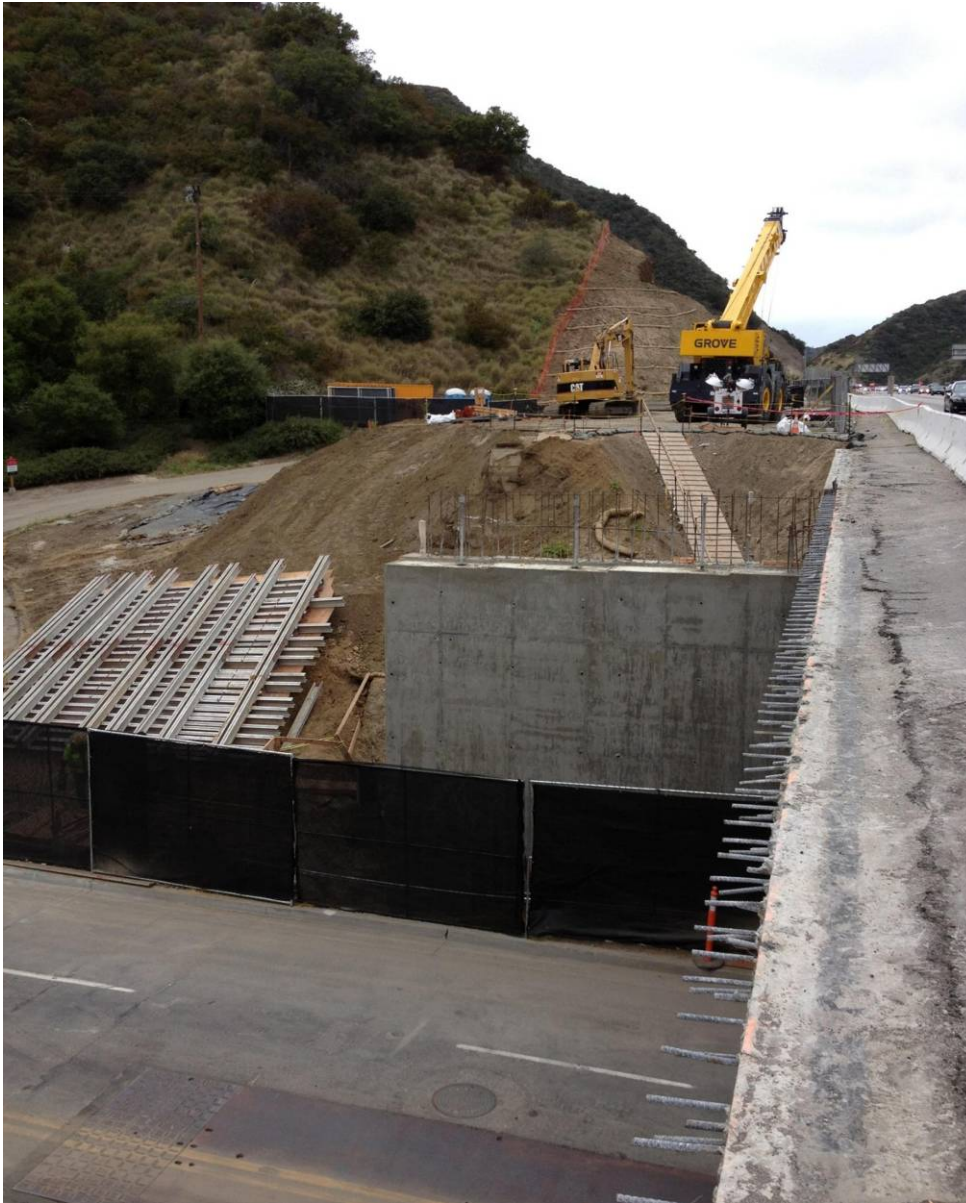
Bridge 18 Getty Center Drive UC.
