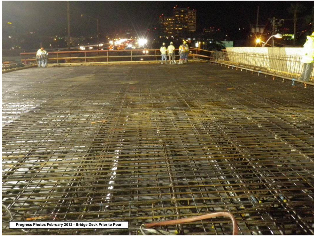
Bridge deck prior to pour.
