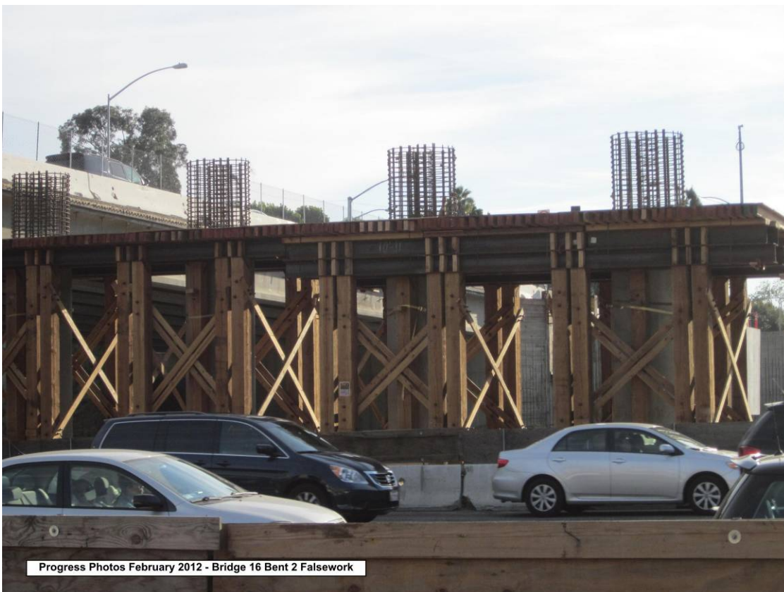
Bridge 16 Bent 2 Falsework.
