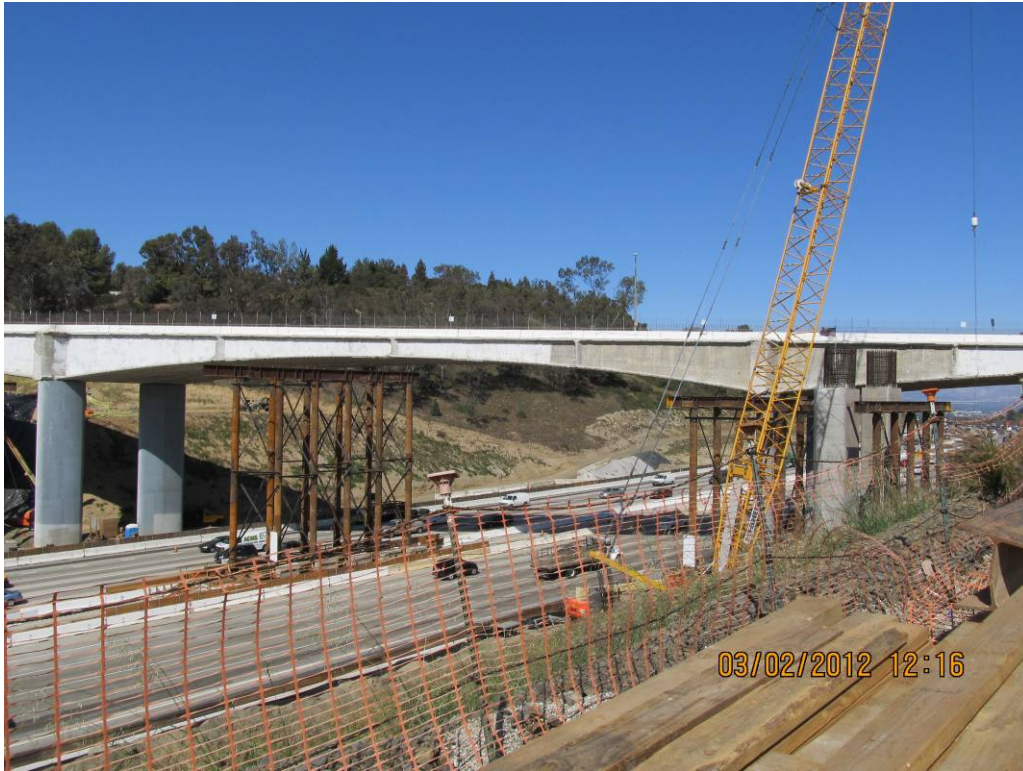
Mulholland Bridge falsework.
