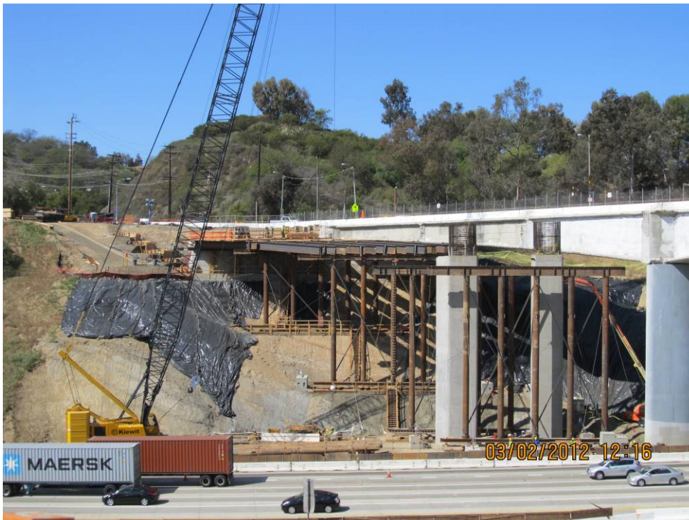
Mulholland Bridge falsework.
