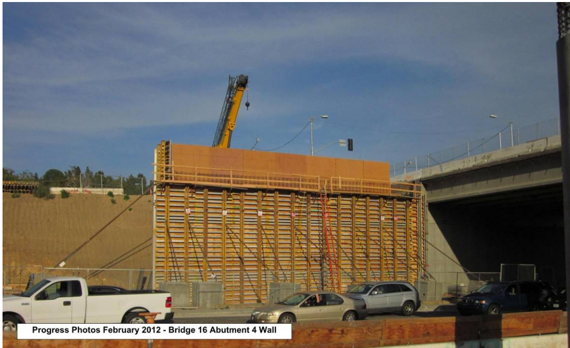
Bridge 16 Abutment 4 Wall.
