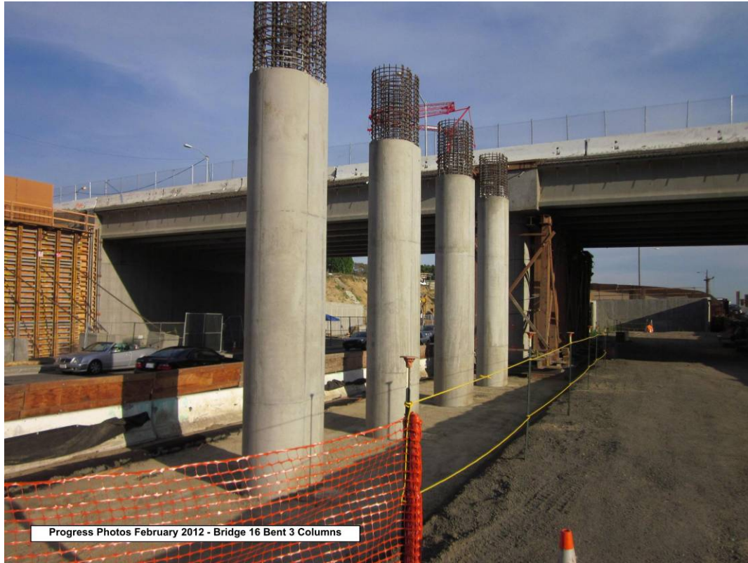
Bridge 16 Bent 3 columns.
