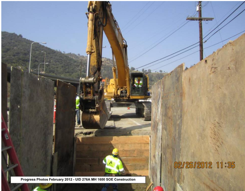
UID 276A MH 1600 SOE Construction.
