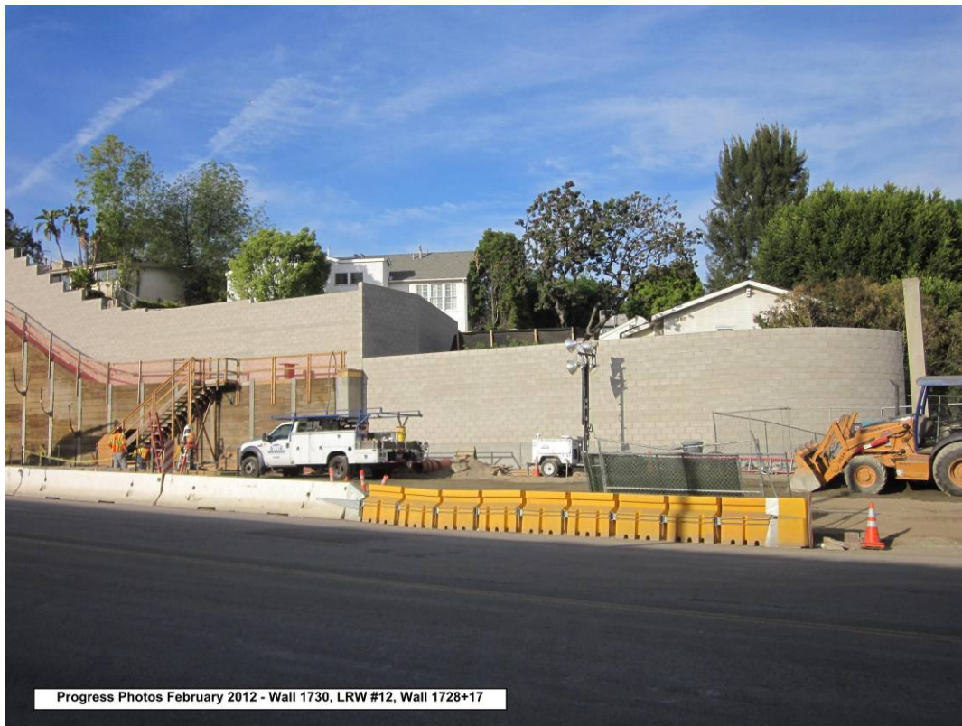
Wall 1730, LRW #12, Wall 1728+17.
