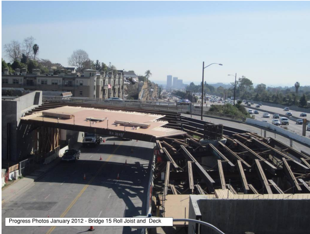
Bridge 15 roll joist and deck.
