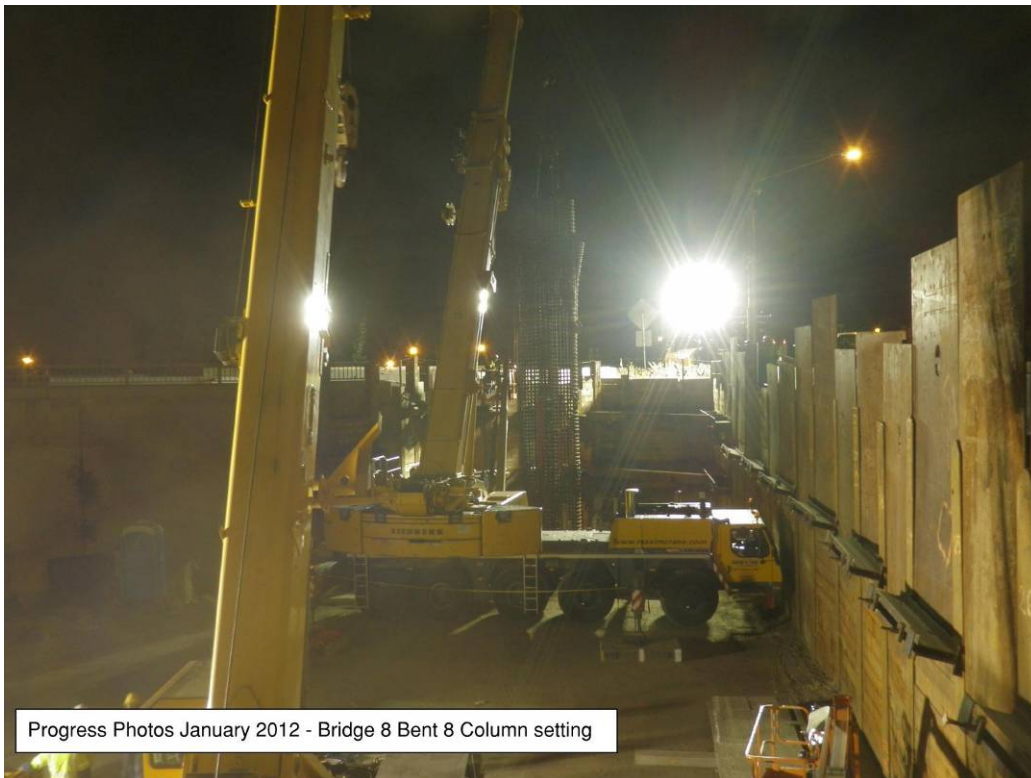
Bridge 8 Bent 8 column setting.
