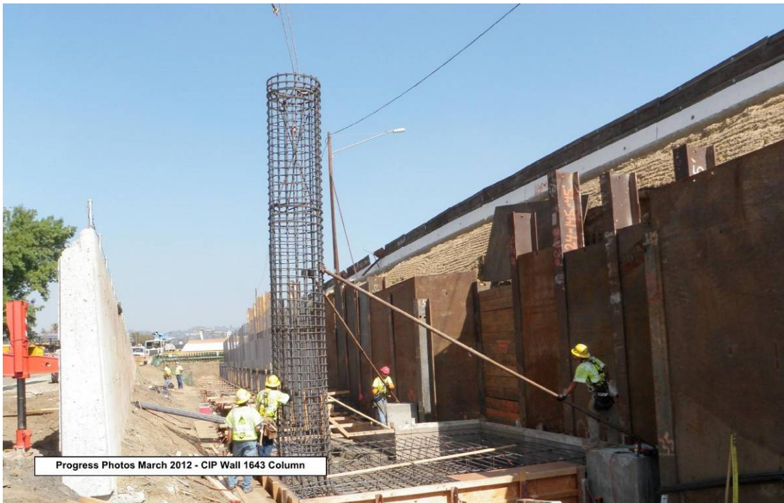
CIP Wall 1643 Columns.
