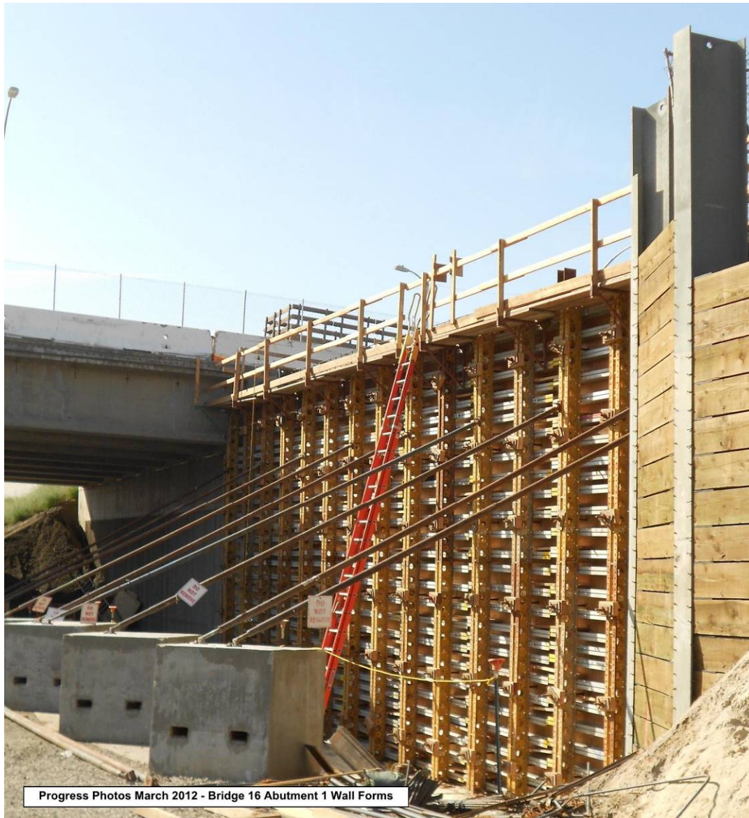
Bridge 16 Abutment 1 Wall Forms.
