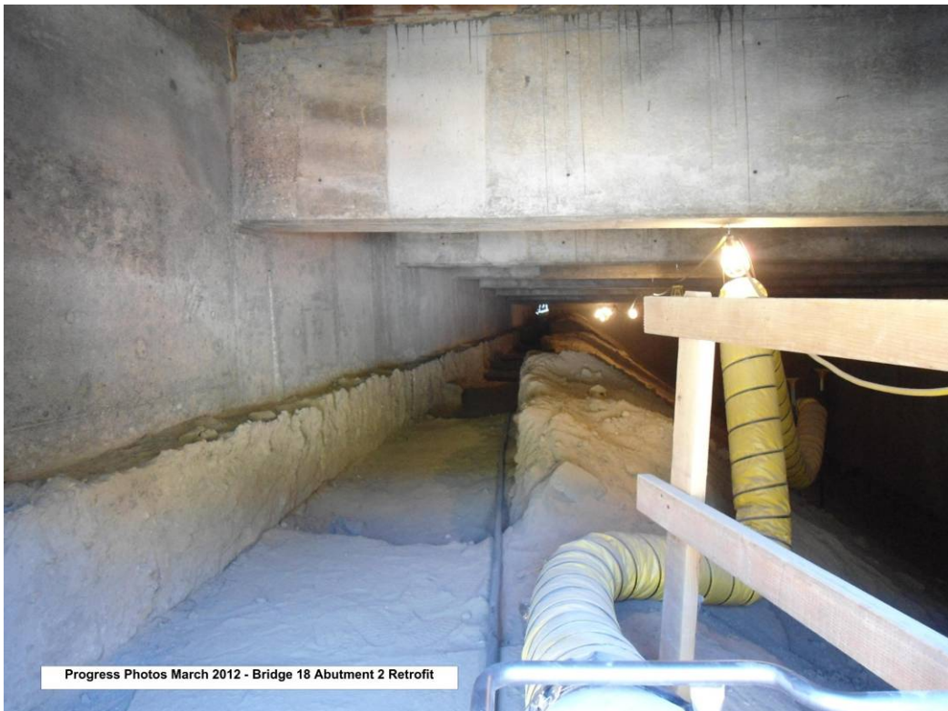
Bridge 18 Abutment 2 Retrofit.
