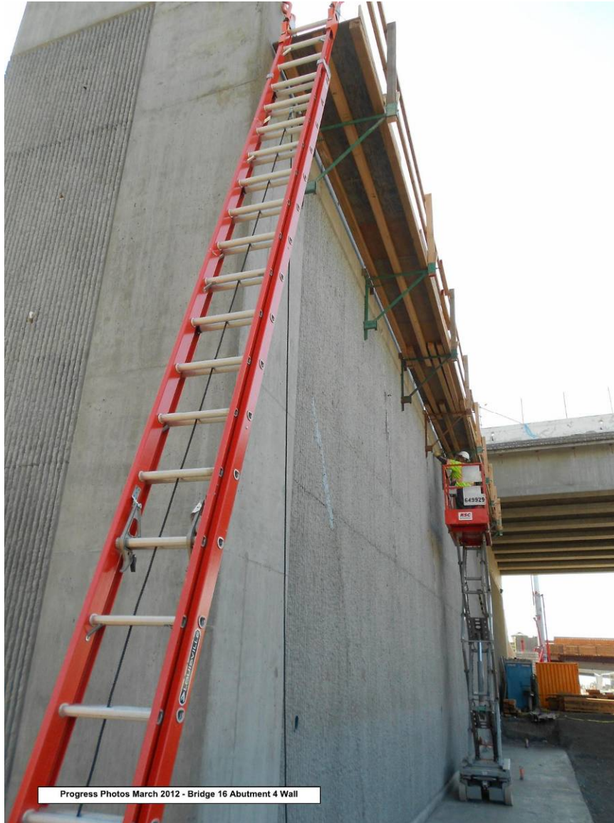
Bridge 16 Abutment 4 Wall.
