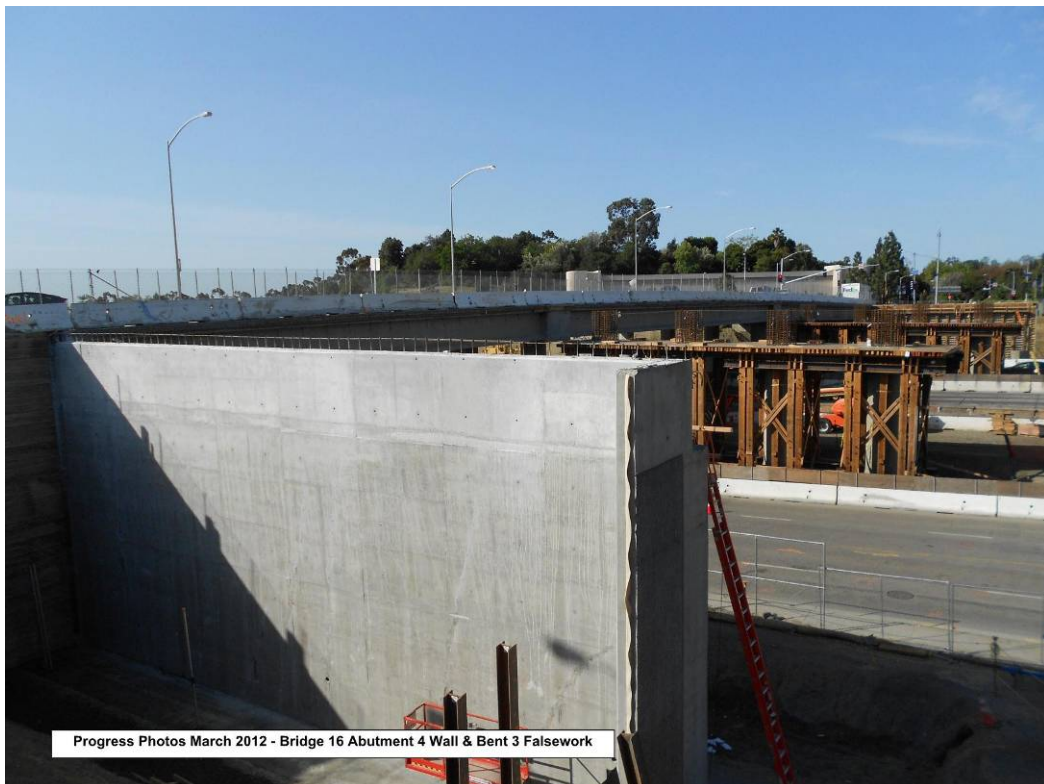
Bridge 16 Abutment 4 Wall & Bent 3 Falsework.
