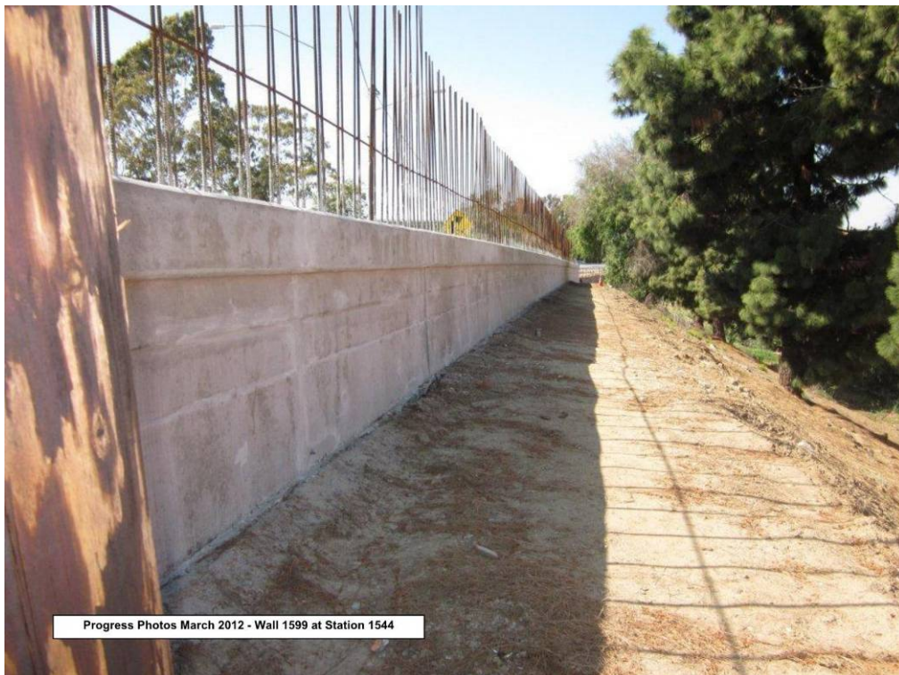
Wall 1599 at Station 1544.
