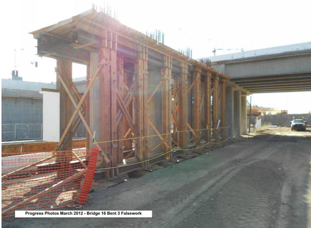
Bridge 16 Bent 3 Falsework.
