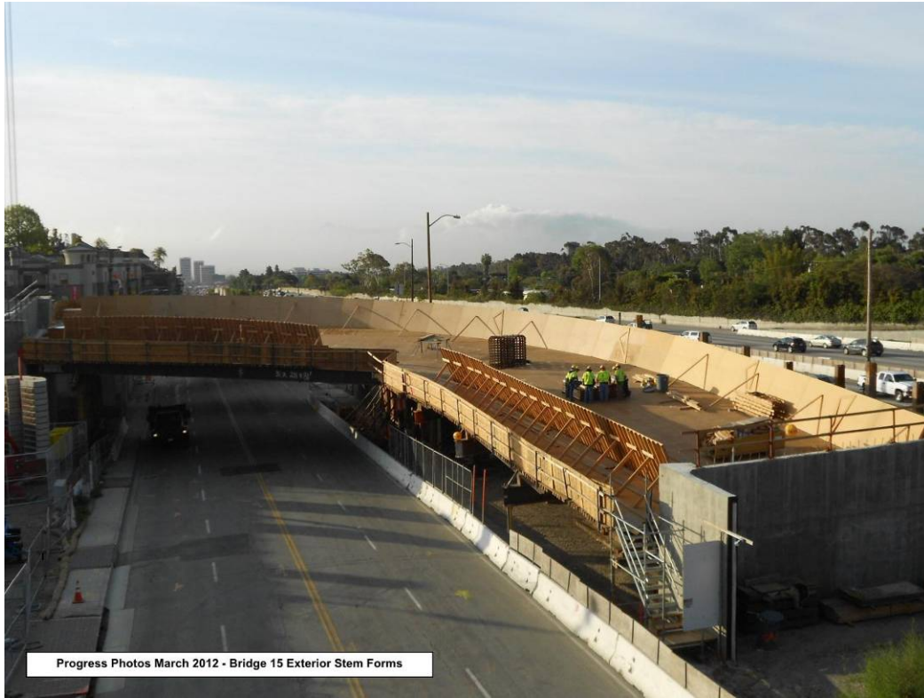
Bridge 15 exterior stem forms.
