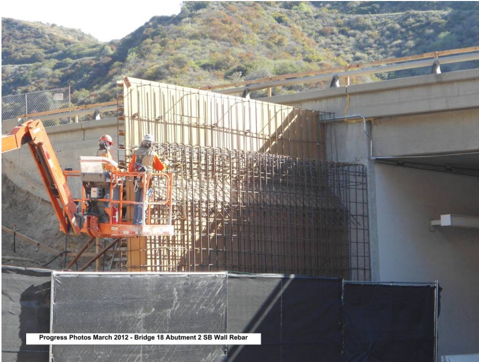
Bridge 18 Abutment 2 SB Wall Rebar.
