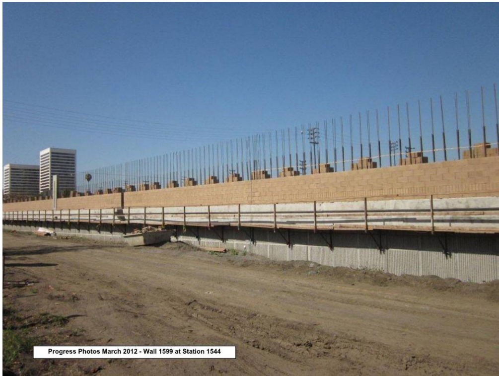
Wall 1599 at Station 1544.
