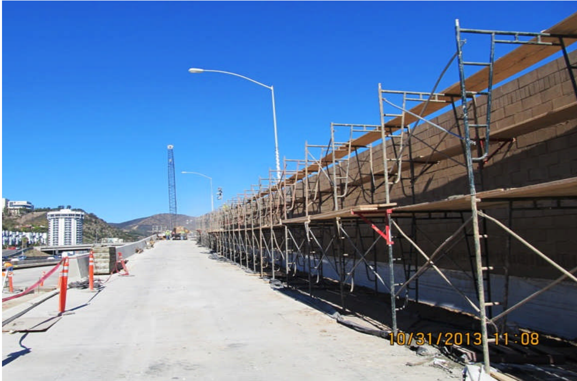
Wall 1718 Soundwall Construction.
