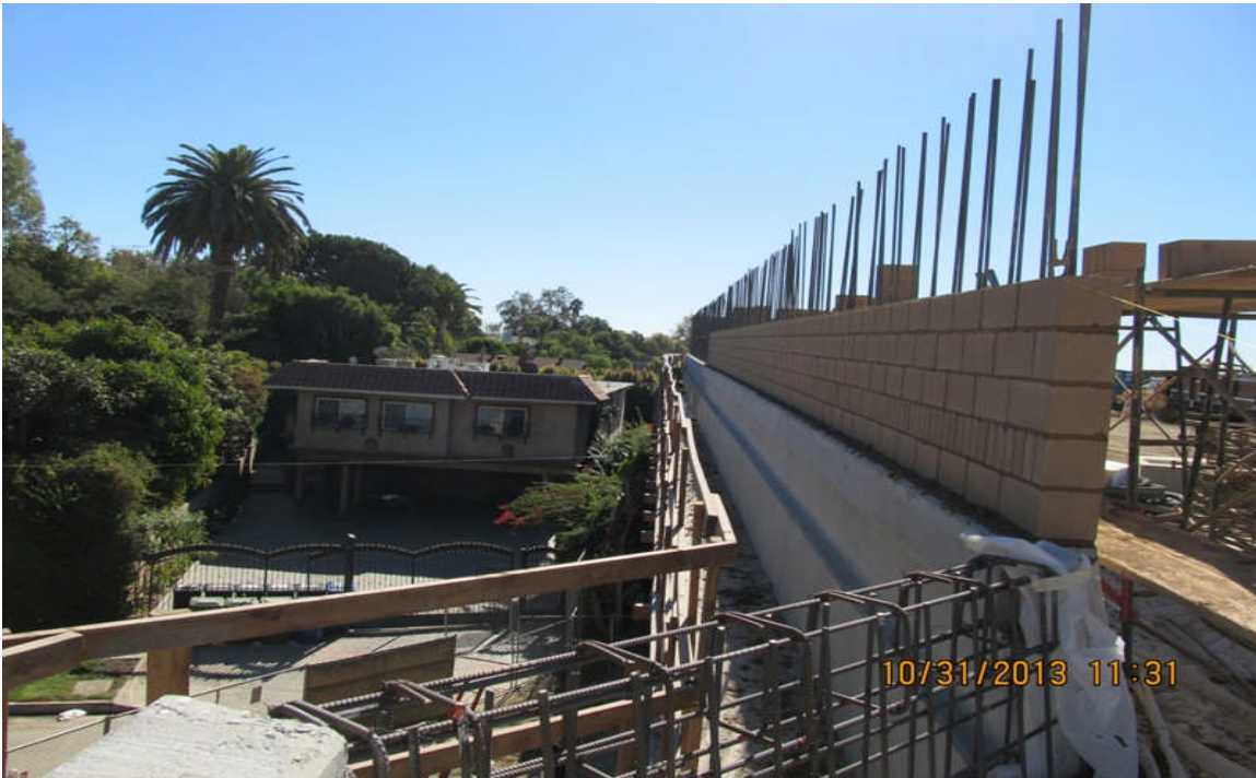
Wall 1738A Soundwall Construction.
