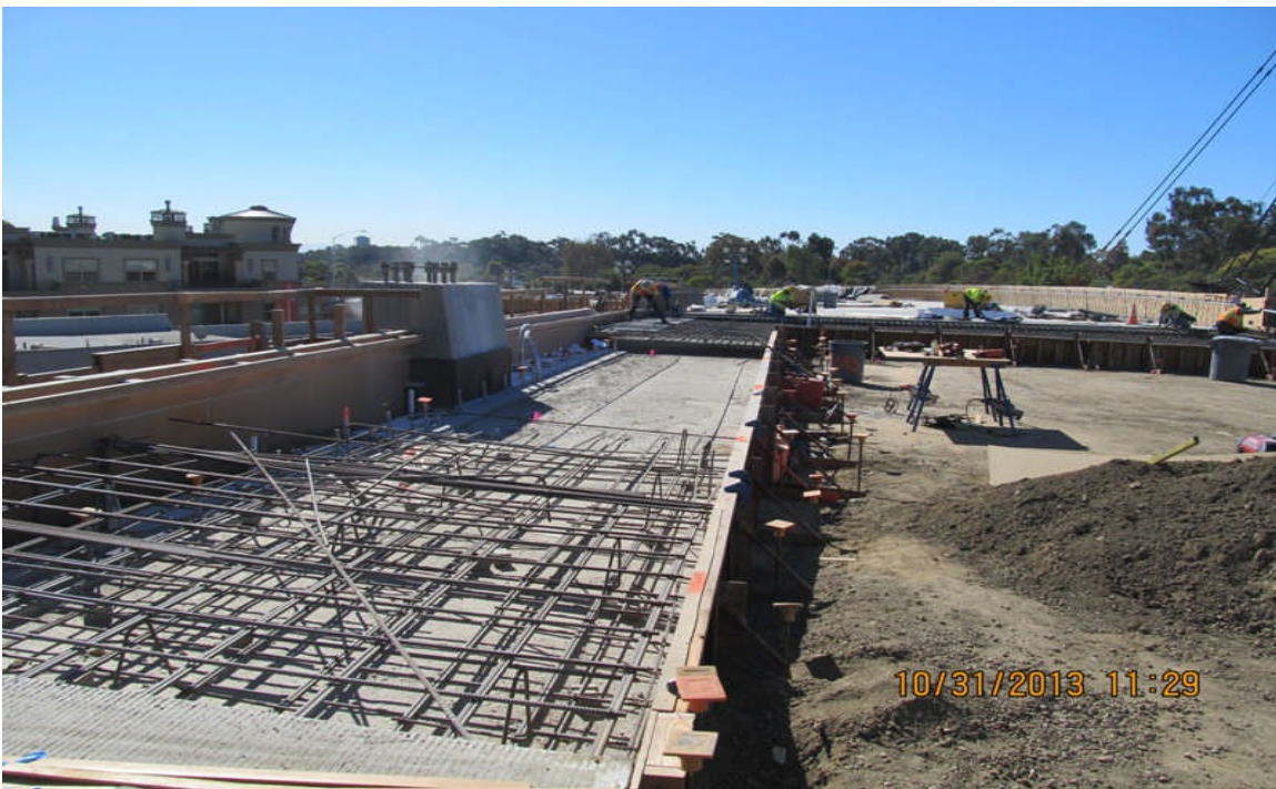
Bridge 14 Moment Slab Form and Rebar Installation.
