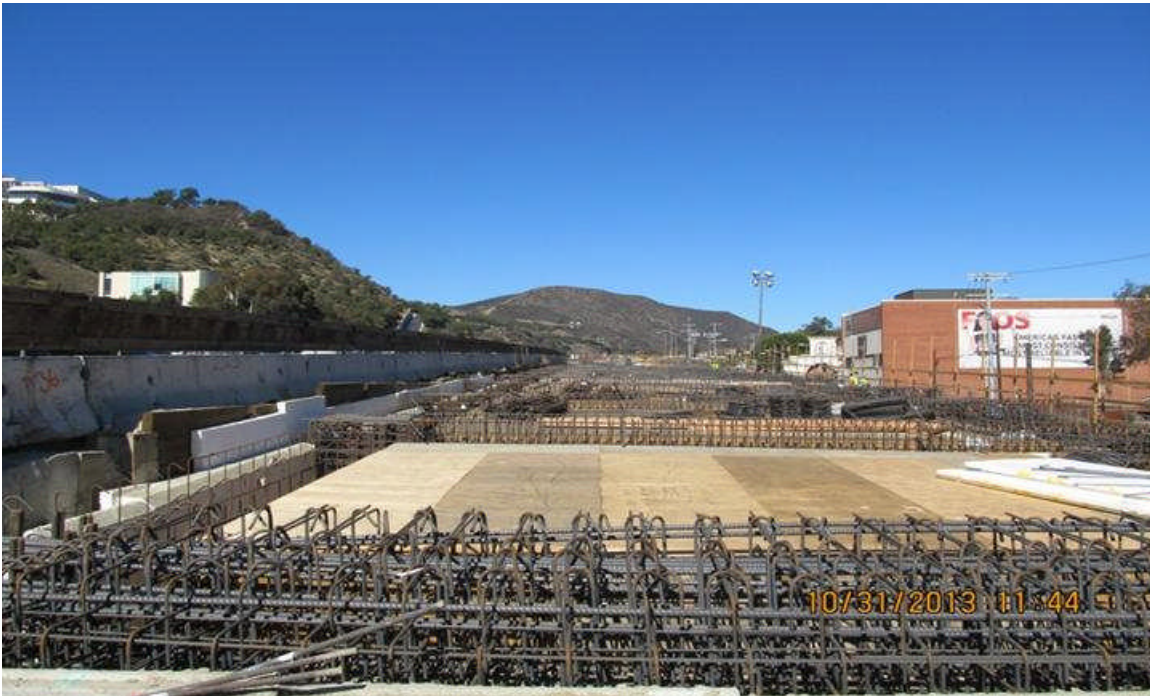
Bridge 17 Rebar Installation.
