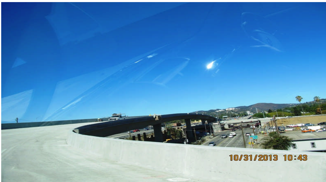
Bridge 8 Falsework Removed.
