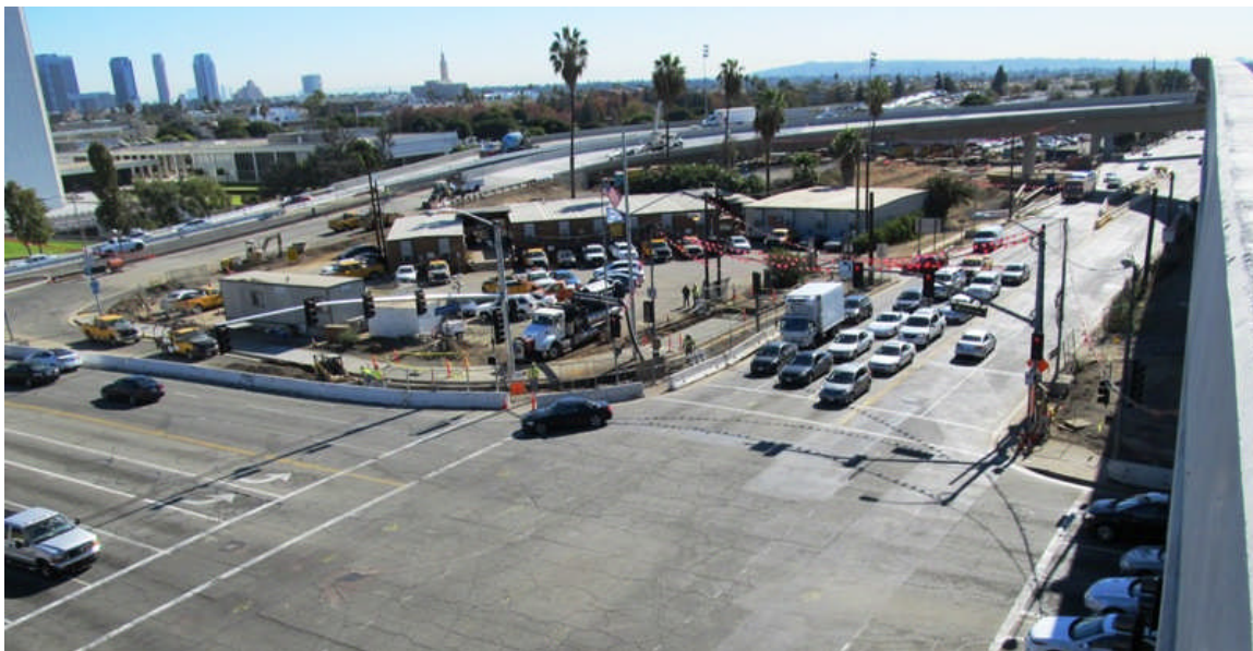
Bridge 8 - Wilshire & Sepulveda Intersection Curb & Gutter and Sidewalk construction.
