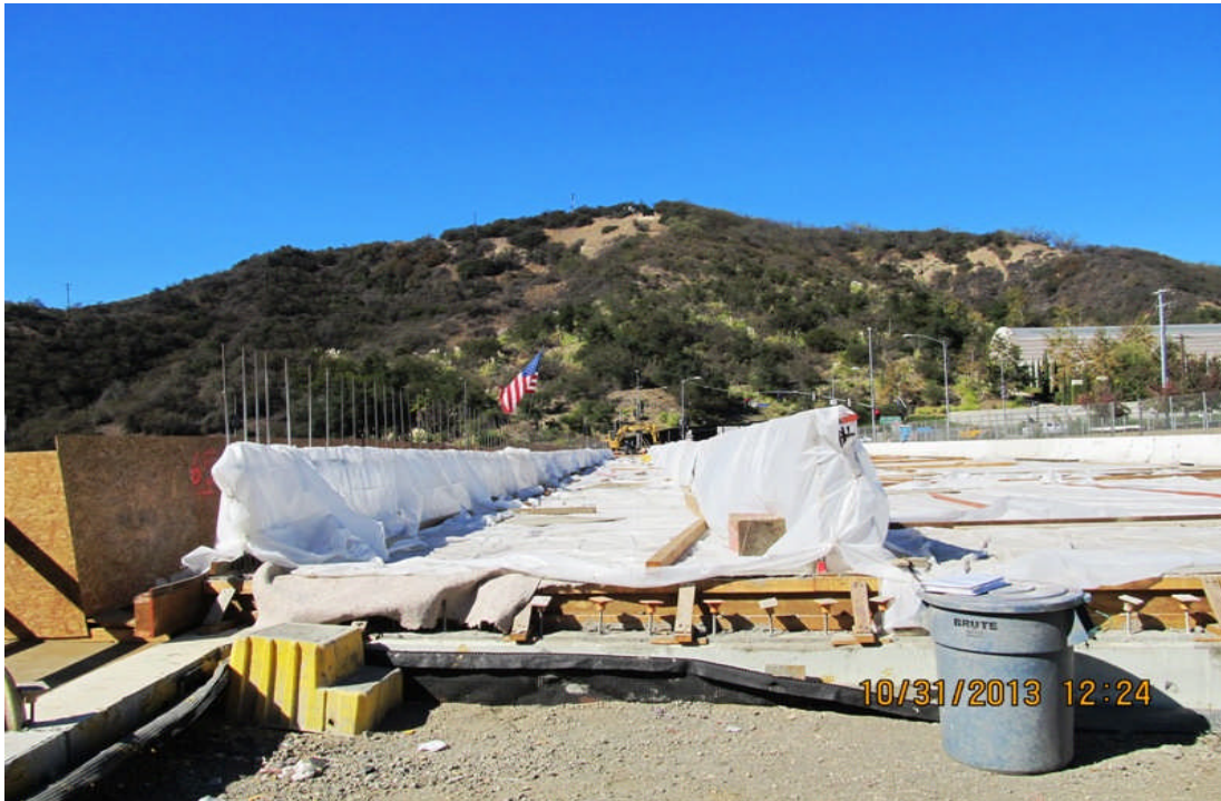
Bridge 21 Top Deck and Wildlife Crossing Poured.
