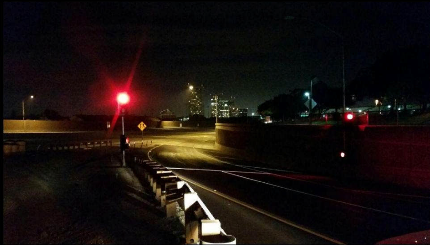
W1 Activated Ramp Metering Signals
