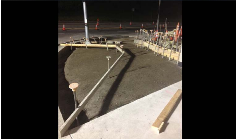
S3. Skirball and Mulholland SW Corner ADA Ramp Pre-Pour
