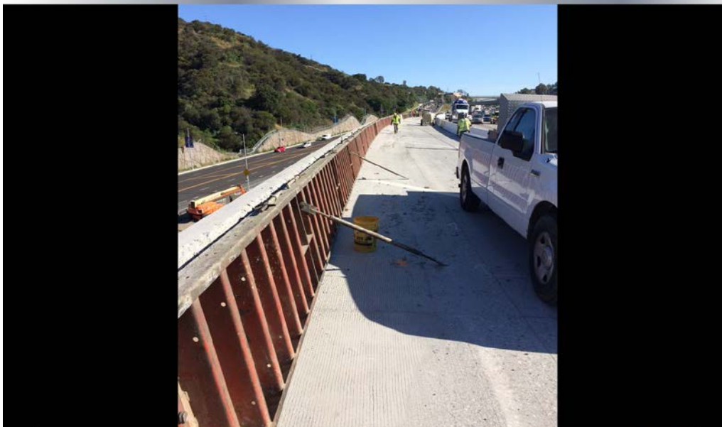
S3. 1921 Barrier Adjacent to Skirball Hook-ramps
