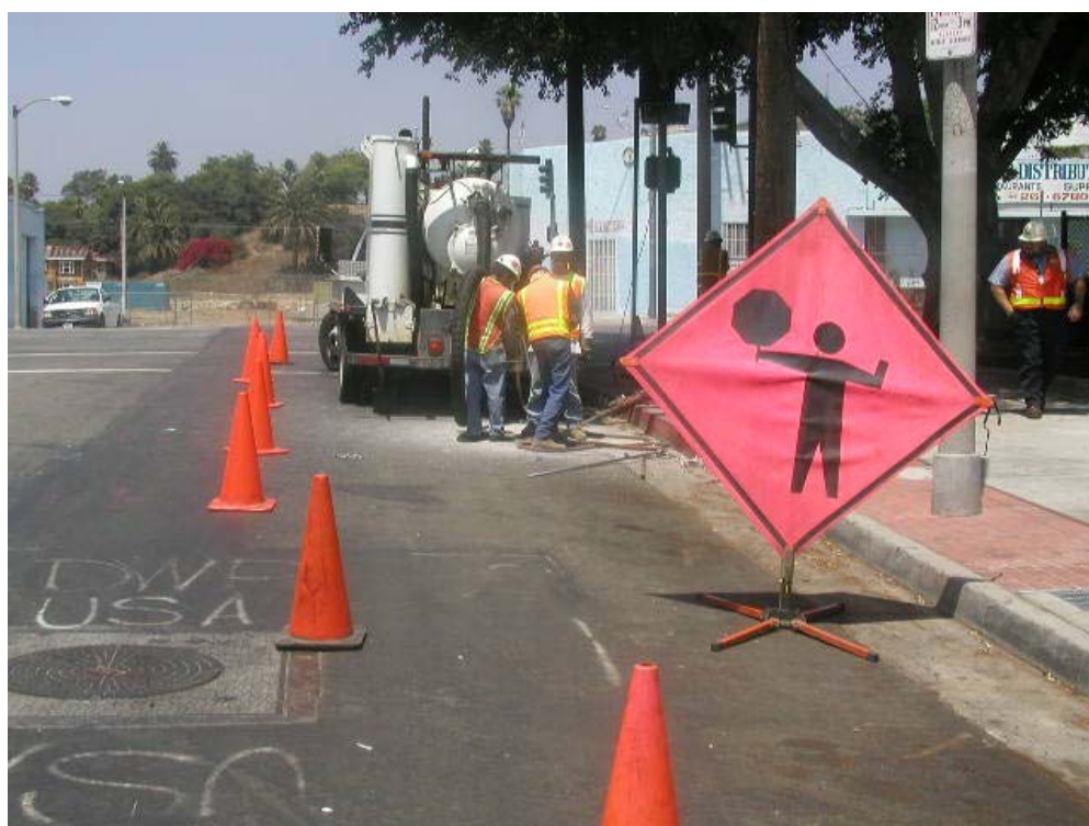
Utility potholing at 1 st Street and Gless Street.
