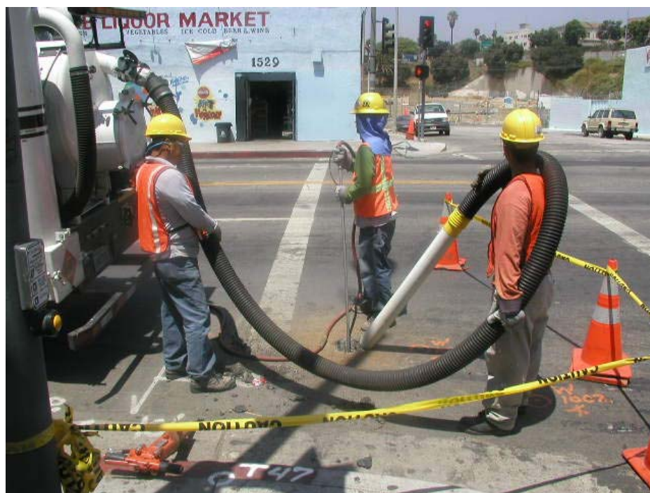
Utility potholing at 1 st Street and Gless Street.
