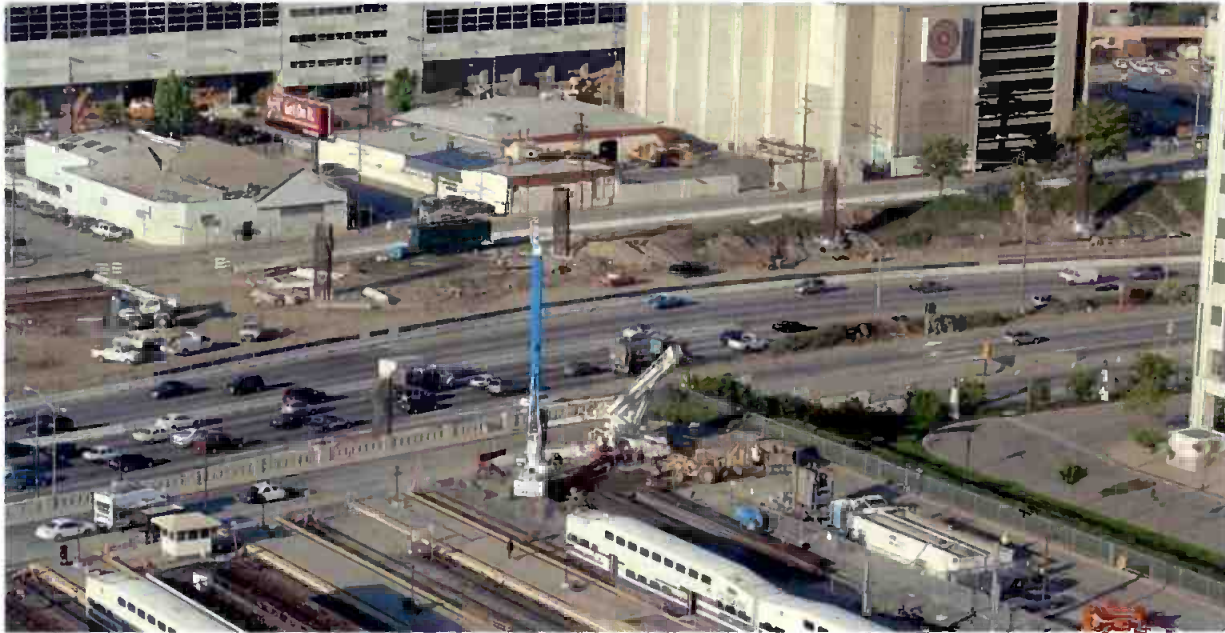
Column rebar cages for the 101 Freeway Overcrossing.
