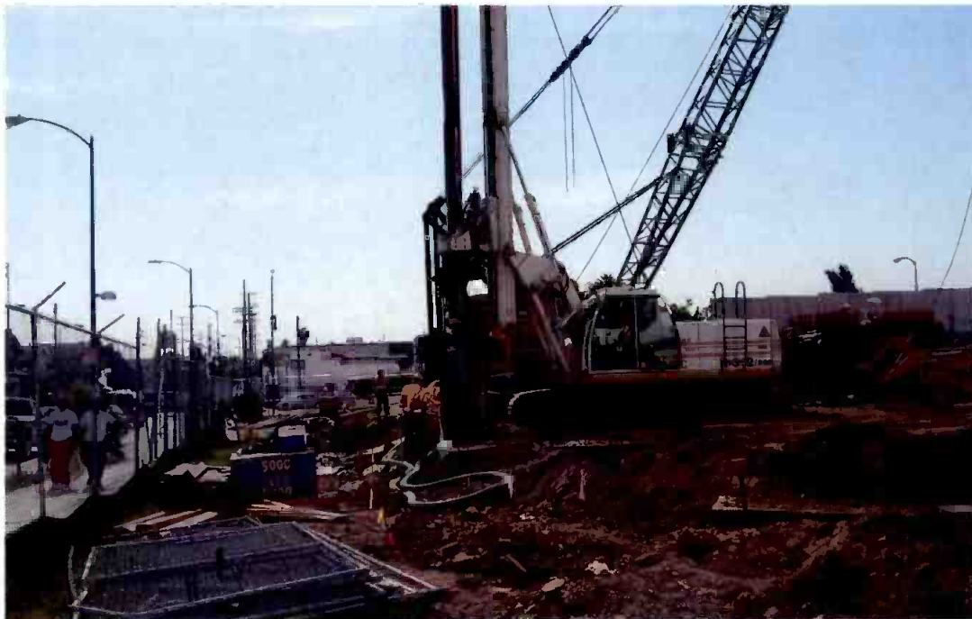
Soldier pile installation at Soto Station.
