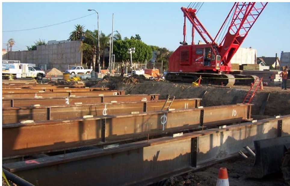
Street deck beams at Soto Station.
