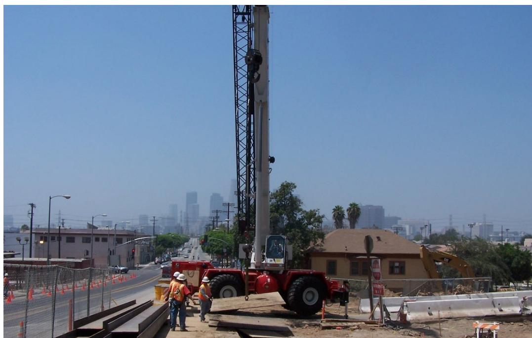
West Portal soldier pile installation.
