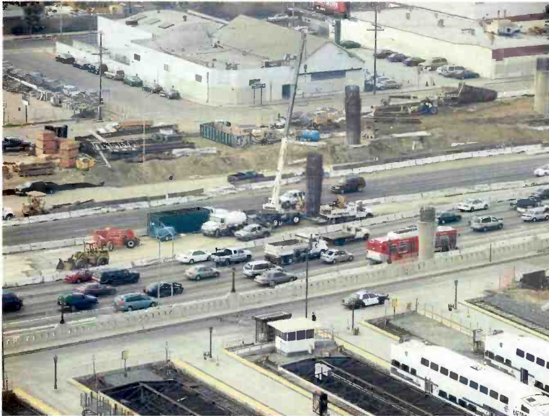
Placement of columns for the 101 Freeway Bridge Overcrossing.
