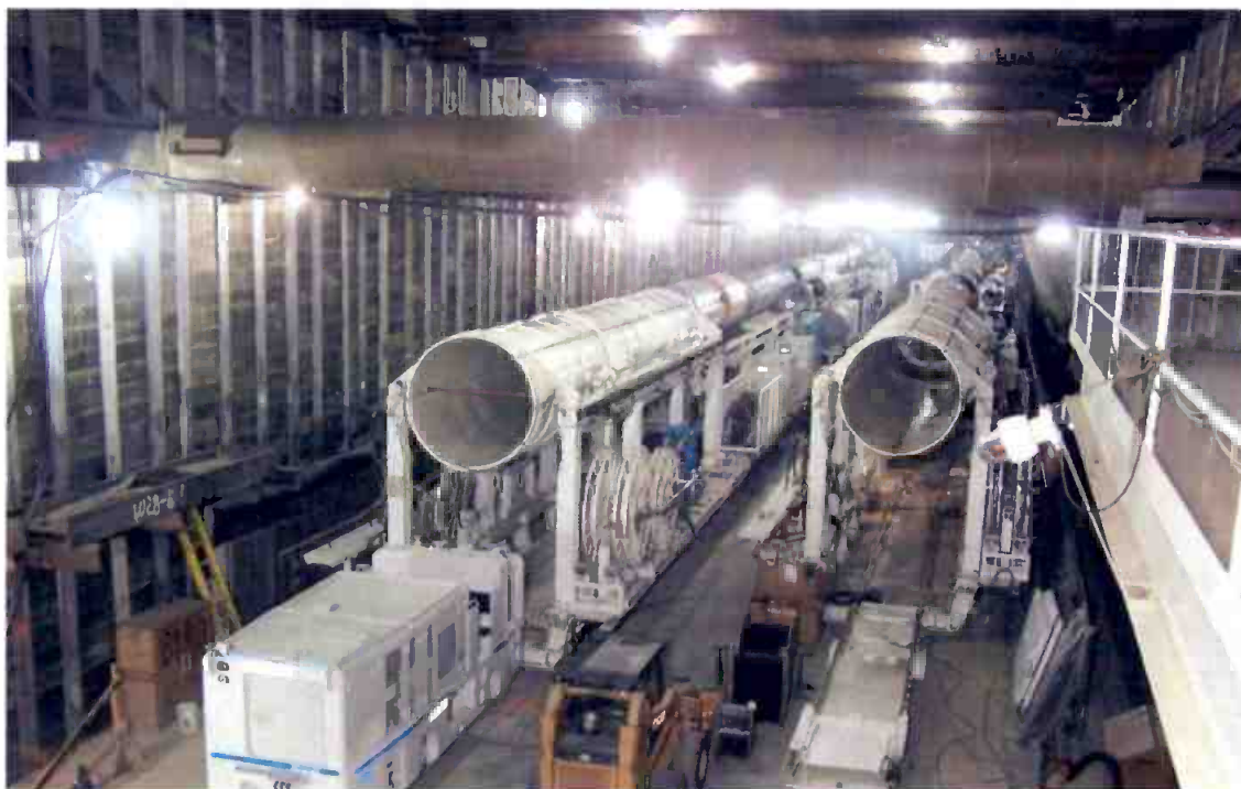
Tunnel Boring Machine assembly.
