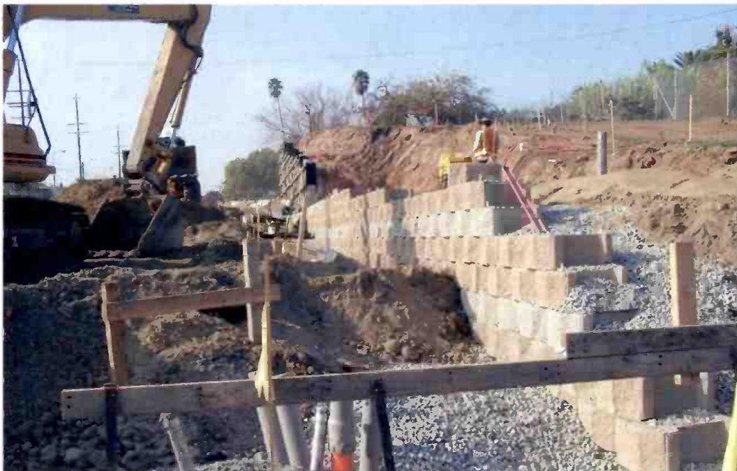
East Portal LA County Crematorium retaining wall.
