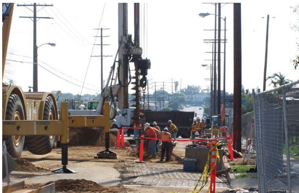
Soldier pile installation at the East Portal.
