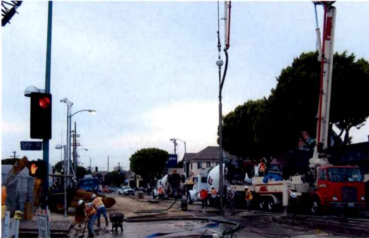
Soldier pile installation at Soto Station.
