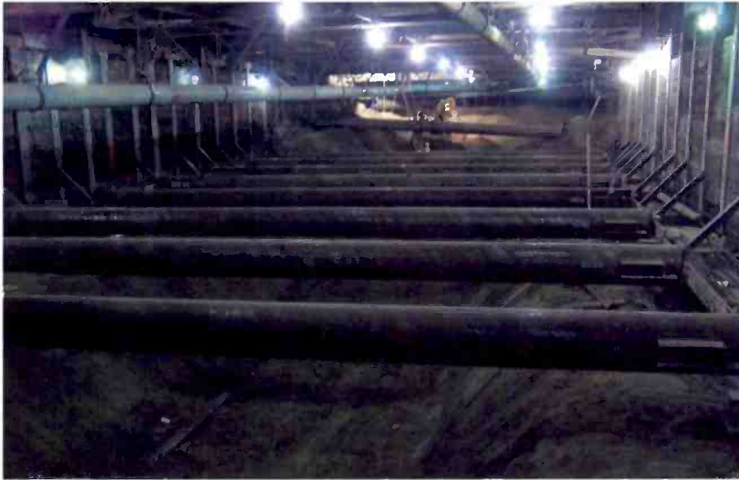
Struts in place and support of utilities at the Boyle Heights/Mariachi Plaza Station.
