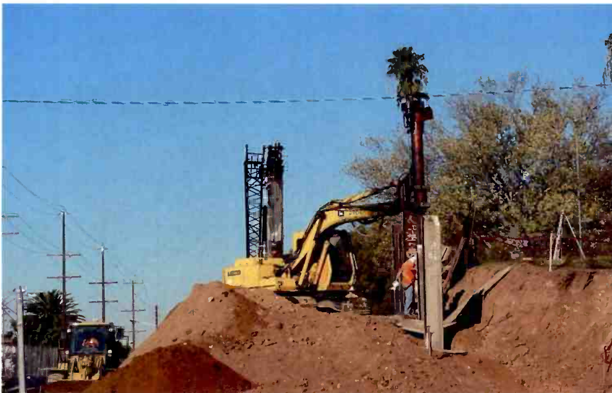
Pile Installation for the New Crematorium Retaining Wall at the East Portal.
