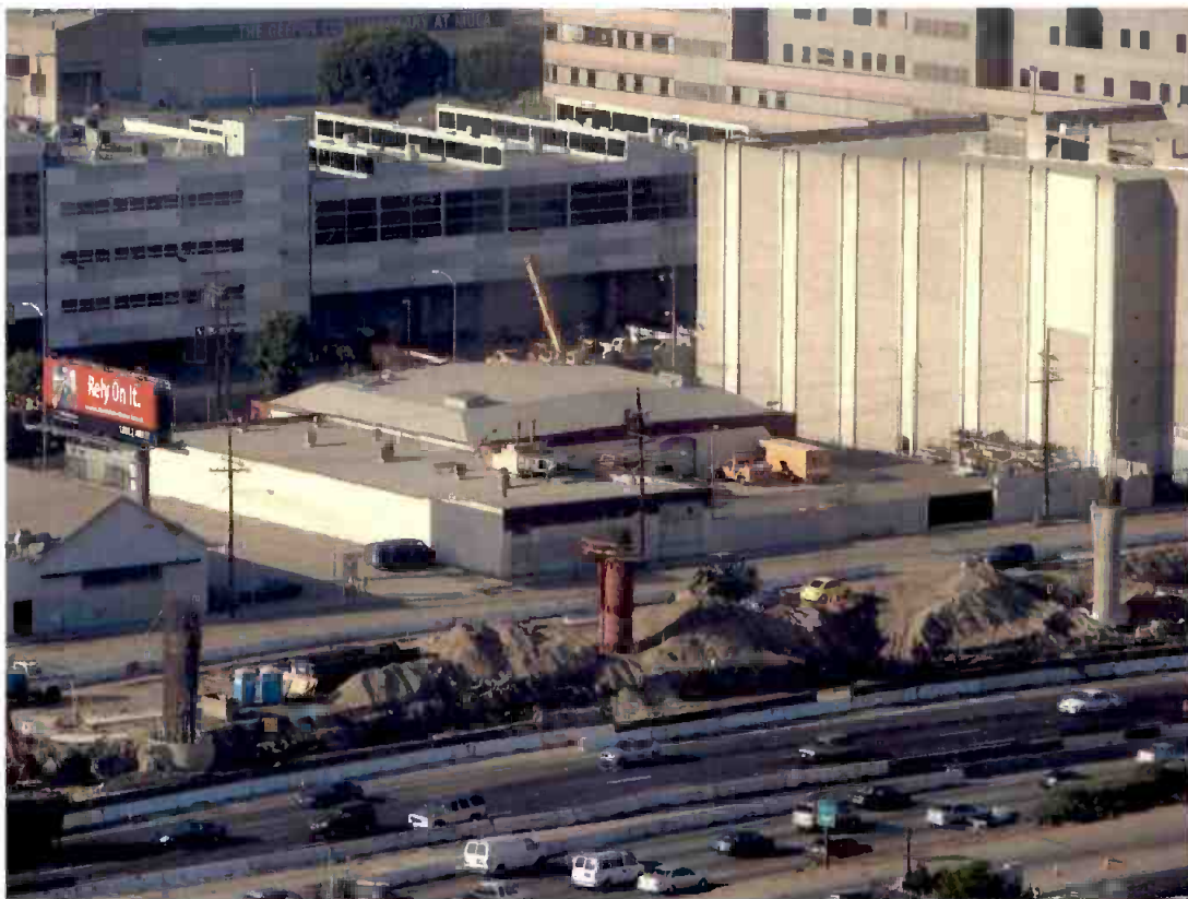
Columns for the 101 Freeway Bridge Overcrossing.
