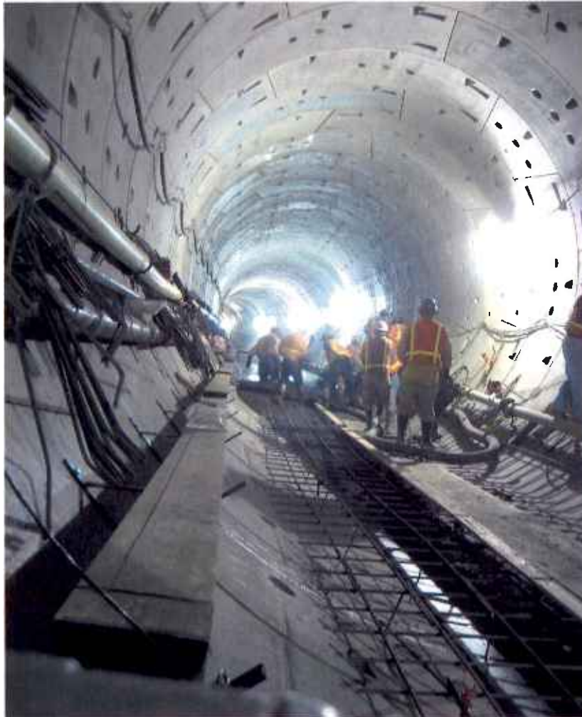
Concrete placement of the invert slab within the eastbound tunnel.
