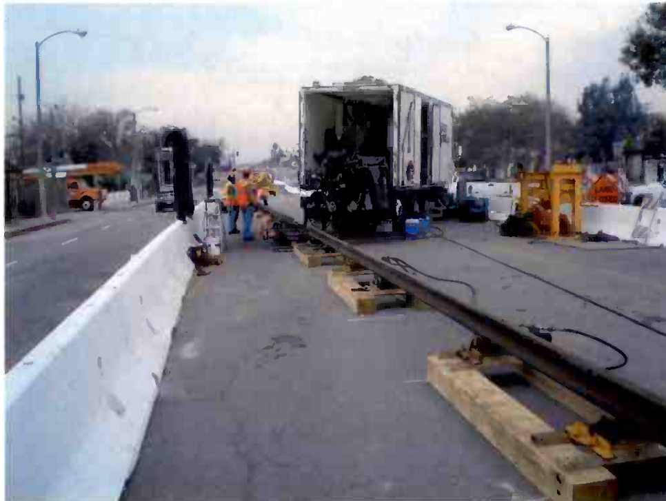
Set up of the rail welding facility on 3 rd Street.
