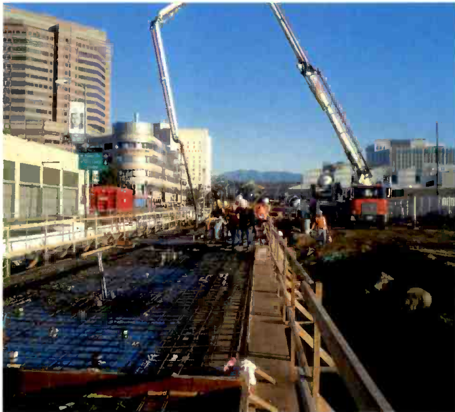
Concrete placement of the Little Tokyo/Arts District Station platform.
