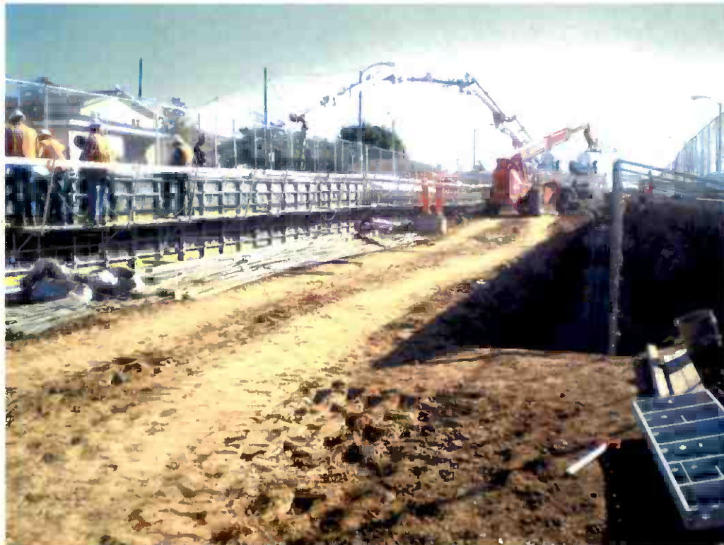
Construction of the retaining walls for the U-Channel on 3 rd Street.
