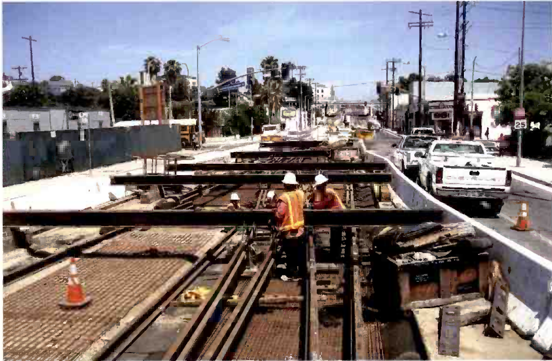
Construction of Segment 2B track crossover.
