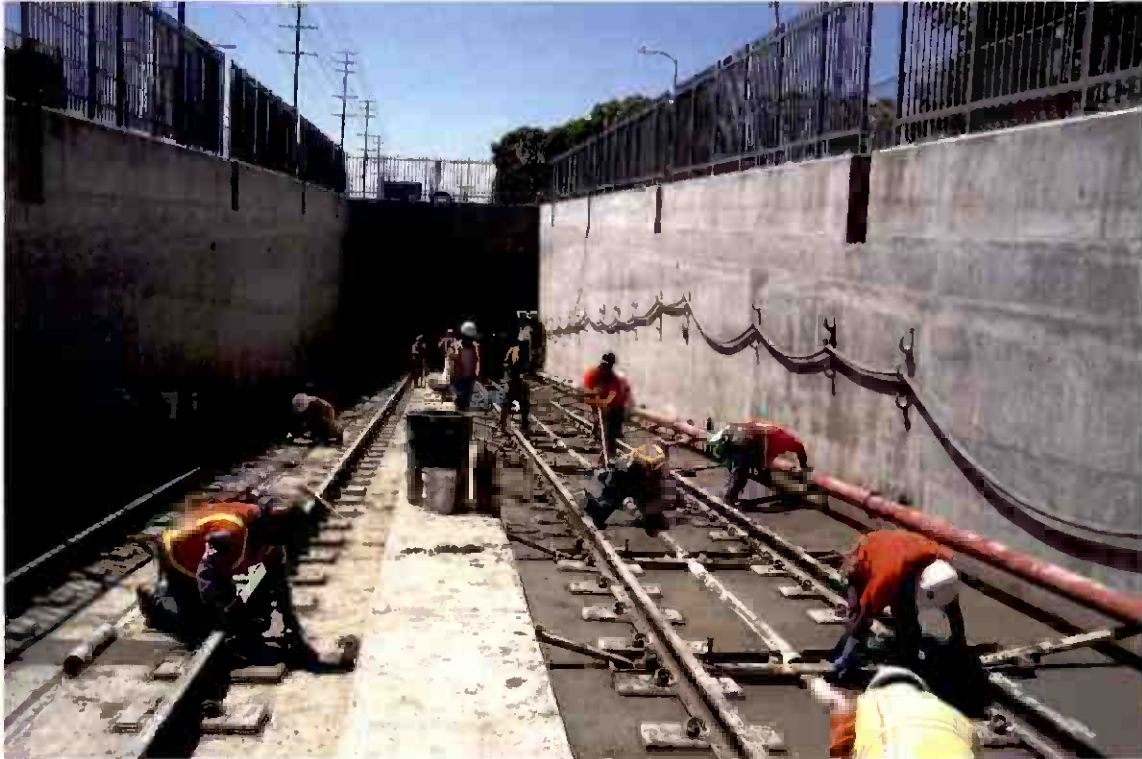
Concrete placement for the WB track at the East Portal.
