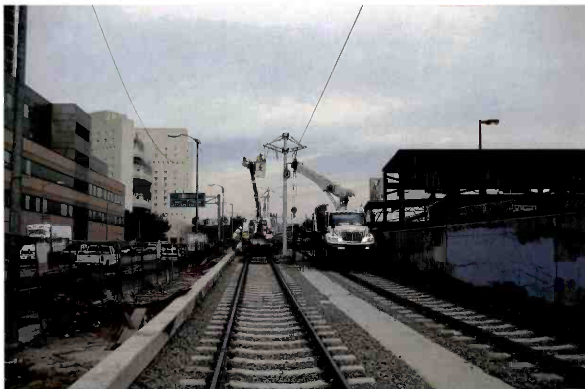
Installation of OCS messenger wire in the guideway along Alameda Street.
