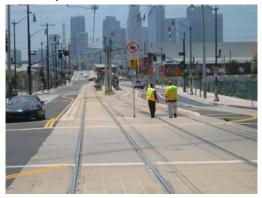
vehicle traffic and to define the dynamic envelope of the train. The latter is particularly important for those segments where trains mix with vehicular traffic, such as in roadway intersections. Typical means to delineate the trainway are by striping, curbs (including mountable curbs), raised buttons or other tactile treatment. Along 1<sup>st</sup> Street and 3<sup>rd</sup> Street, the trainway is delineated by a 6-inch mountable curb, colored stamped concrete, and in some
