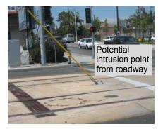
At several locations, catenary poles and catenary guy wires are located at the intrusion entry point of the trainway. The poles and guy wires need to be protected from errant vehicles. An option is to protect the poles and guys with bollards striped with retro-reflective tape. See Figure 3.
