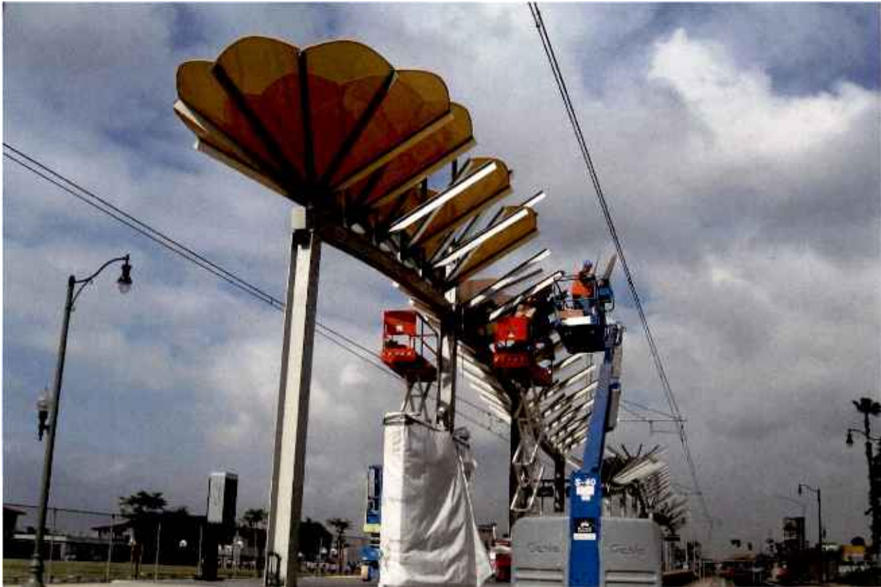
Installation of Lexan panels in the canopy at the East LA Civic Center Station.
