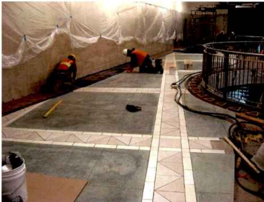
Placement of mezzanine floor tiles at the Boyle Heights/Mariachi Plaza Station.
