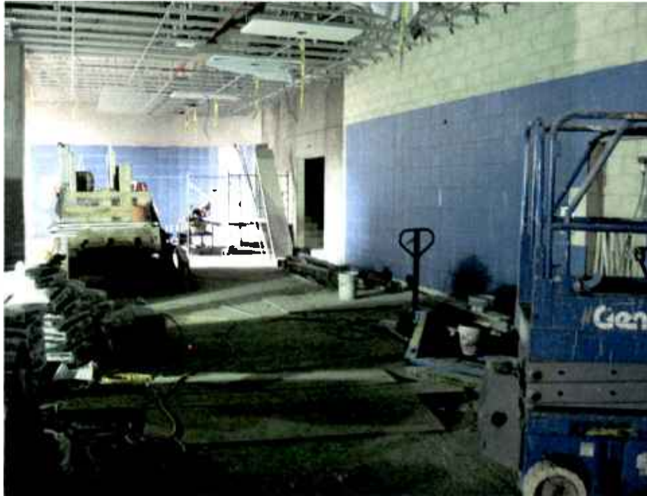
Installation of Soto Station entrance wall tiles.
