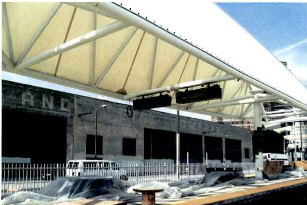
Installation of variable message signs and public address speakers within the Little Tokyo/Arts District Station canopy.
