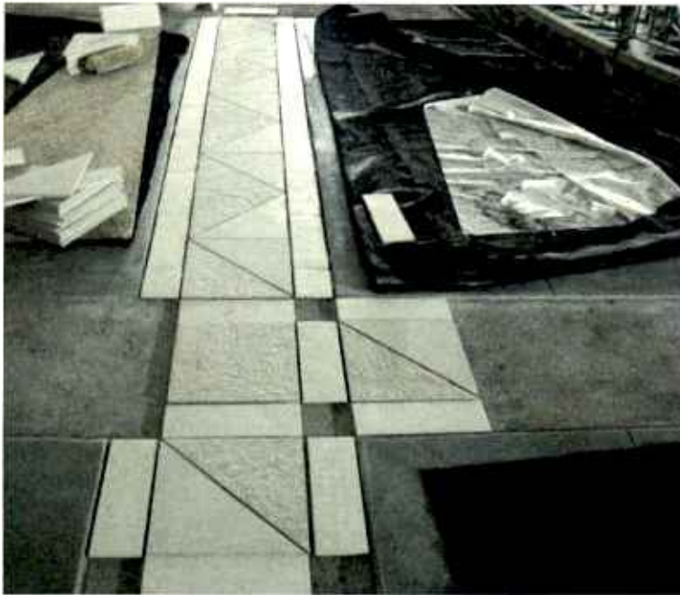
Placement of mezzanine floor tiles at the Boyle Heights/Mariachi Plaza Station.
