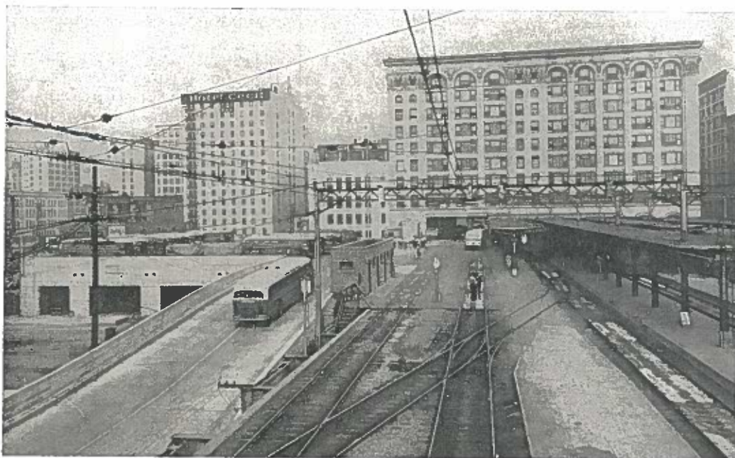
ELEVATED RAIL AND MOTOR BUS TERMINAL CONSTRUCTED IN CENTRAL LOS ANGELES
