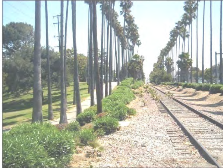
Harbor Subdivision looking east, adjacent to Edward Vincent Jr. Park and Florence Avenue.
