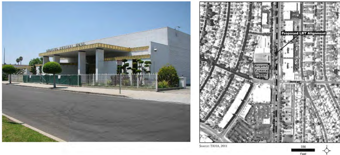
Figure 4-49. Angelus Funeral Home – 3886 Crenshaw Boulevard
