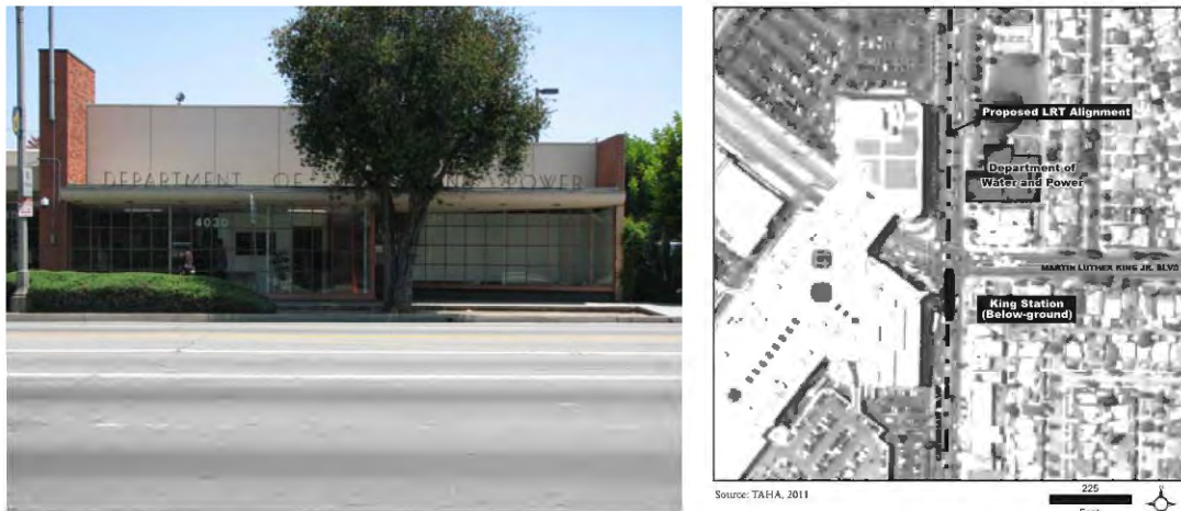
Figure 4-48. Department of Water and Power – 4030 Crenshaw Boulevard
