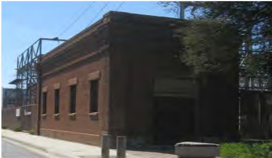
Figure 4-52. Edison Substation – Florence and Fir Avenues
