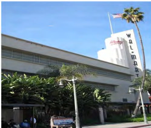
The distinct architecture of the Wal-Mart (former Broadway Department Store) building located in the Baldwin Hills-Crenshaw Plaza at Martin Luther King Jr. Boulevard. (C3)
