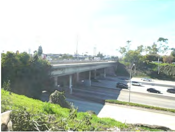
Florence Avenue bridge over I-405 looking northeast.
