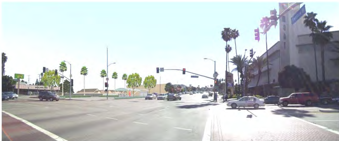
Crenshaw/King Station southeast portal, looking south on Crenshaw Boulevard at Martin Luther King Jr. Blvd. would result in the removal of commercial buildings but would not adversely affect the visual character of the area.
