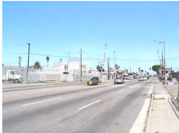
South of the Harbor Subdivision looking north on Crenshaw Blvd (alignment also below grade).
