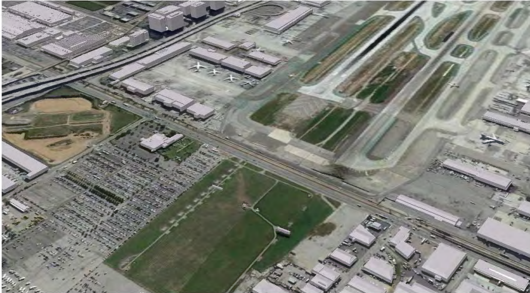
Existing view of Aviation Boulevard in front of the LAX south runways.
