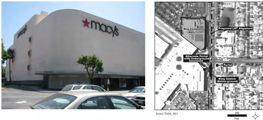
Figure 4-47. May Company Department Store (now Macy's) – 4005 Crenshaw Boulevard
