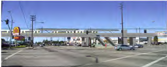
Aerial structure across Manchester Avenue.
