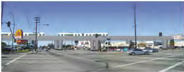
Aerial structure across Manchester Avenue.
