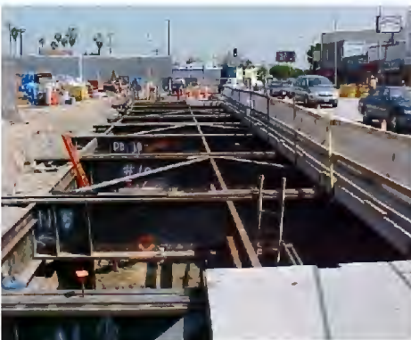
Cut and Cover Construction Goldline Eastside Extension
