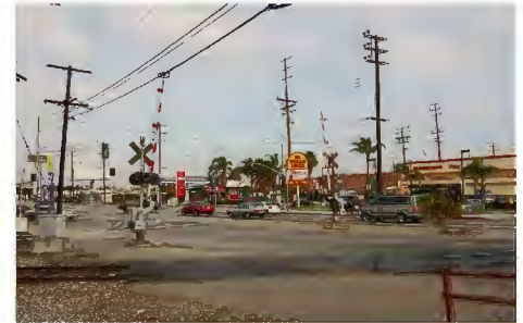
Grade Crossing at Manchester.
